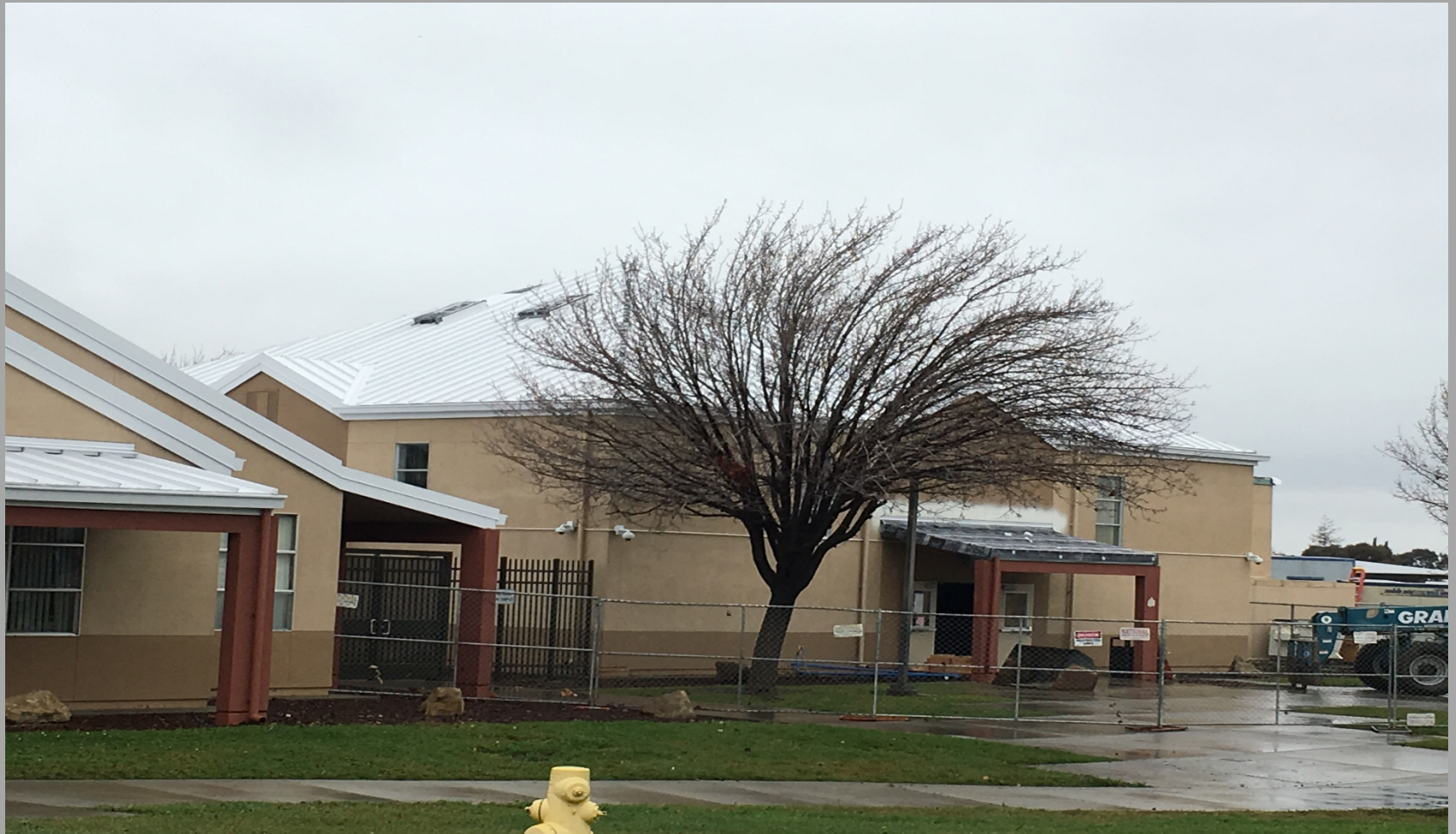
View of Roofing Replacement Work @ Building E - Looking Northeast
