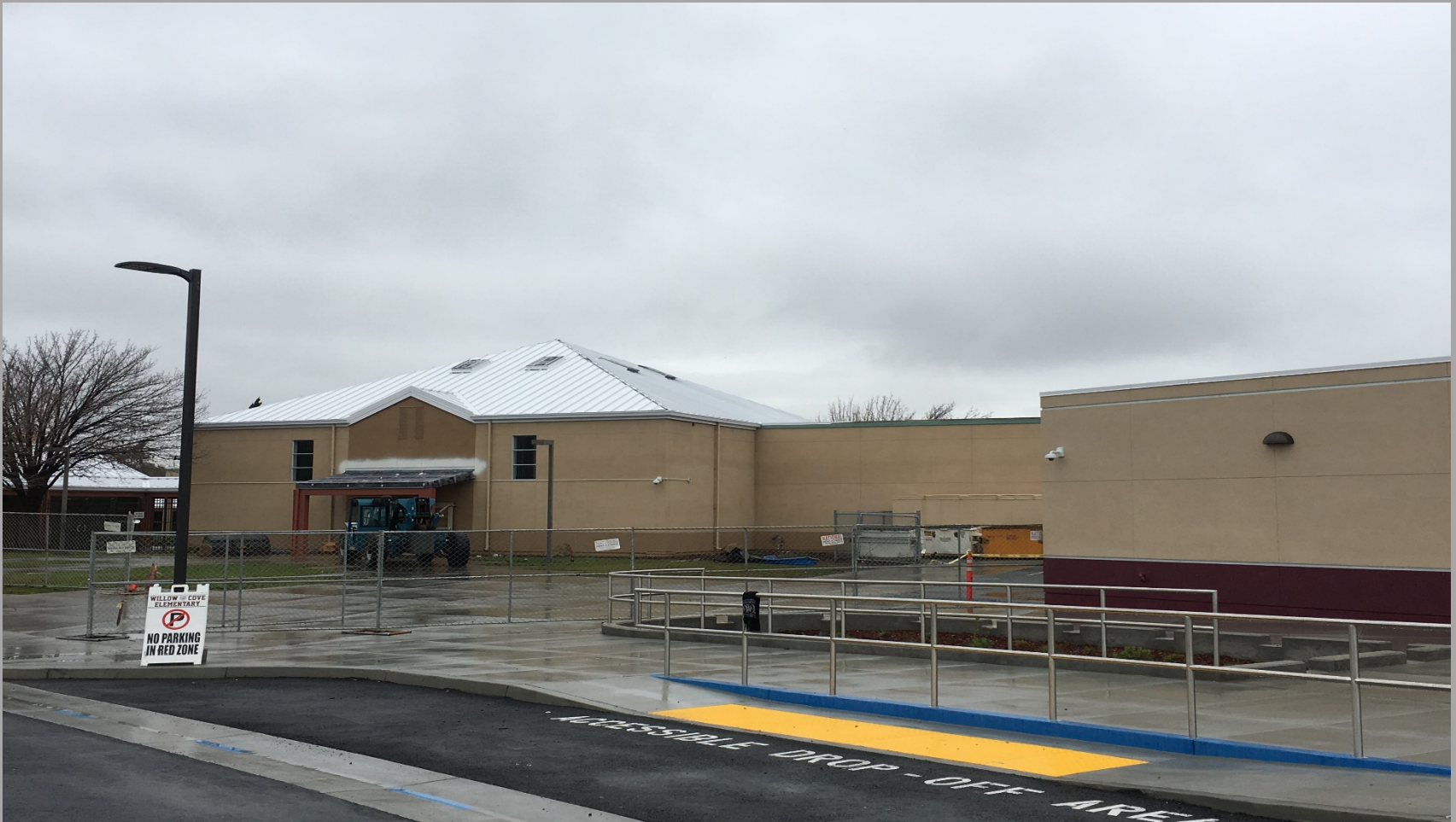
View of Roofing Replacement Work @ Building E - Looking Northwest
