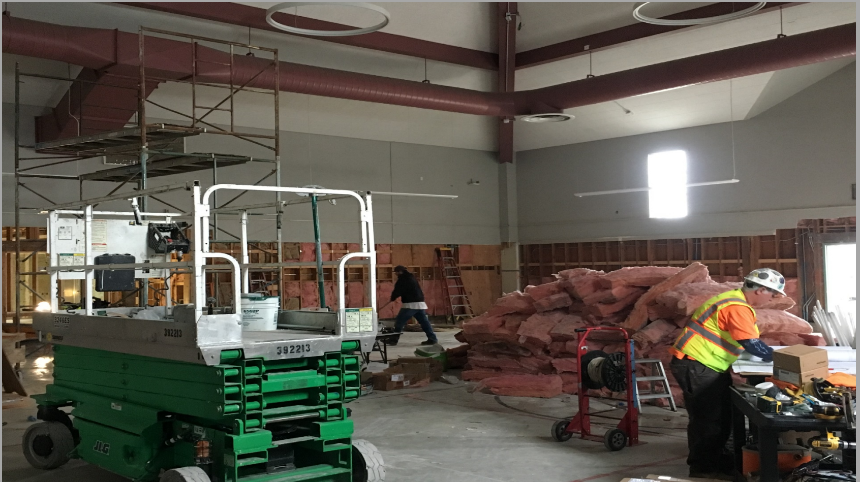
View of Demolition Completion Inside of Building E - Looking Southwest
