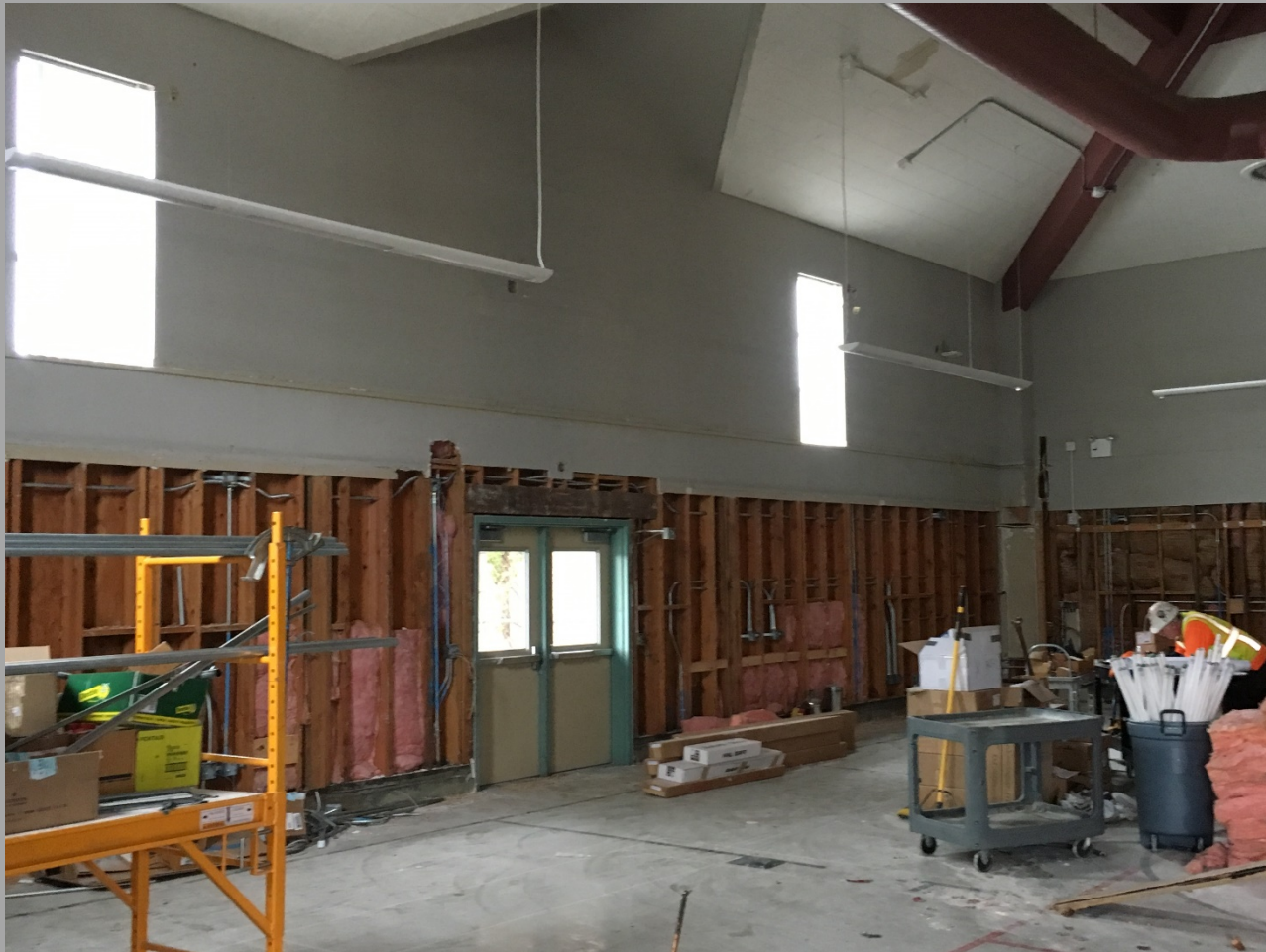
View of Demolition Completion Inside of Building E - Looking Northwest
