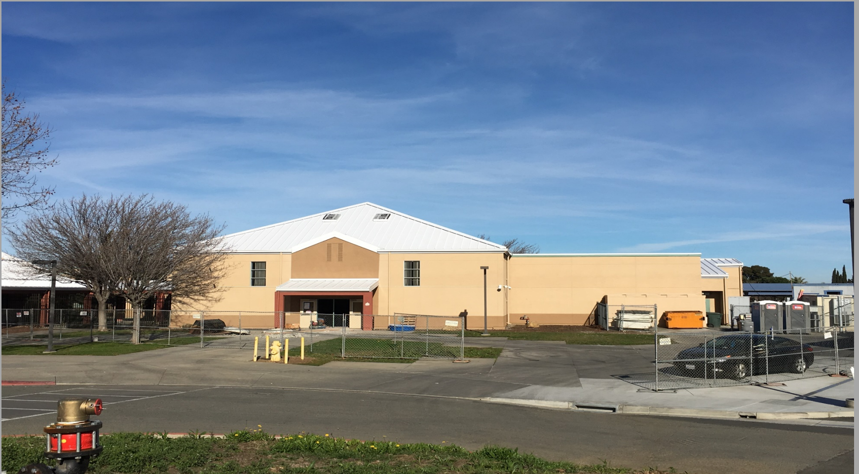
View of Nearly Complete Roofing Replacement Work @ Building E - Looking Northwest
