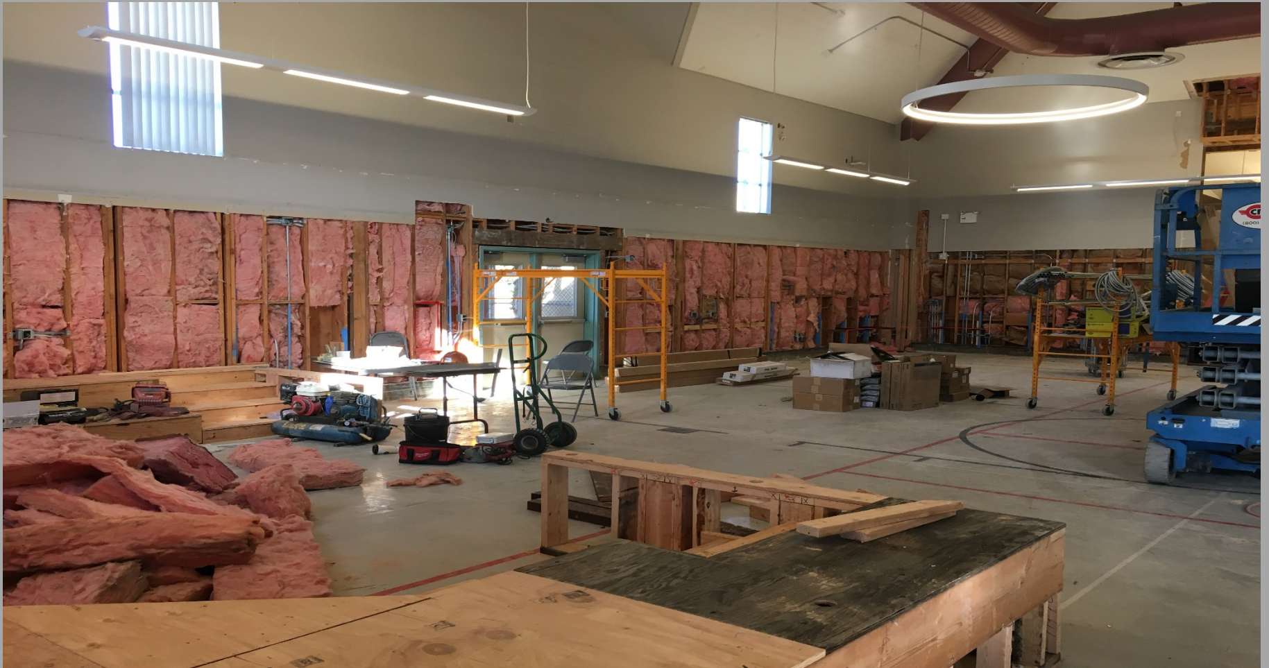
View of Modernization Work @ Building E - Looking Northwest
