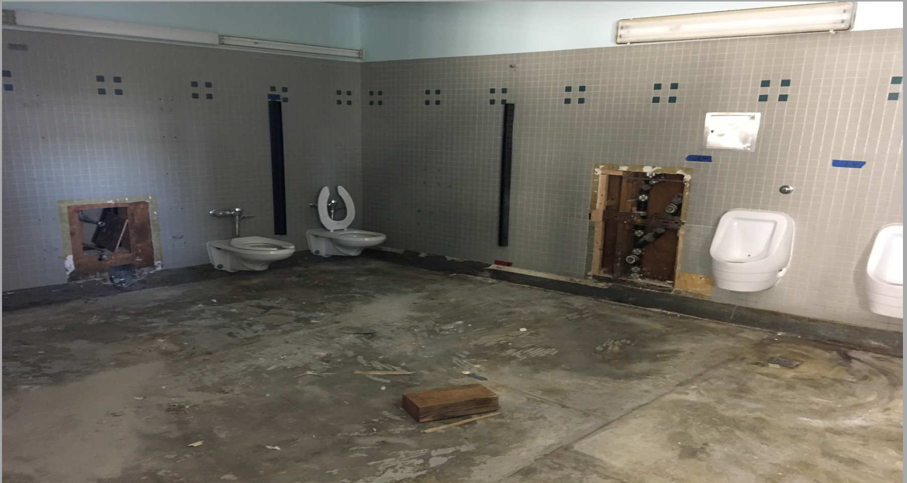
View of Boys Restroom Demolition Work @ Building E - Looking Southeast
