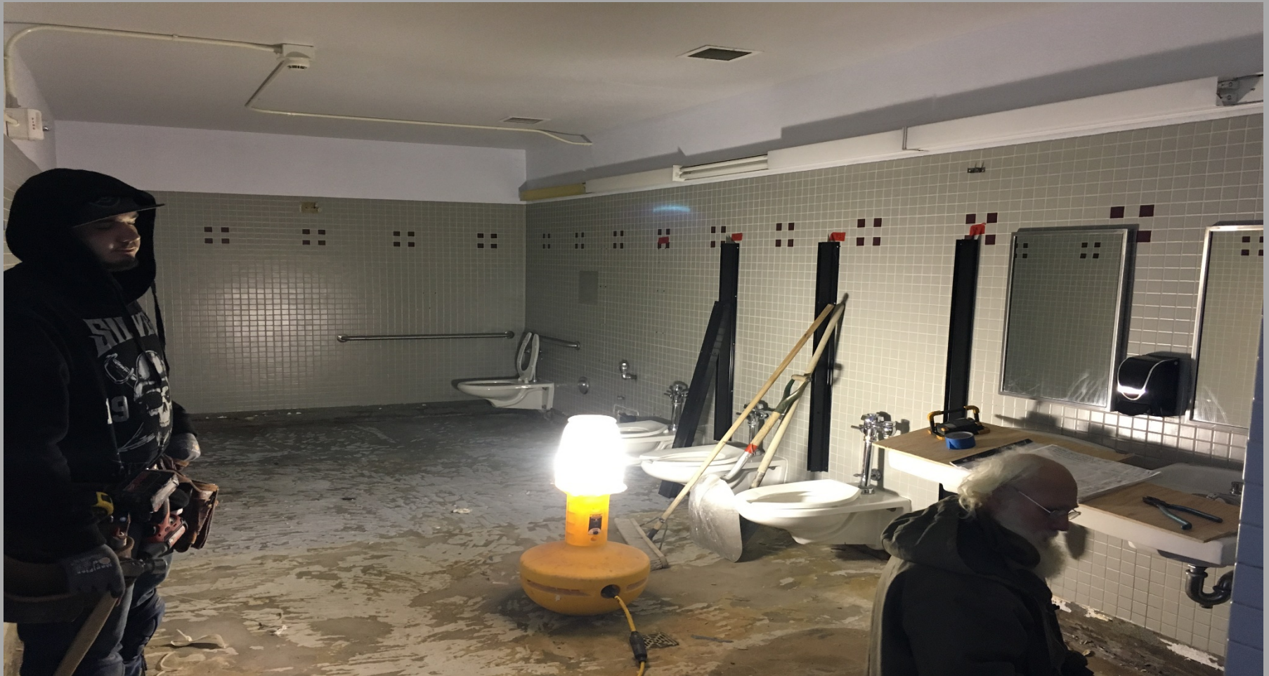
View of Girls Restroom Demolition Work @ Building E - Looking Southwest
