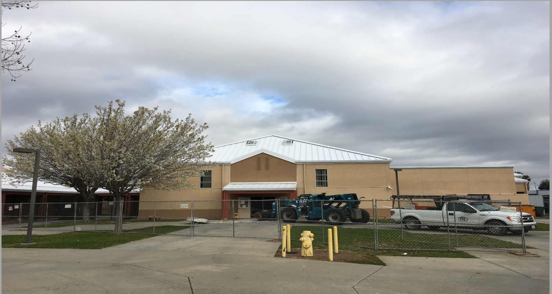
View of New Roofing on Building E - Looking North
