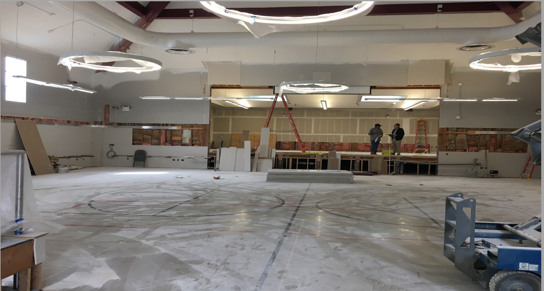
View of Modernization Work @ Building E - Looking North toward Computer Lab.
