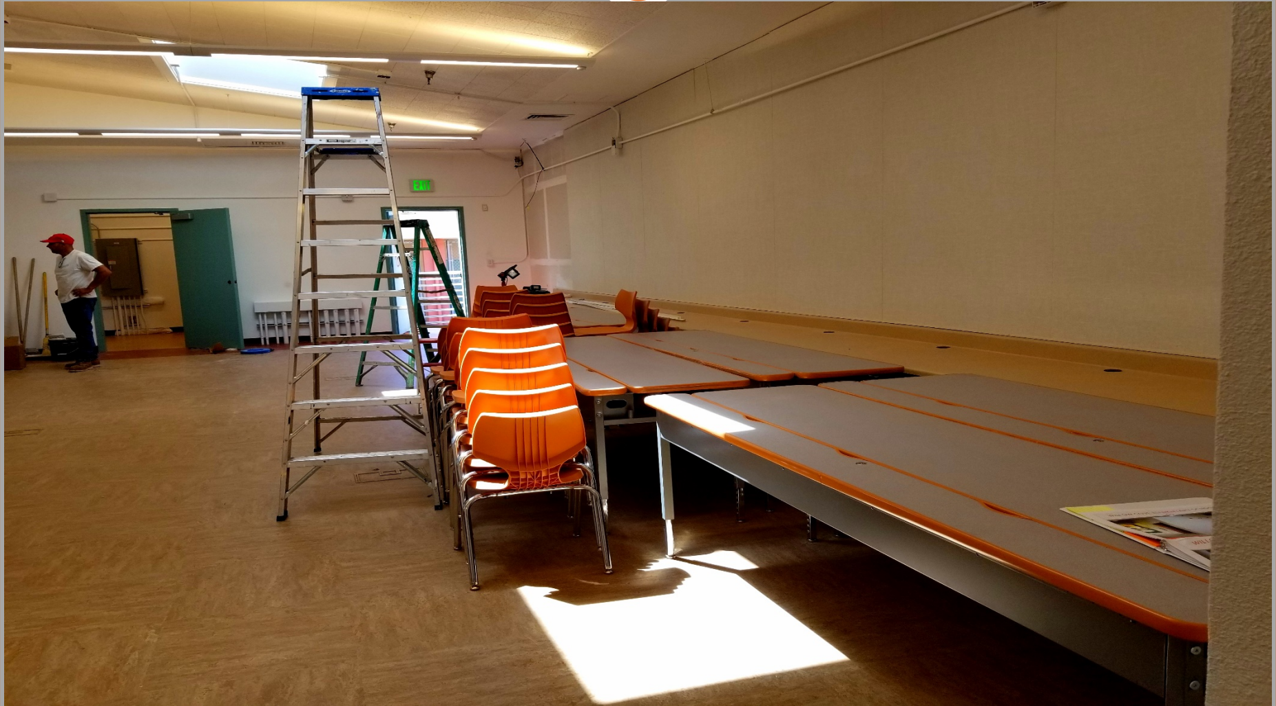
Building E - Computer room furniture tackable wall board installation nearly completed.
