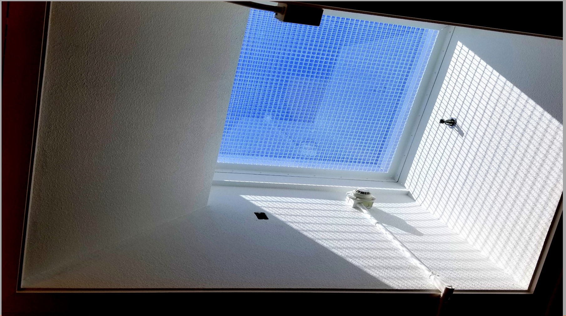
Building E - Security screen has been installed.
