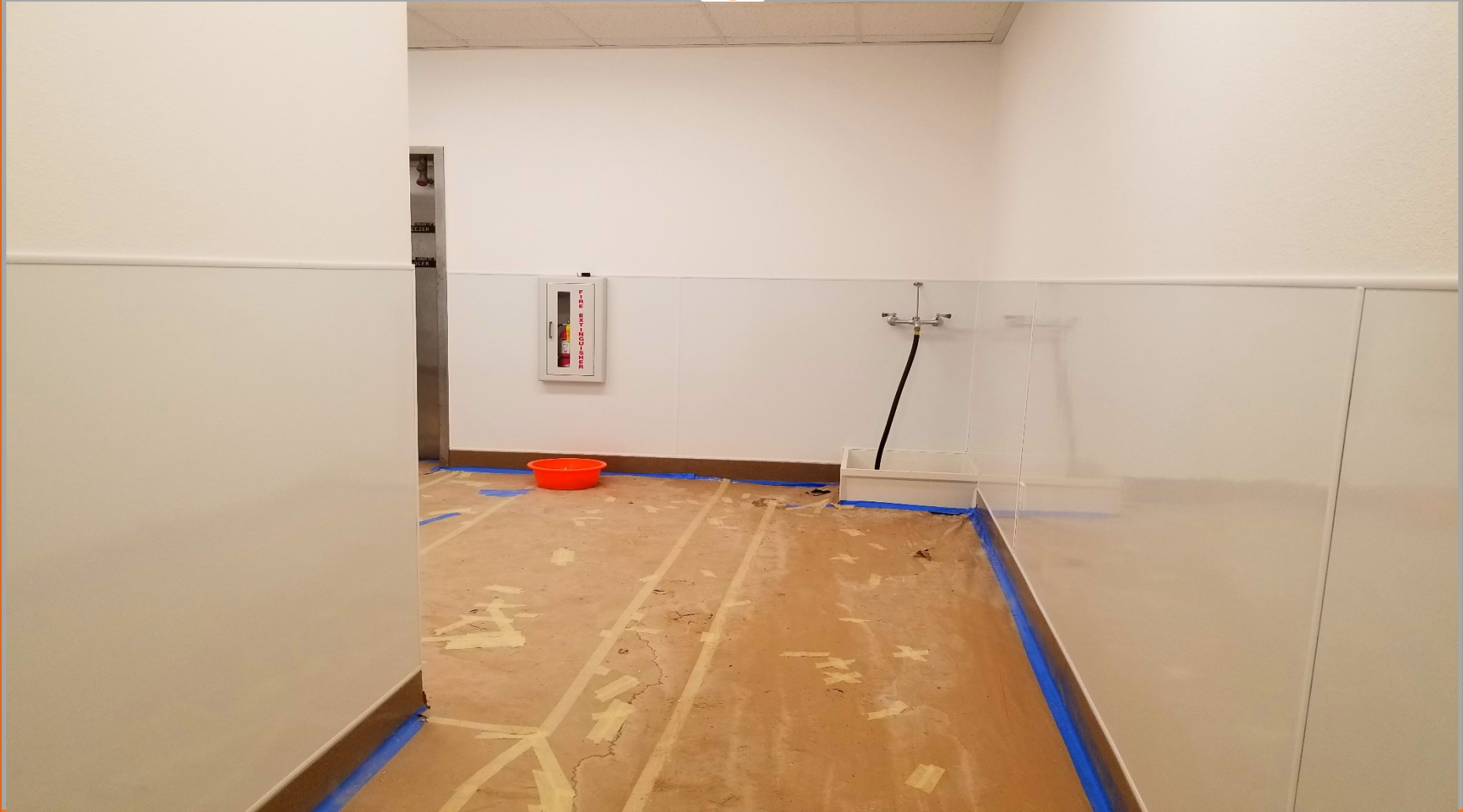
Building E – View of the Custodial Room with paper-protecting epoxy floor.
