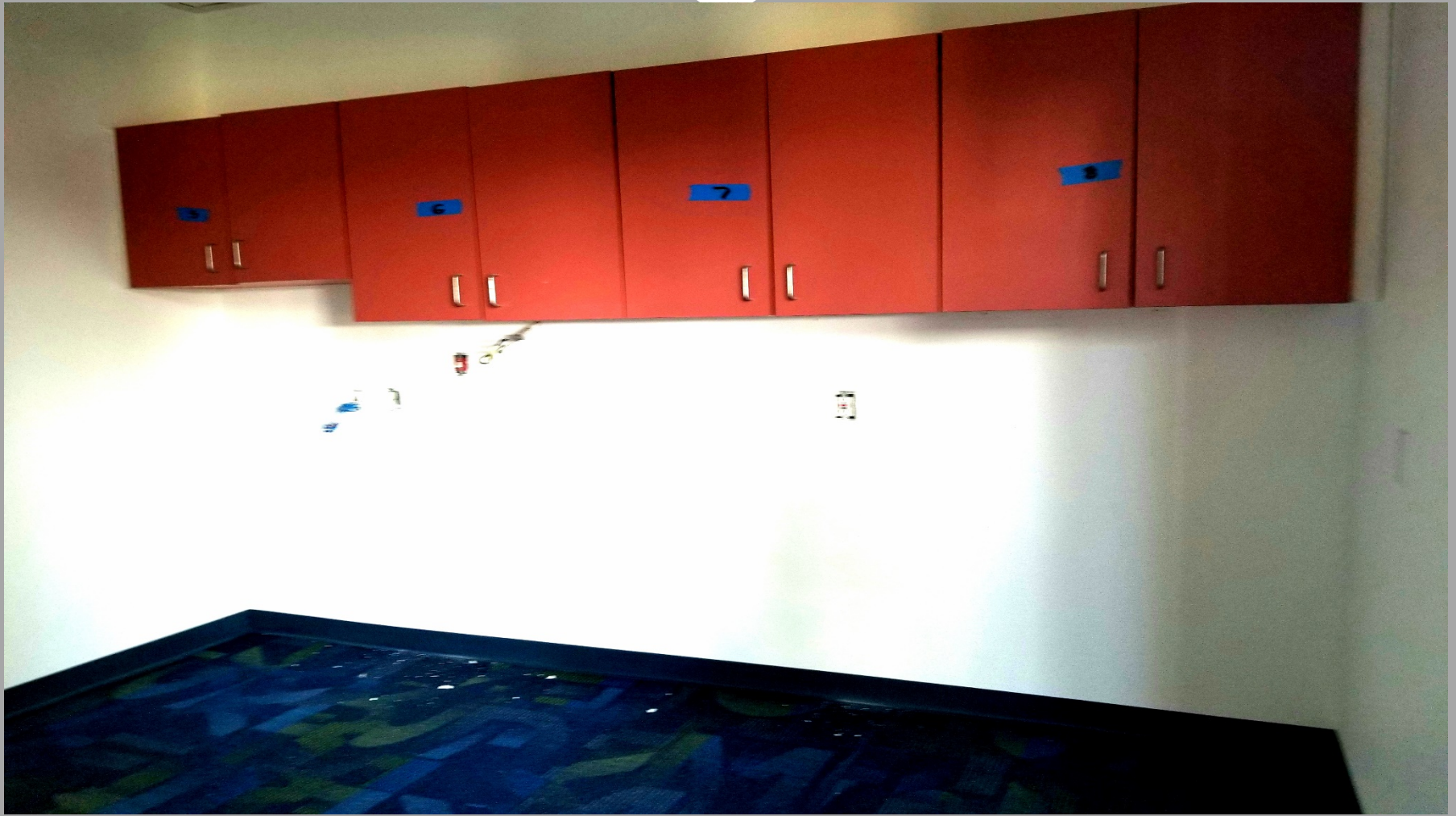
Office in Building D - nearing completion.
