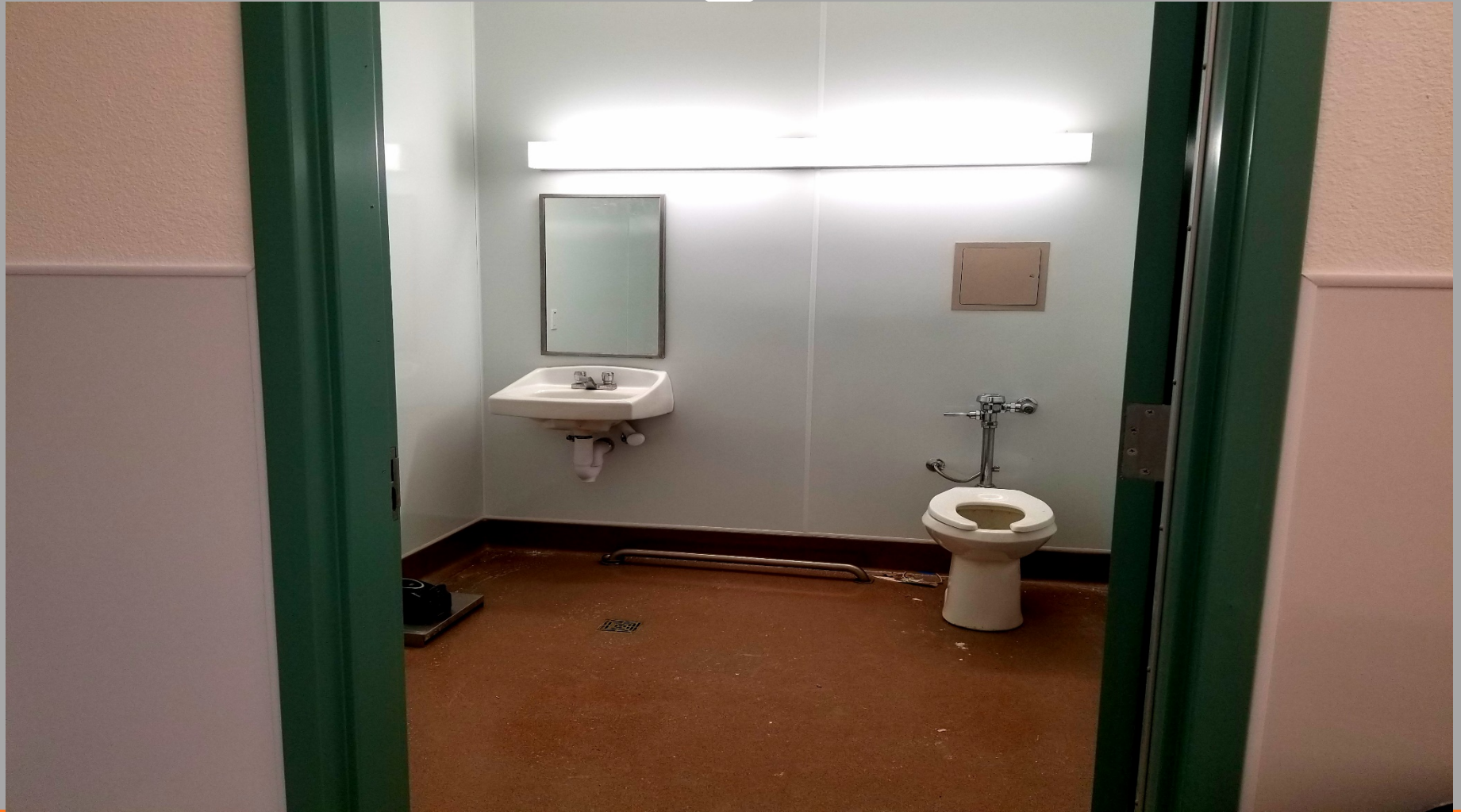
Building E - Bathroom fixtures has been set.
