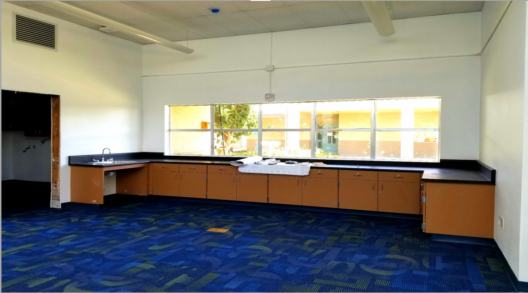
Building D – Carpeting and cabinets have been installed.
