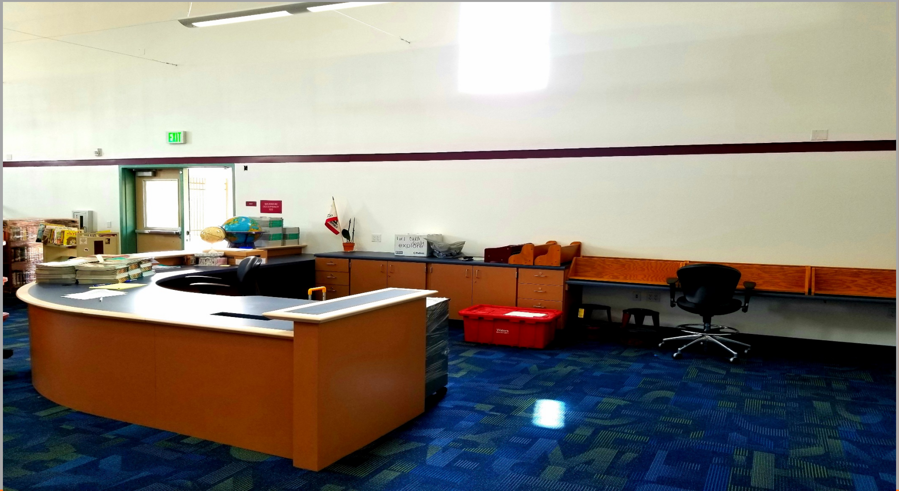
View of Modernization Work @ Building E - New Library is getting set up at her desk.
