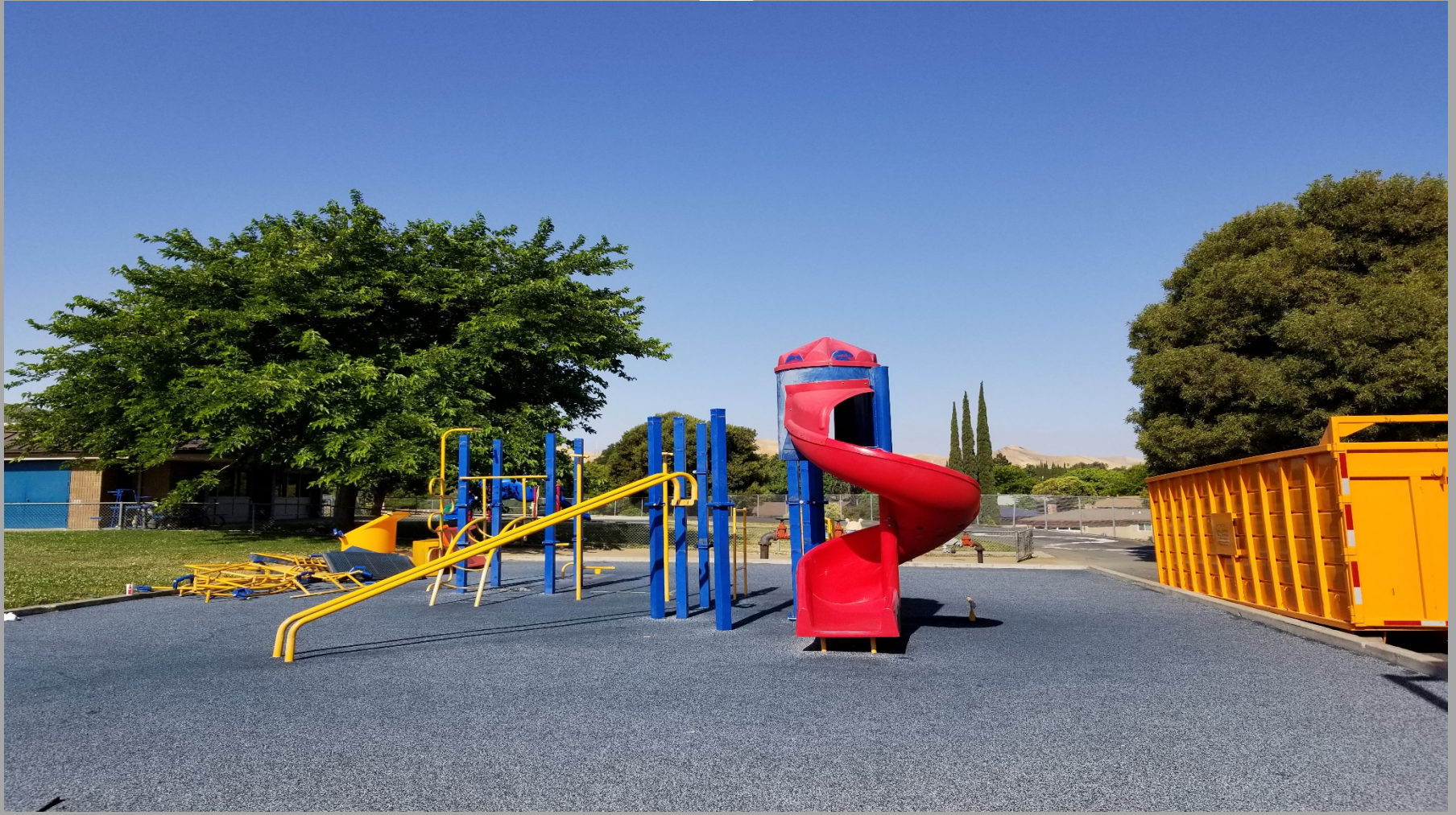
Foothill ES - Old Play Structure demolition in progress
