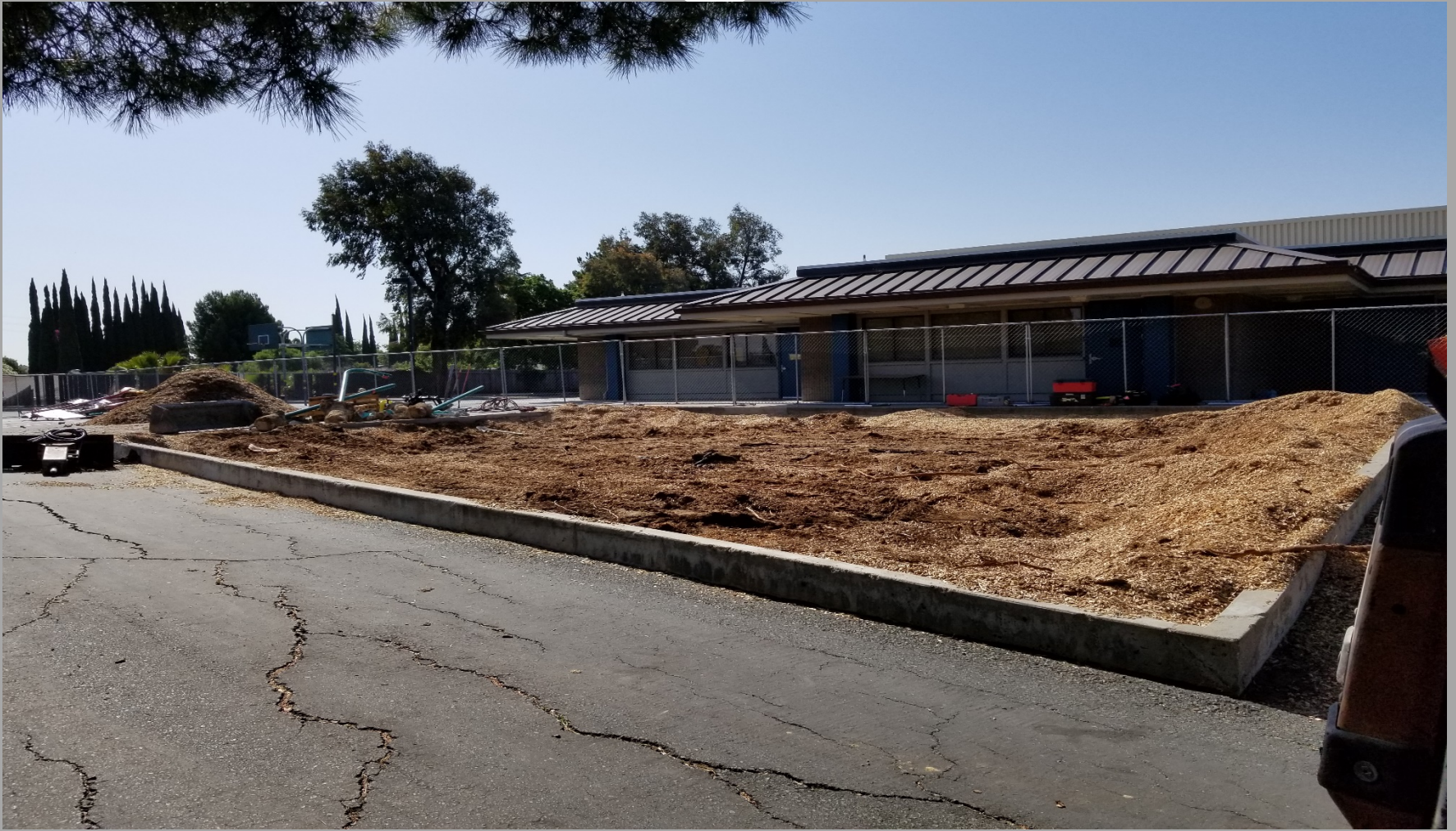
Foothill ES - Old Play Structure demolition in progress
