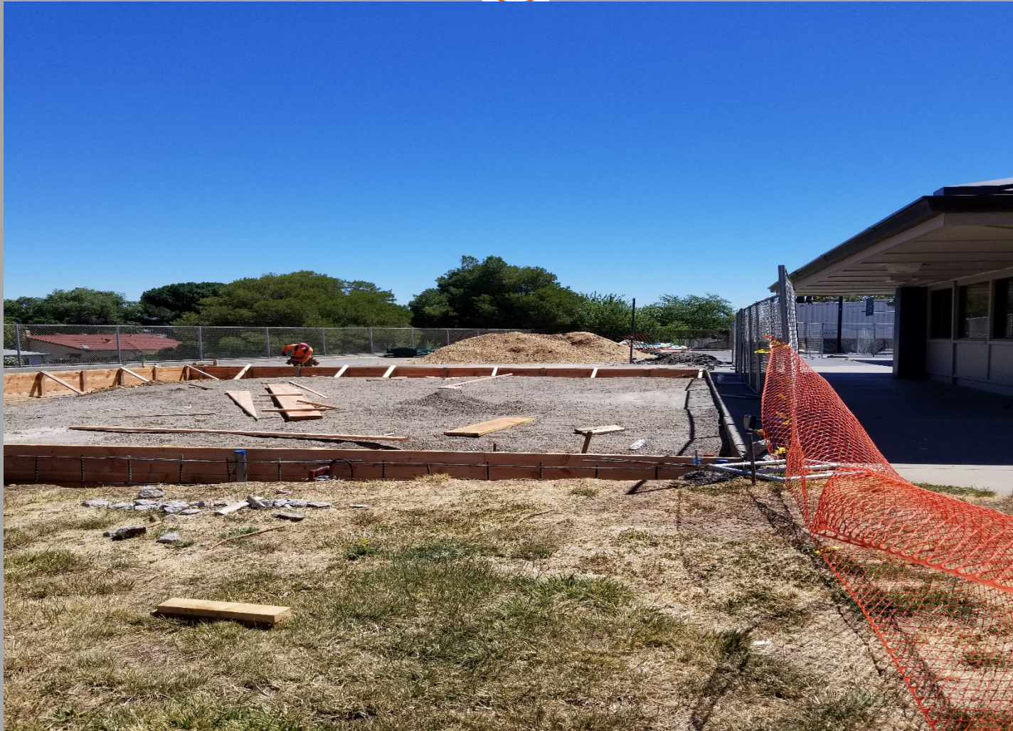
Foothill ES - Laying out foundation in progress.
