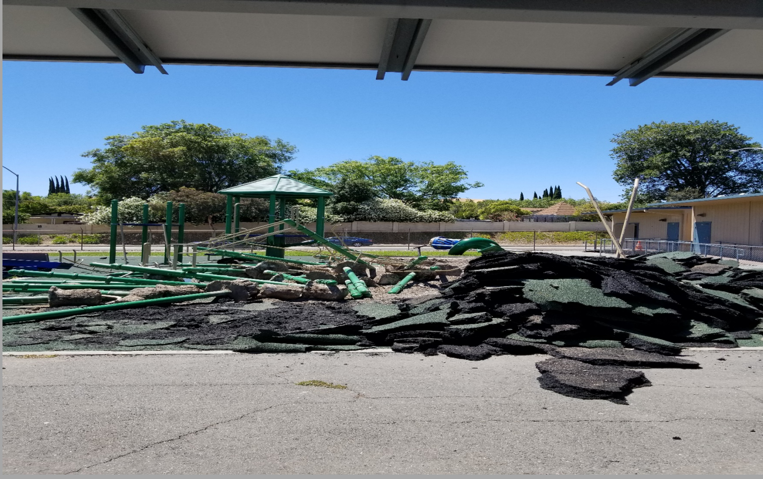
Highlands ES - Old Play Structure demolition in progress.
