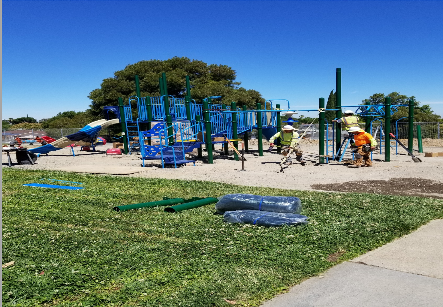
Foothill ES - Installation of New Play Structure is in progress.
