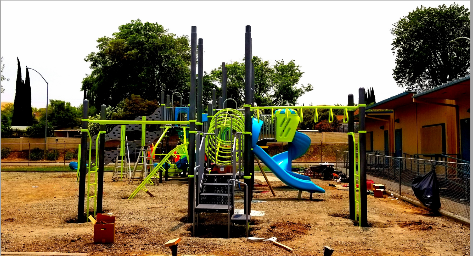
Highlands ES New Play Structure installation in progress.
