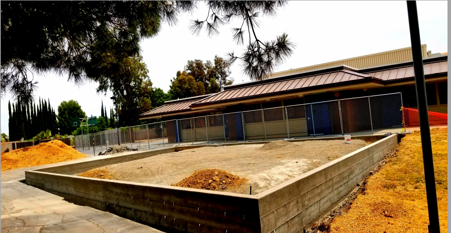
Foothill ES 2 nd Play Structure in progress.
