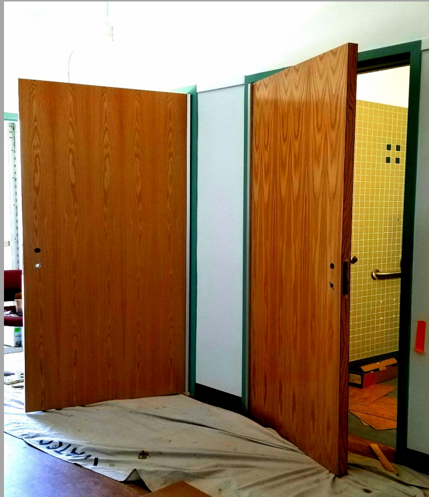
Willow Cove ES - Building E New Bathroom Doors Installation, in progress.
