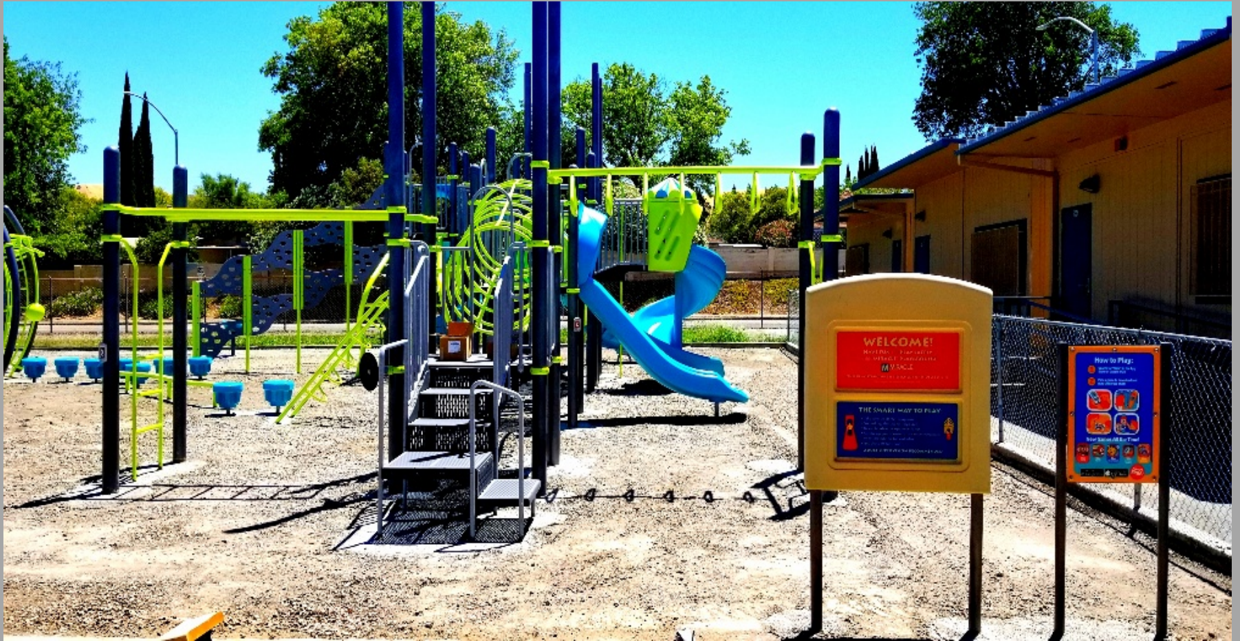
Highlands ES New Play Structure – Concrete Pour Done.
