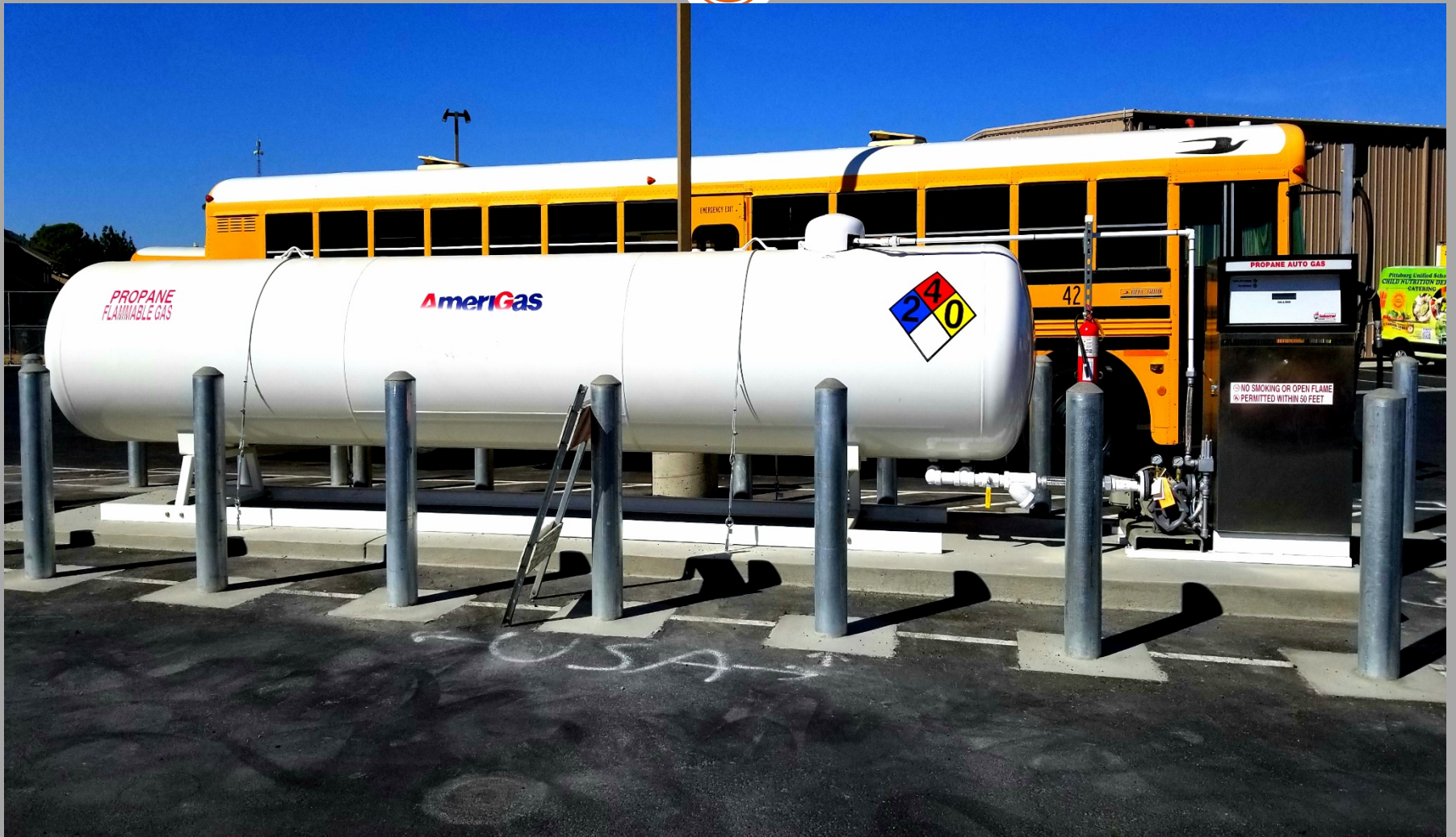
Propane Tank Pad and Bollards Project, installed.
