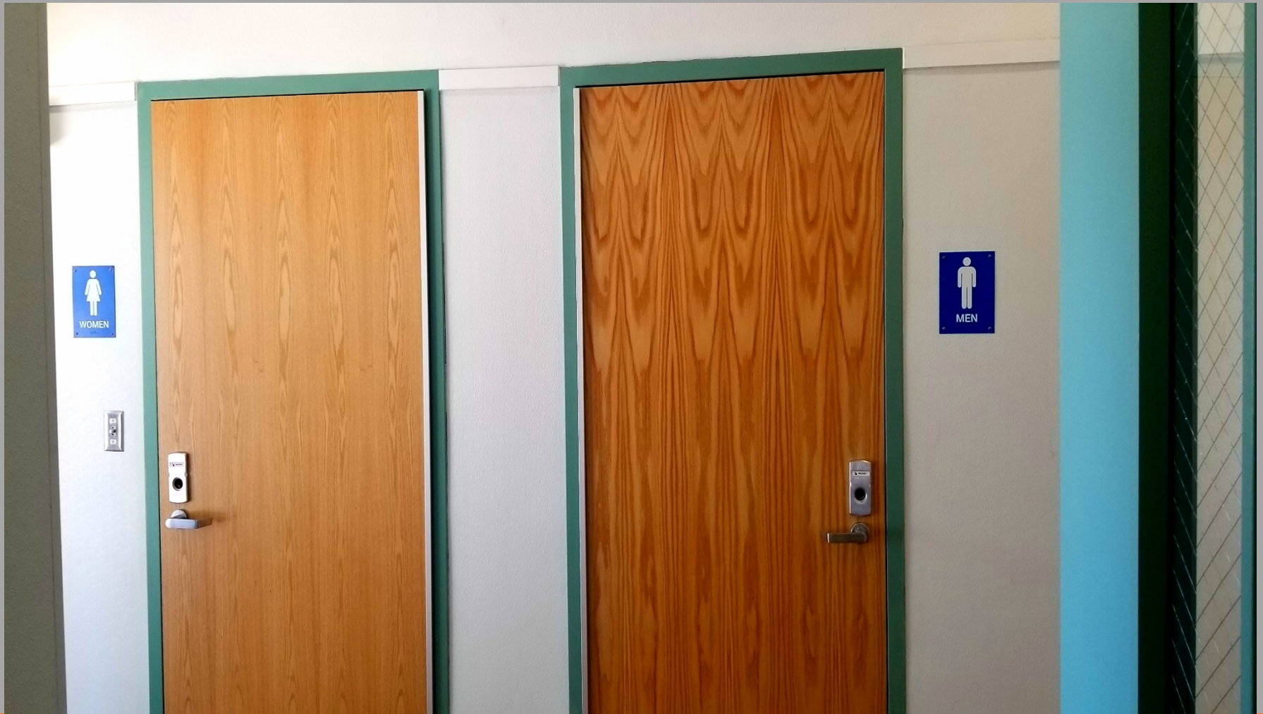
Willow Cove ES - Building E New Bathroom Doors Installed.
