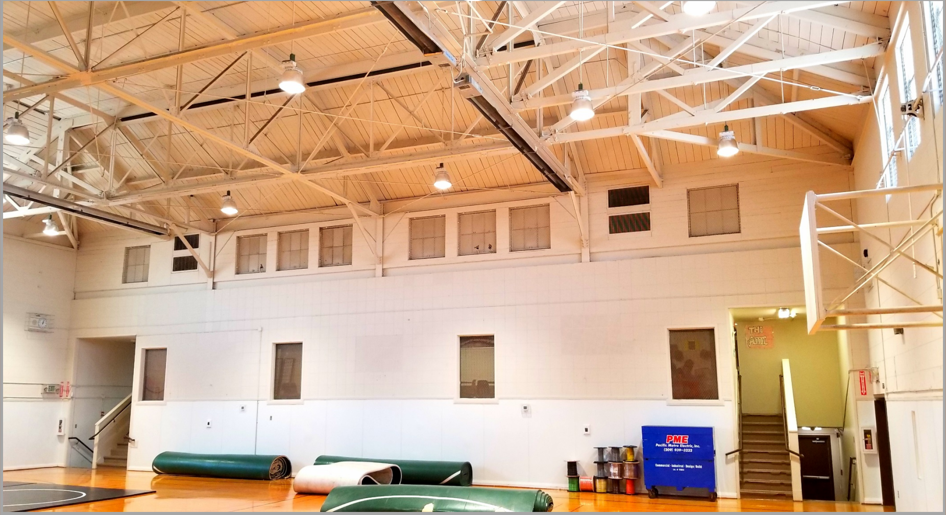
PHS Gym Buildings Lighting Retrofit. Wrestling Gym - Lights installed.
