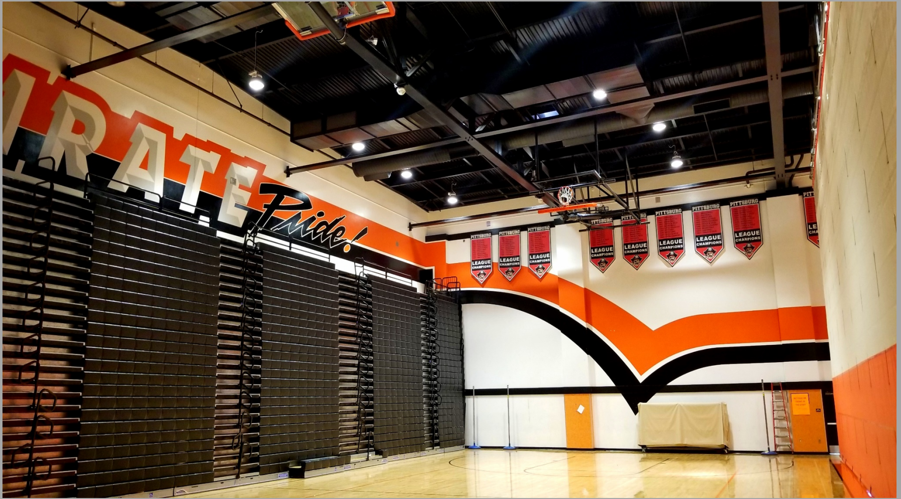
PHS Gym Buildings Lighting Retrofit. Main/New Gym – New Lights installed.
