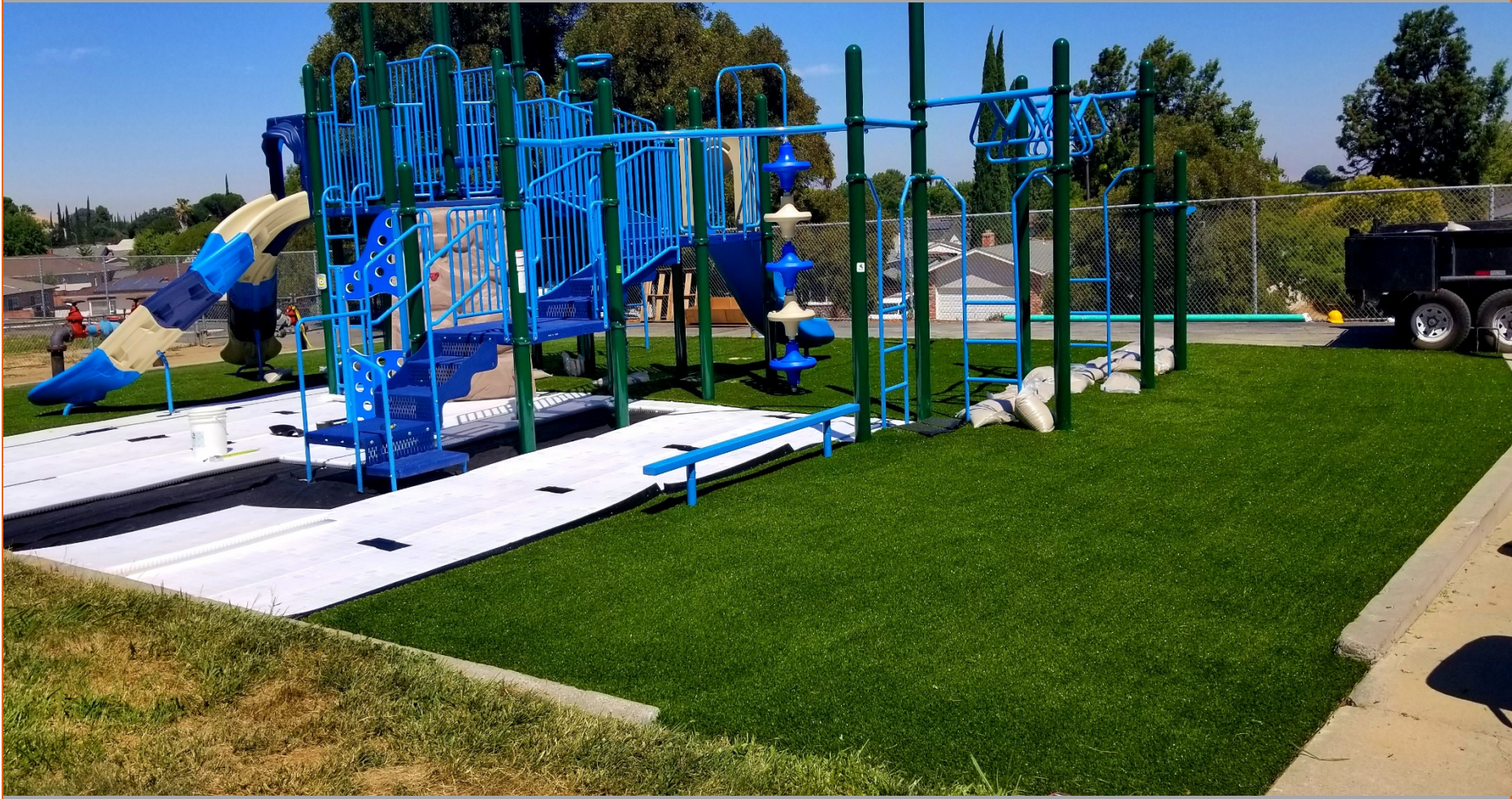
Foothill ES New Play Structure - Turf installed.
