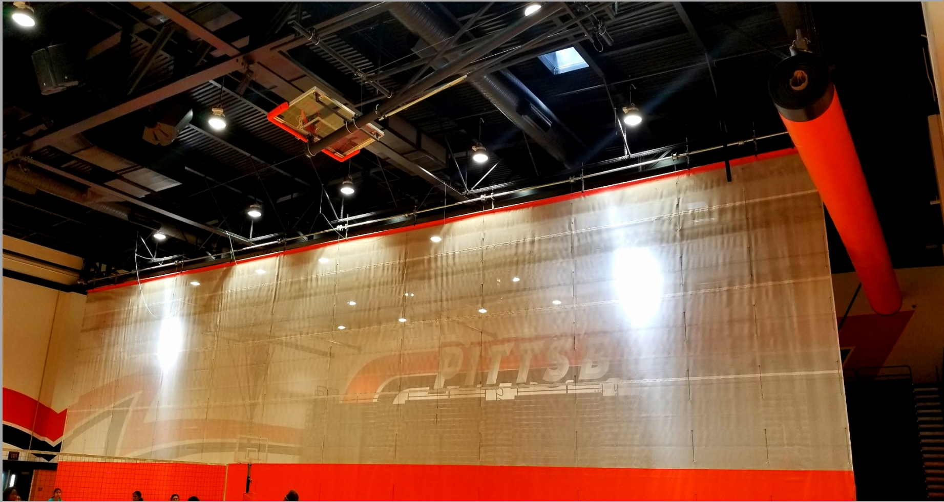
PHS Gym Buildings Lighting Retrofit. Main/New Gym - Bright, well-lit.
