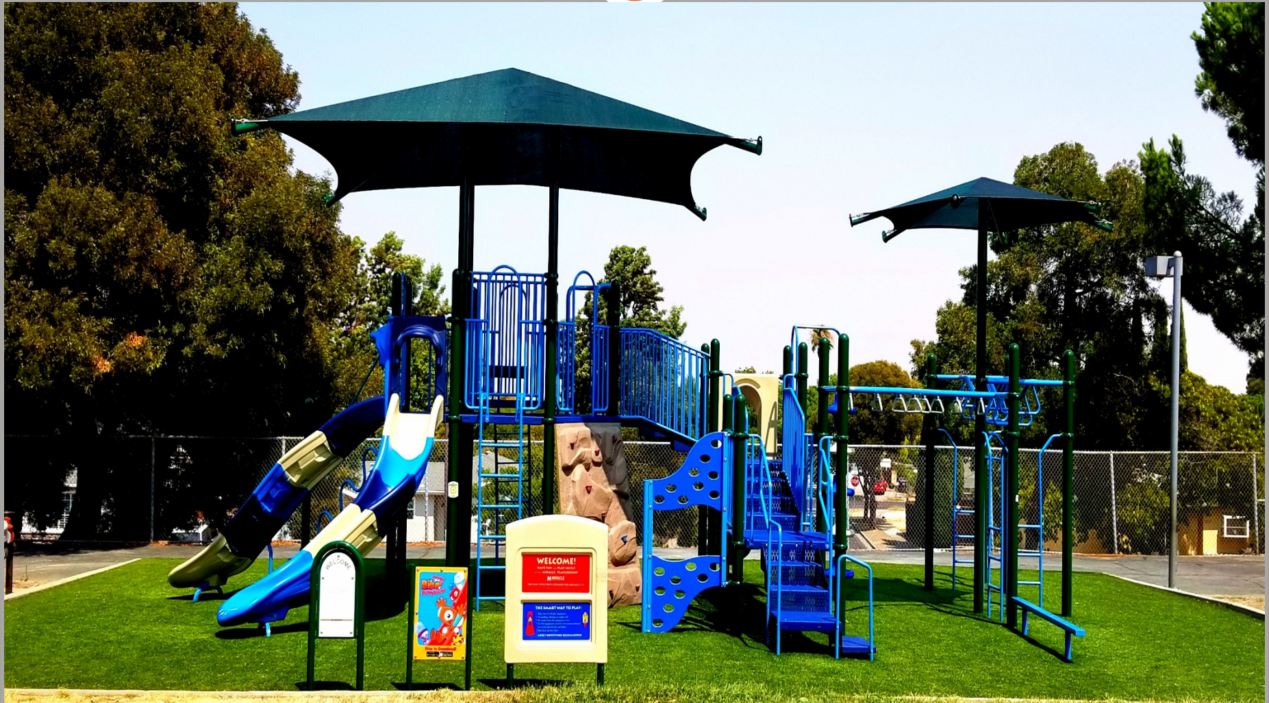
Play Structures Project at Foothill ES: Equipment is 100% completed.
