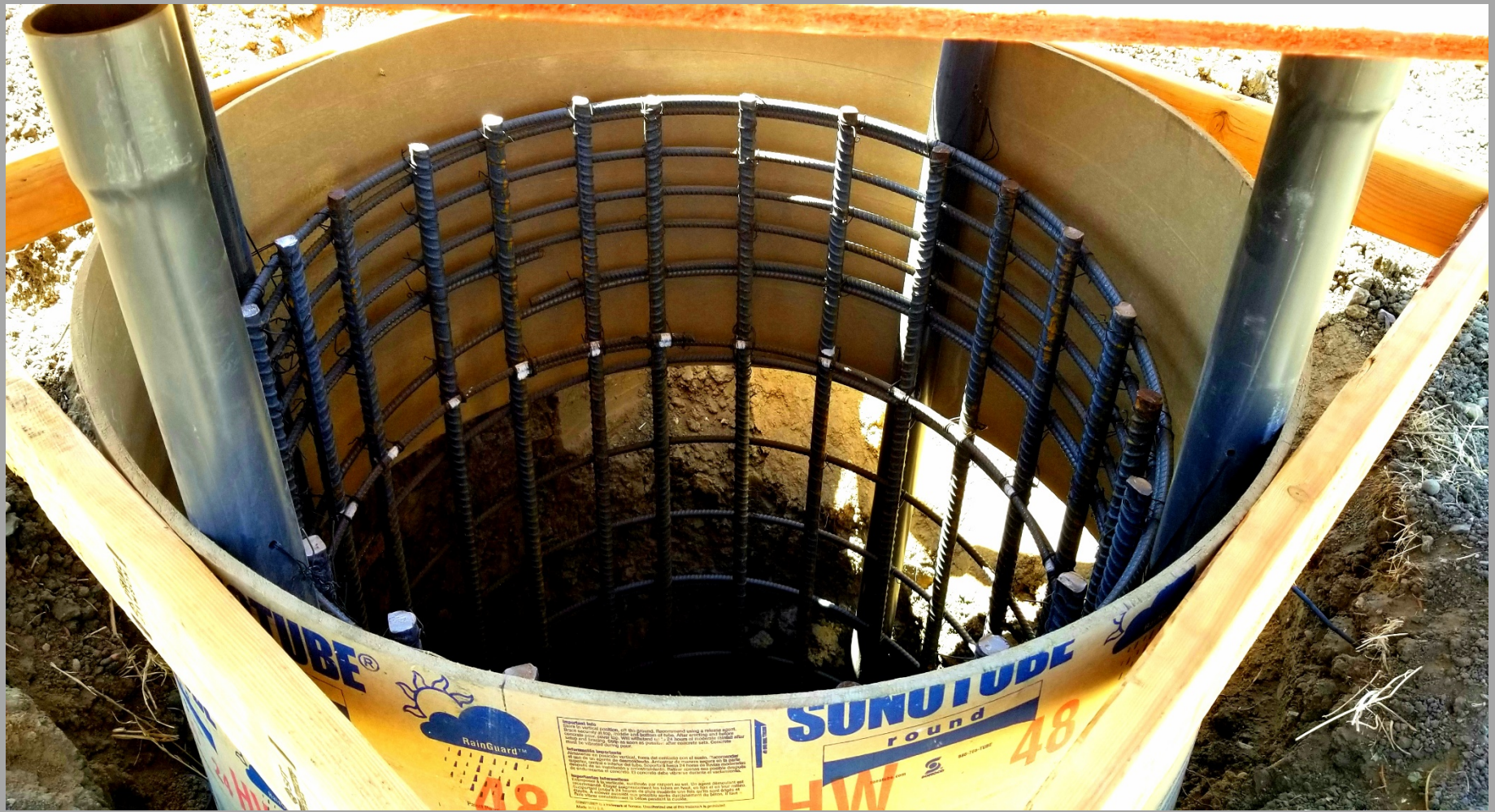
Footing/foundation for Wind Turbine
