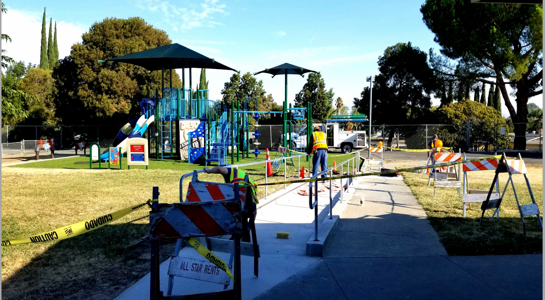
Handrails for Play Structures installed
