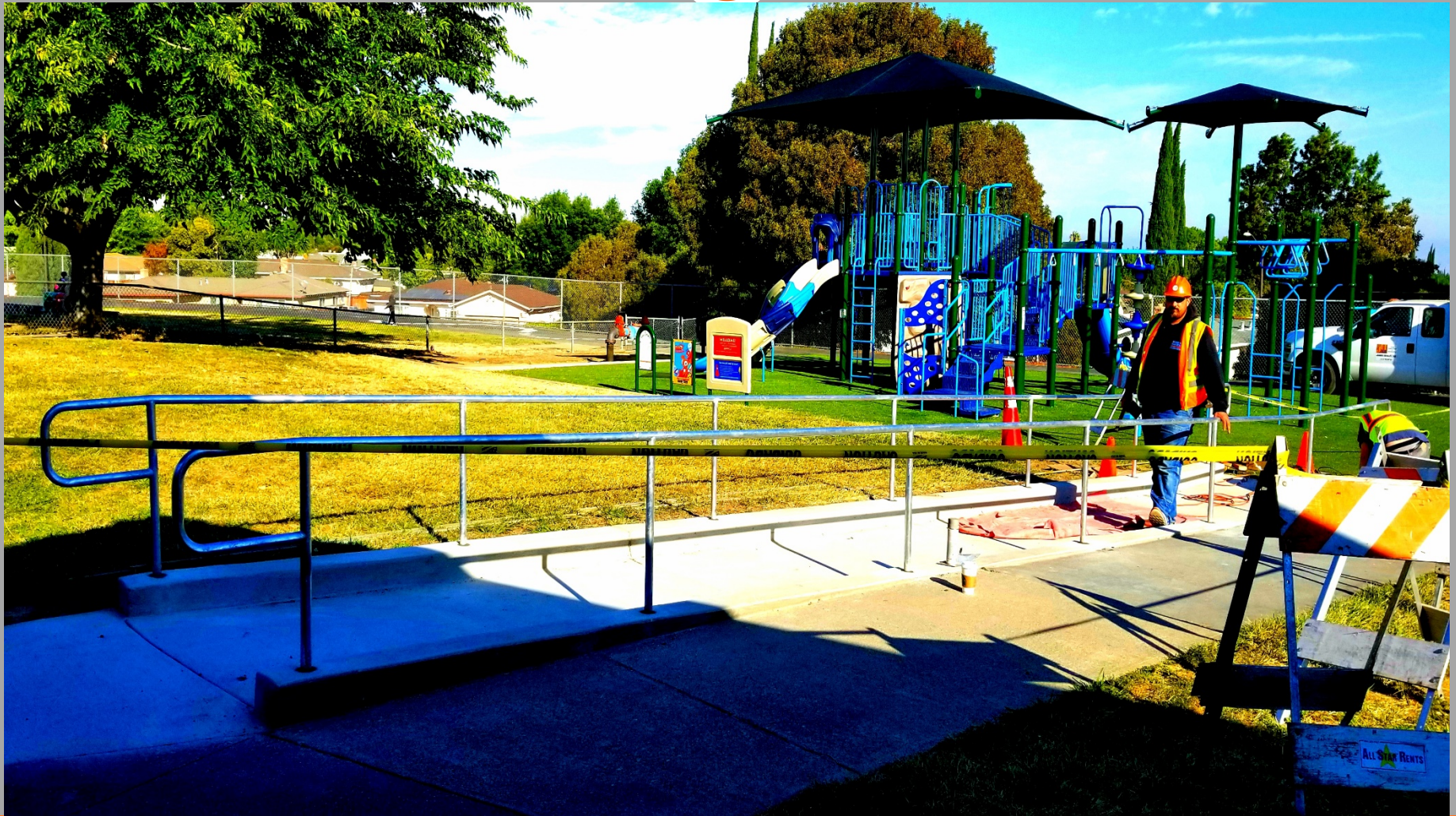
Handrails for Play Structures at a different angle
