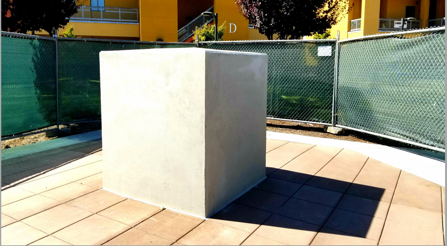
Concrete of Pedestal, another angle
