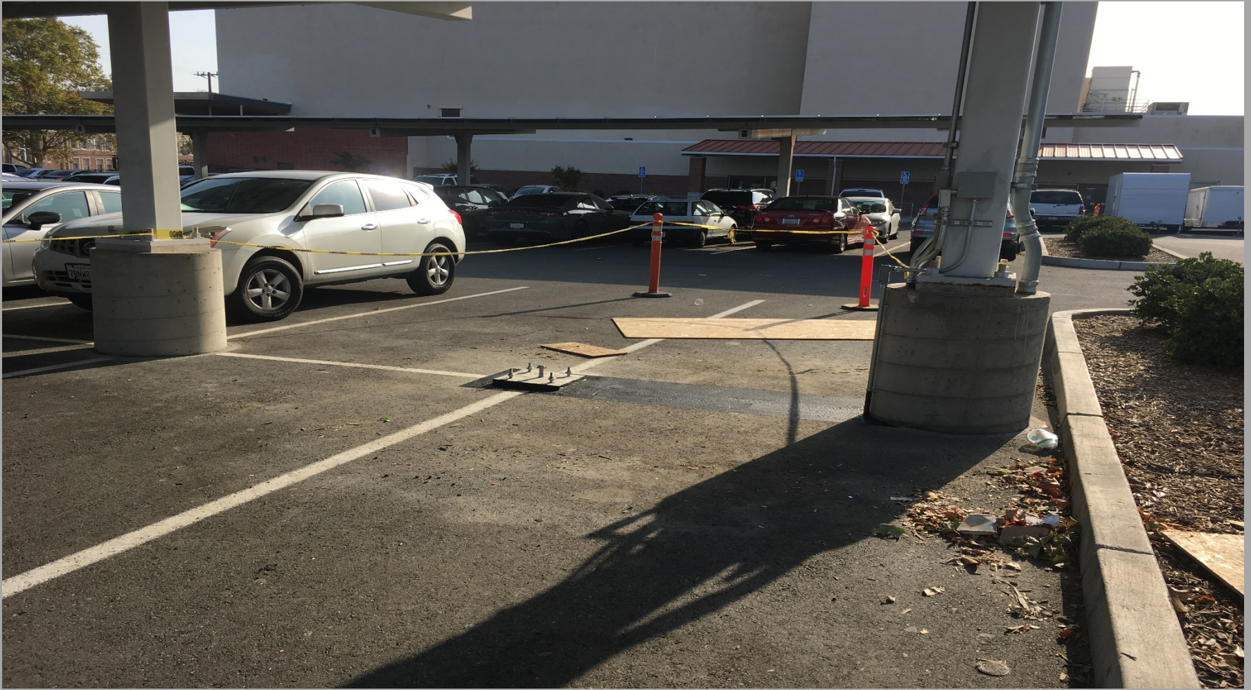
View of Dual Head Charging Station Concrete Pedestal
