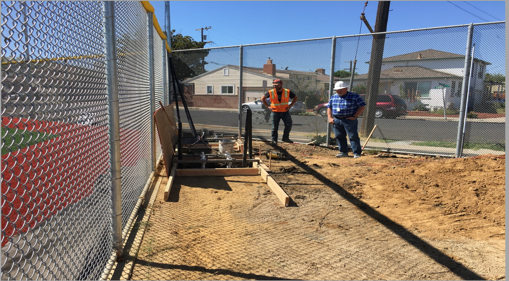
View of Formwork for Baseball Scoreboard Structure Footings
