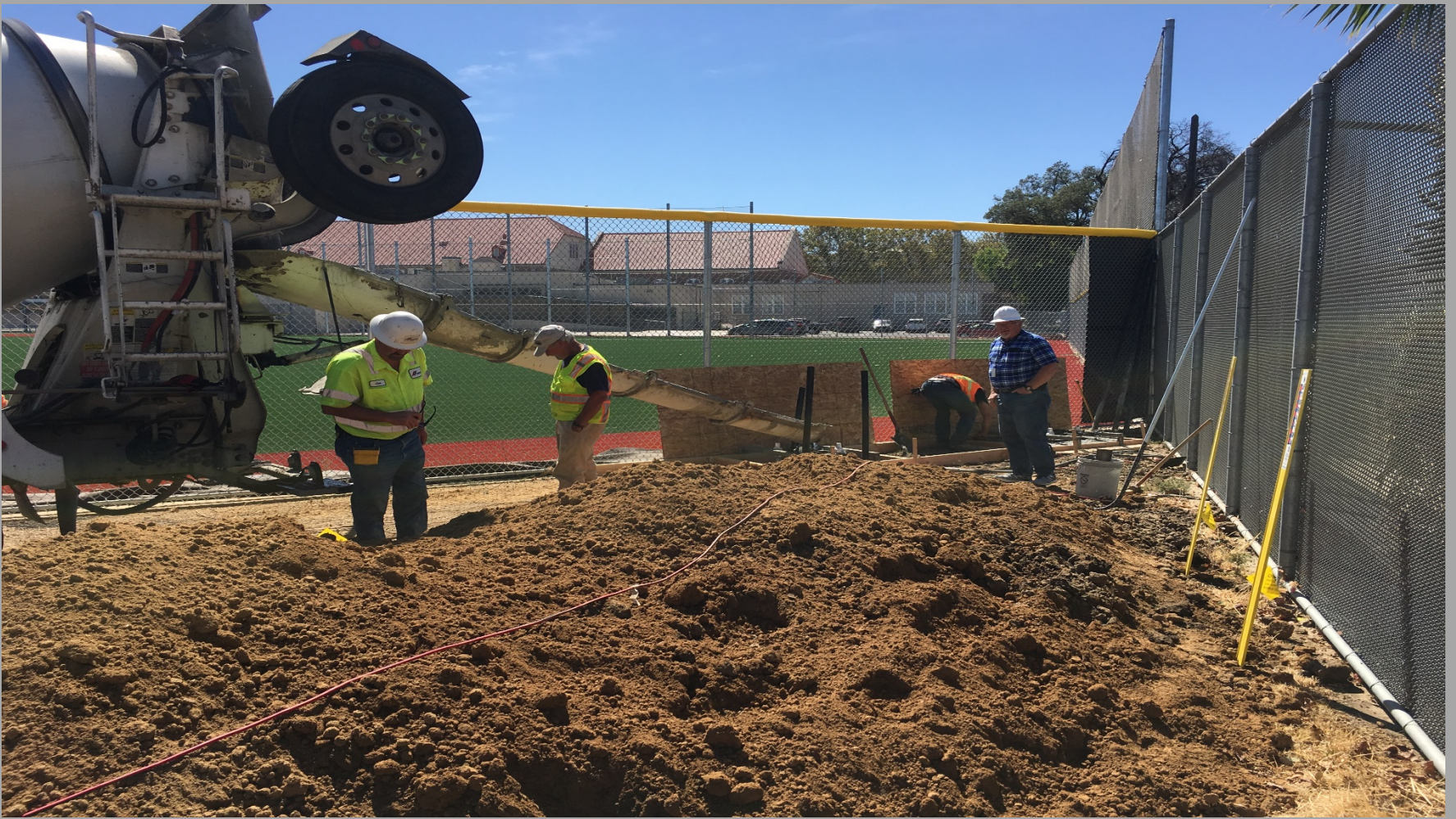
View of Concrete Pour @ Baseball Scoreboard Structure Footings
