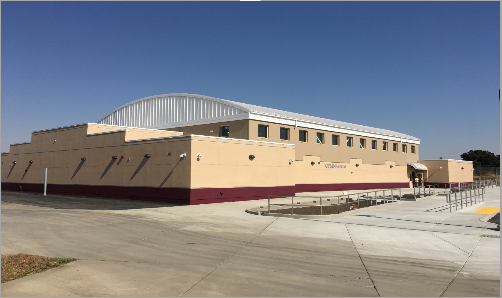
View of New Building Looking Northeast
