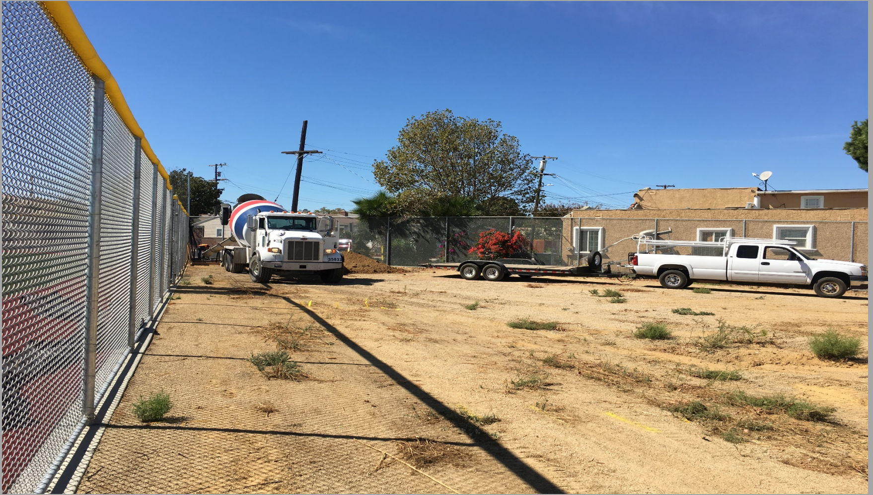
View of Concrete Pour @ Baseball Scoreboard Structure
