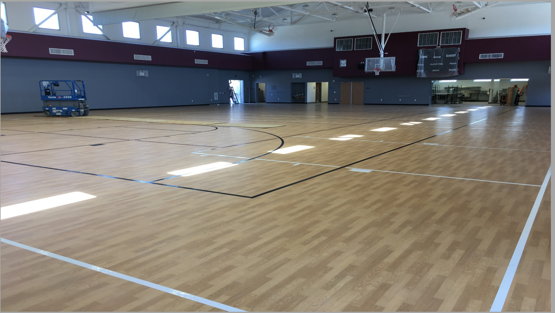
View of Completed Flooring Installation in Gym./MP Space
