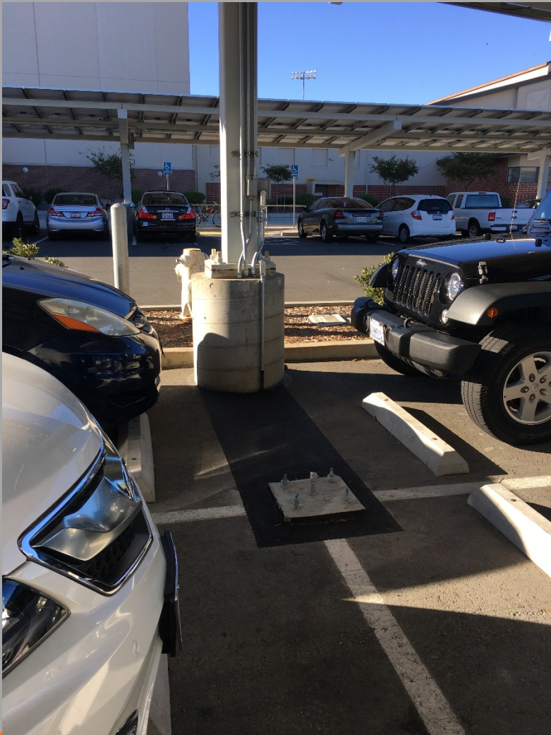
View of Concrete Pedestals for EV Charging Stations
