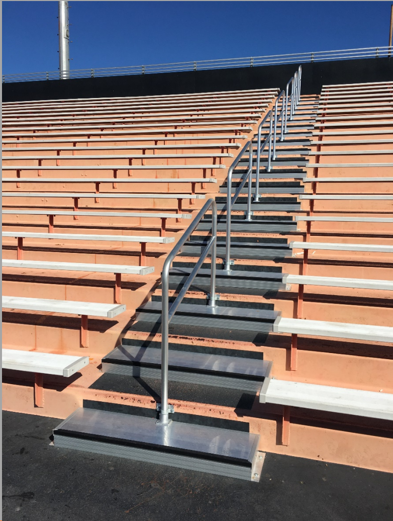
Up-close View of Added Handrails and Steps at Visitor Side Grandstand
