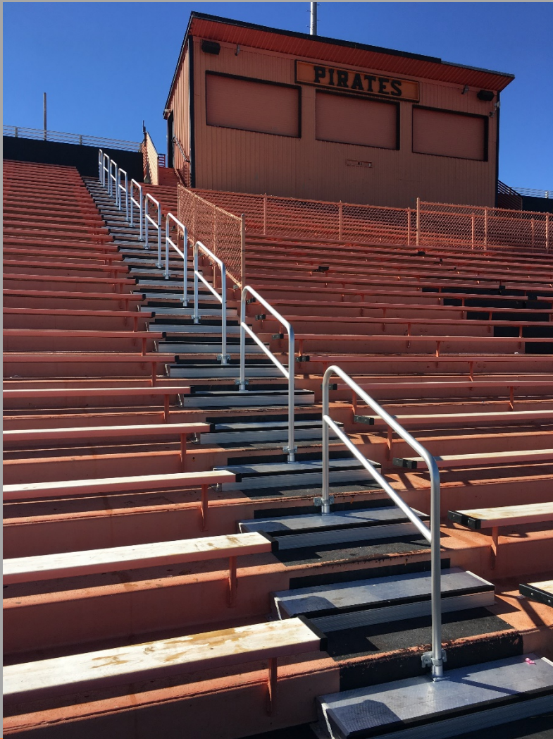
Up-close View of Added Handrails and Steps at Home Side Grandstand
