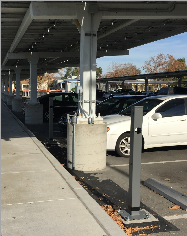
View of Pedestals for EV Charging Stations – Chargers to be Installed
