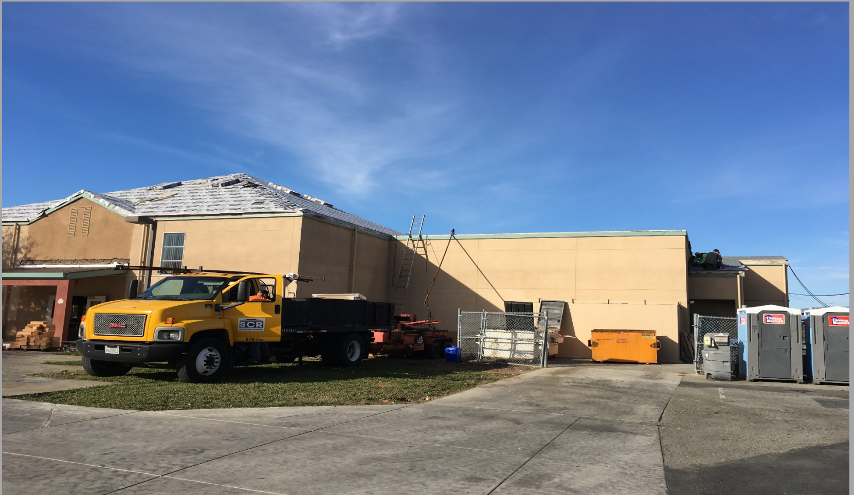
View of Roofing Replacement Work @ Building E - Looking North
