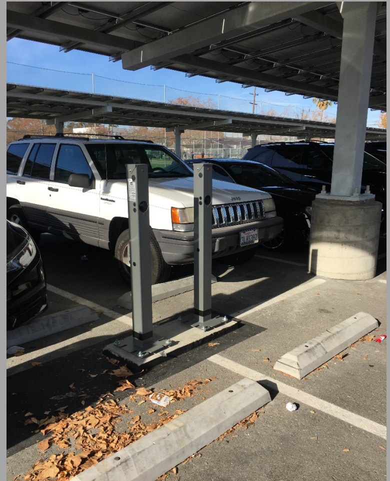
View of Pedestals for EV Charging Stations – Chargers to be Installed
