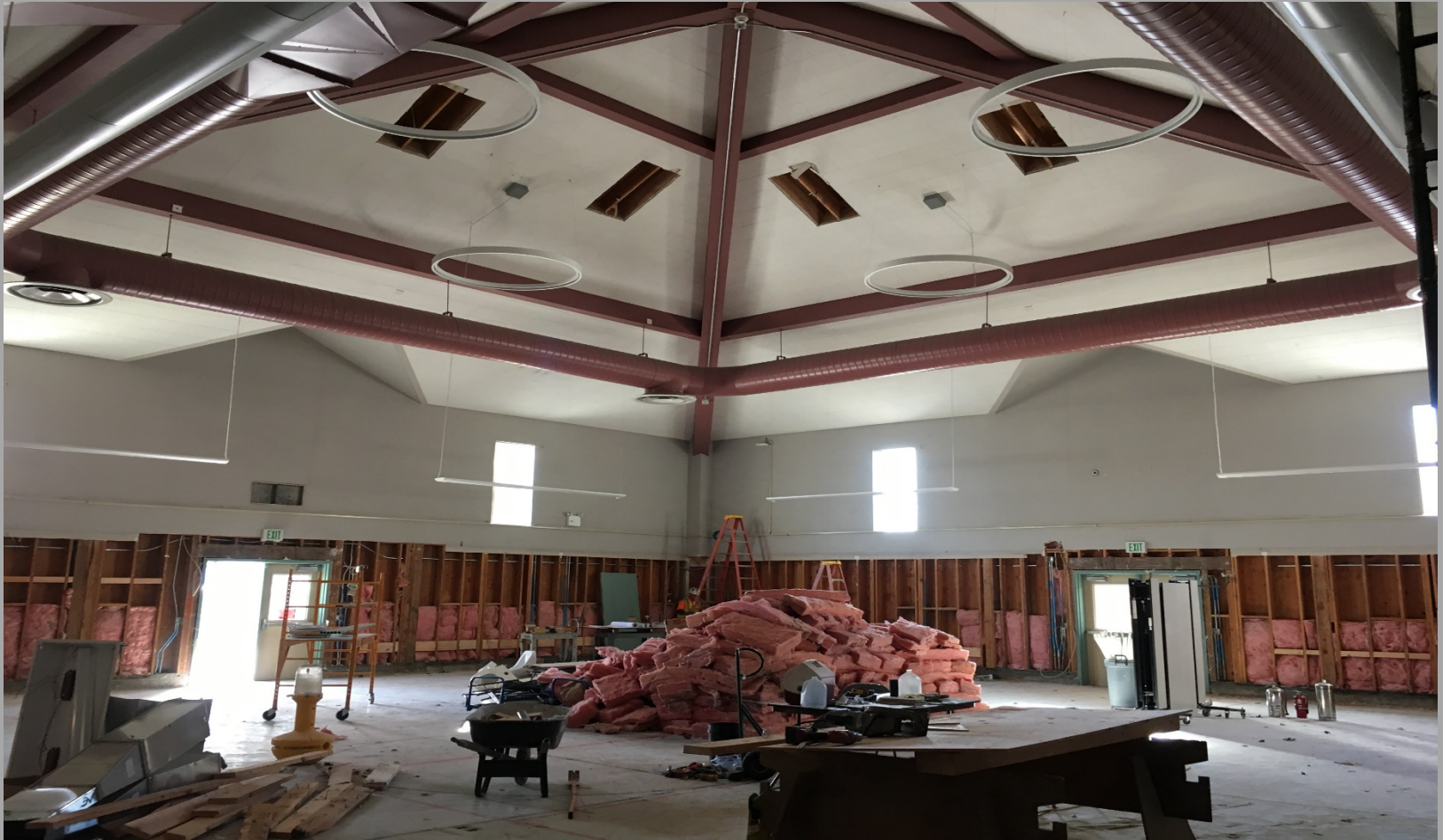
View of Demolition Inside of Building E – Looking Southwest
