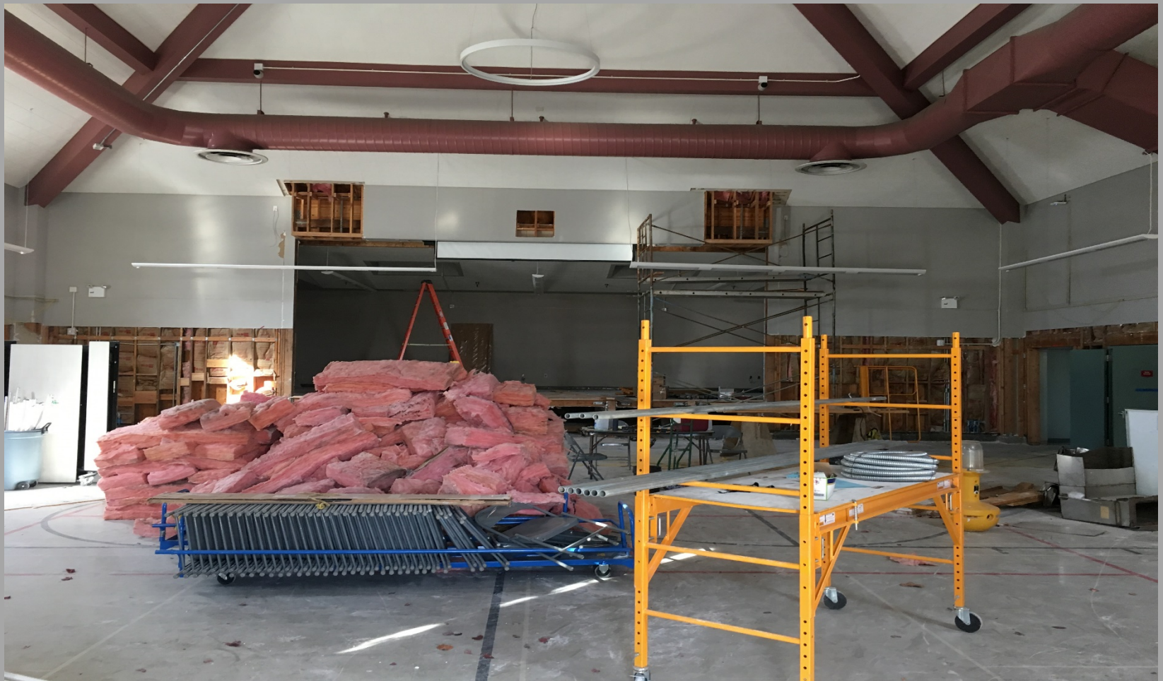
View of Demolition Work Inside of Building E - Looking North
