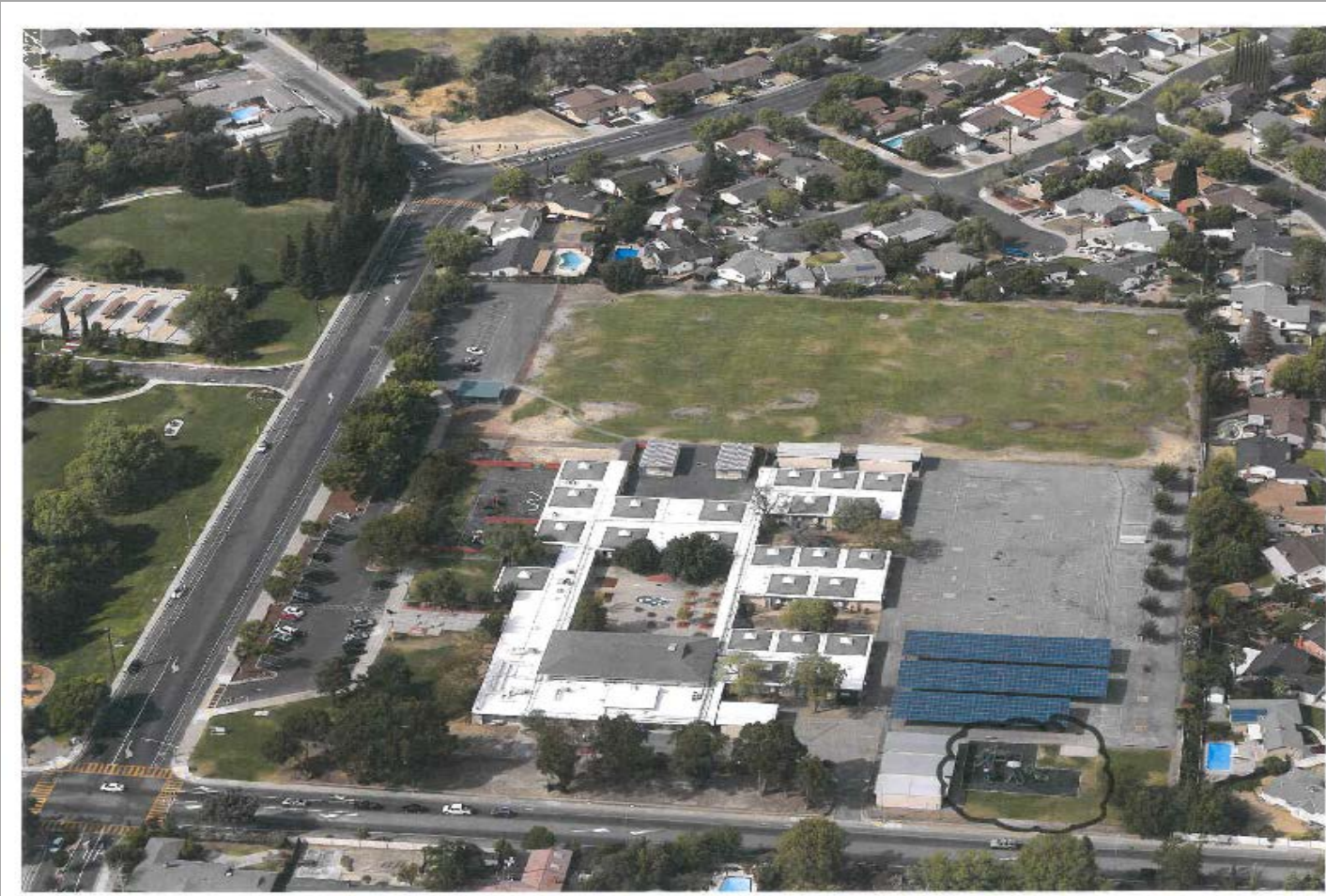
Arial View of Upper Grades Play Structure Location @ Highlands ES
