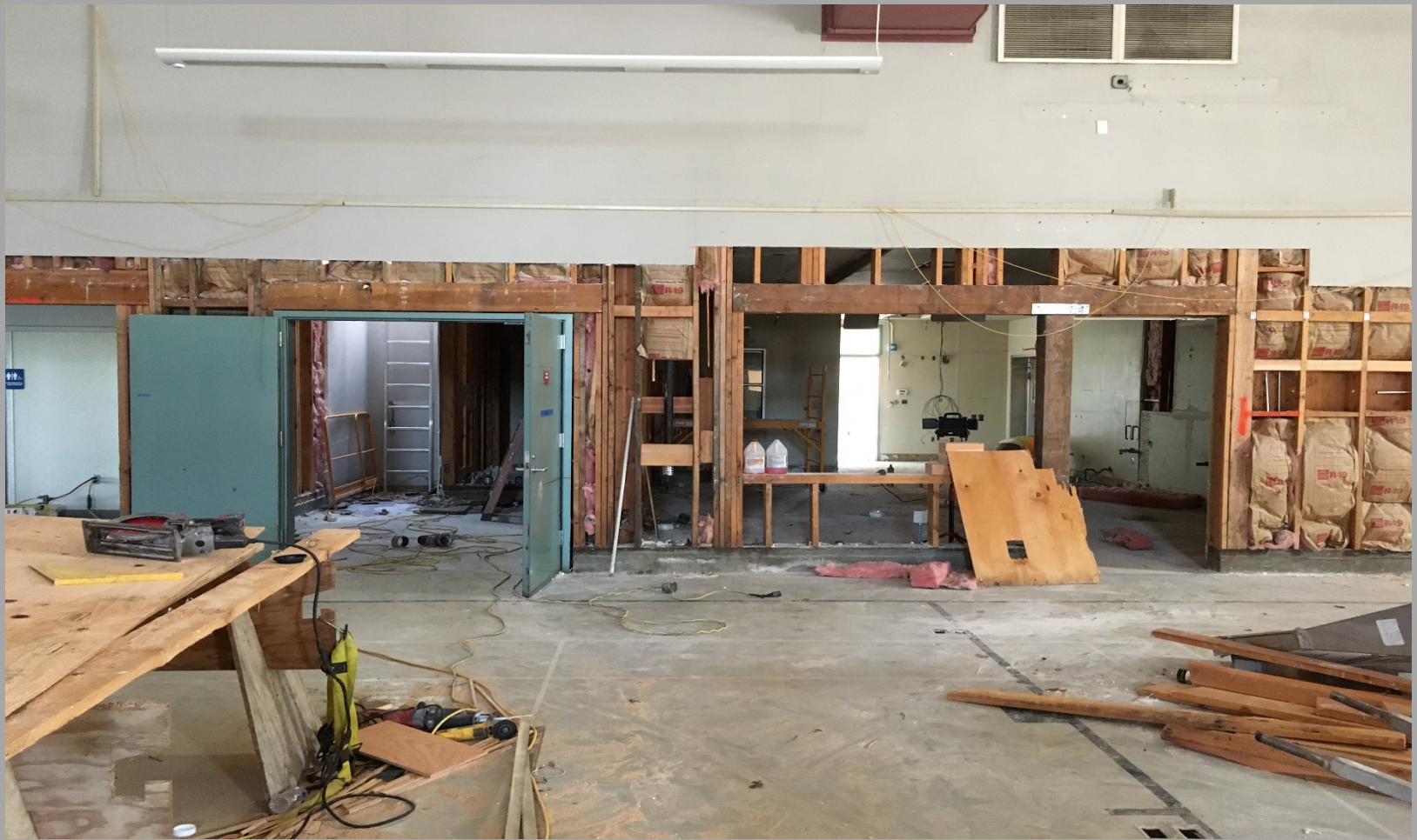
View of Demolition Inside of Building E - Looking East
