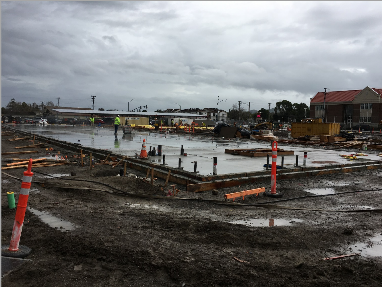
New 12 Classrooms Bldg. (Bldg. N1) Slab Poured - Looking Southeast
