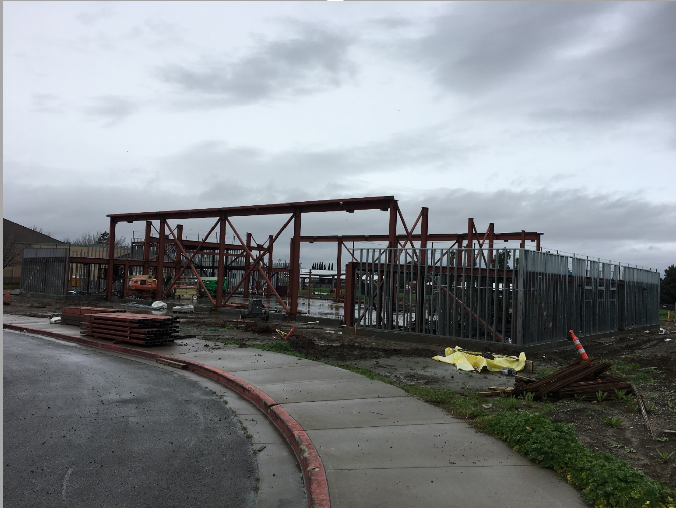
New Gym./MP Bldg. Structural Steel & Exterior Walls Framing Ongoing - Looking Northwest
