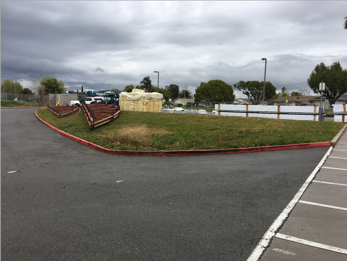
New Gym./MP Bldg. Roof Trusses On Site and Ready for Installation
