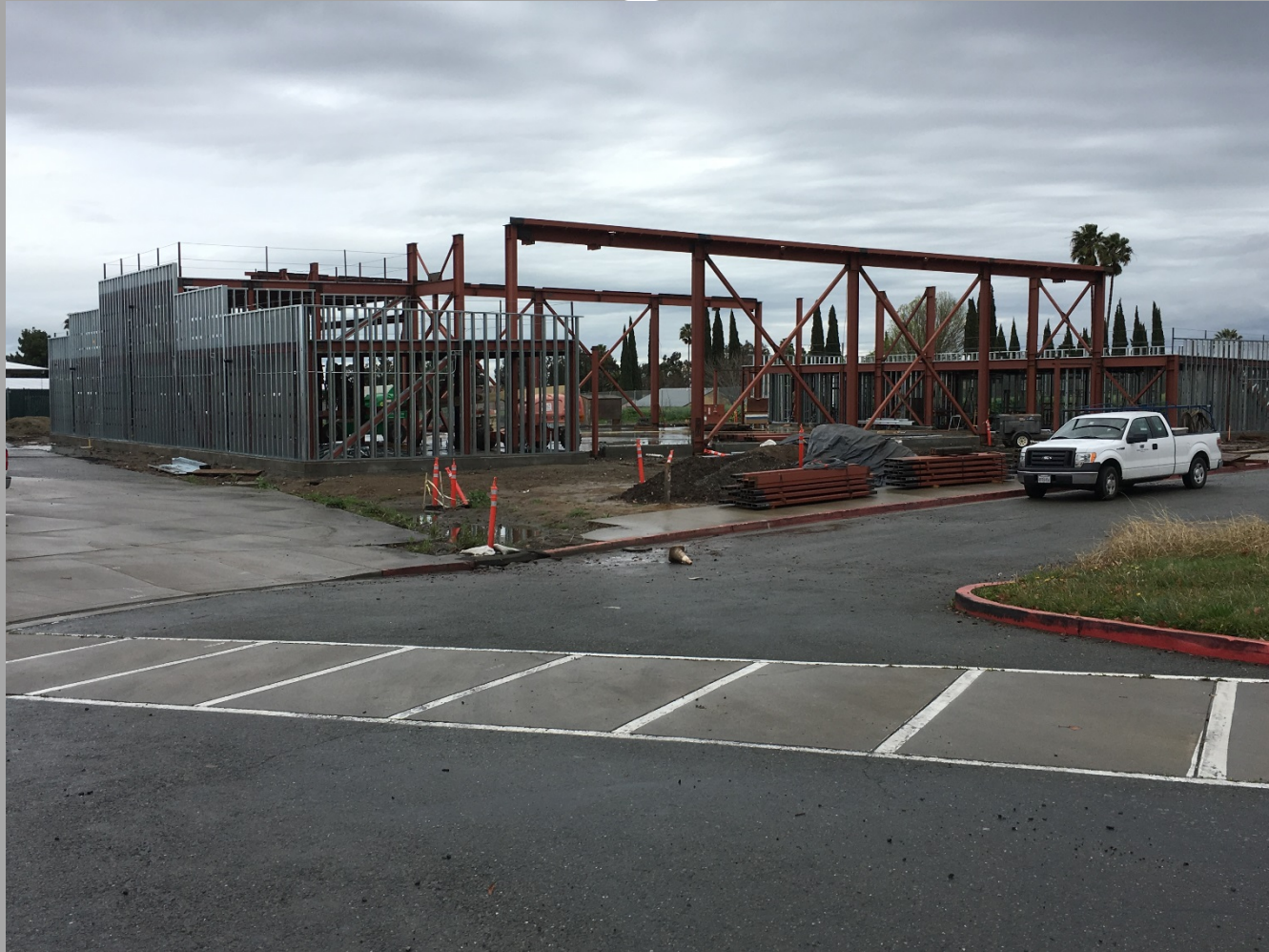
New Gym./MP Bldg. Structural Steel & Exterior Walls Framing Ongoing- Looking Northeast
