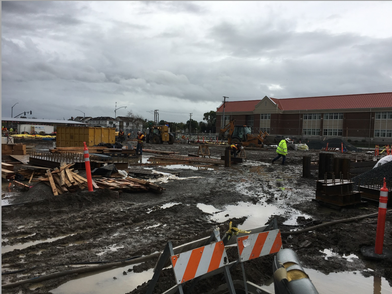
New Classrooms Bldgs. Site Utilities & Footings Preparation Ongoing – Looking Southeast
