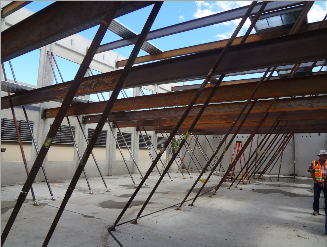
View Of Structural Steel Inside Of Building N1
