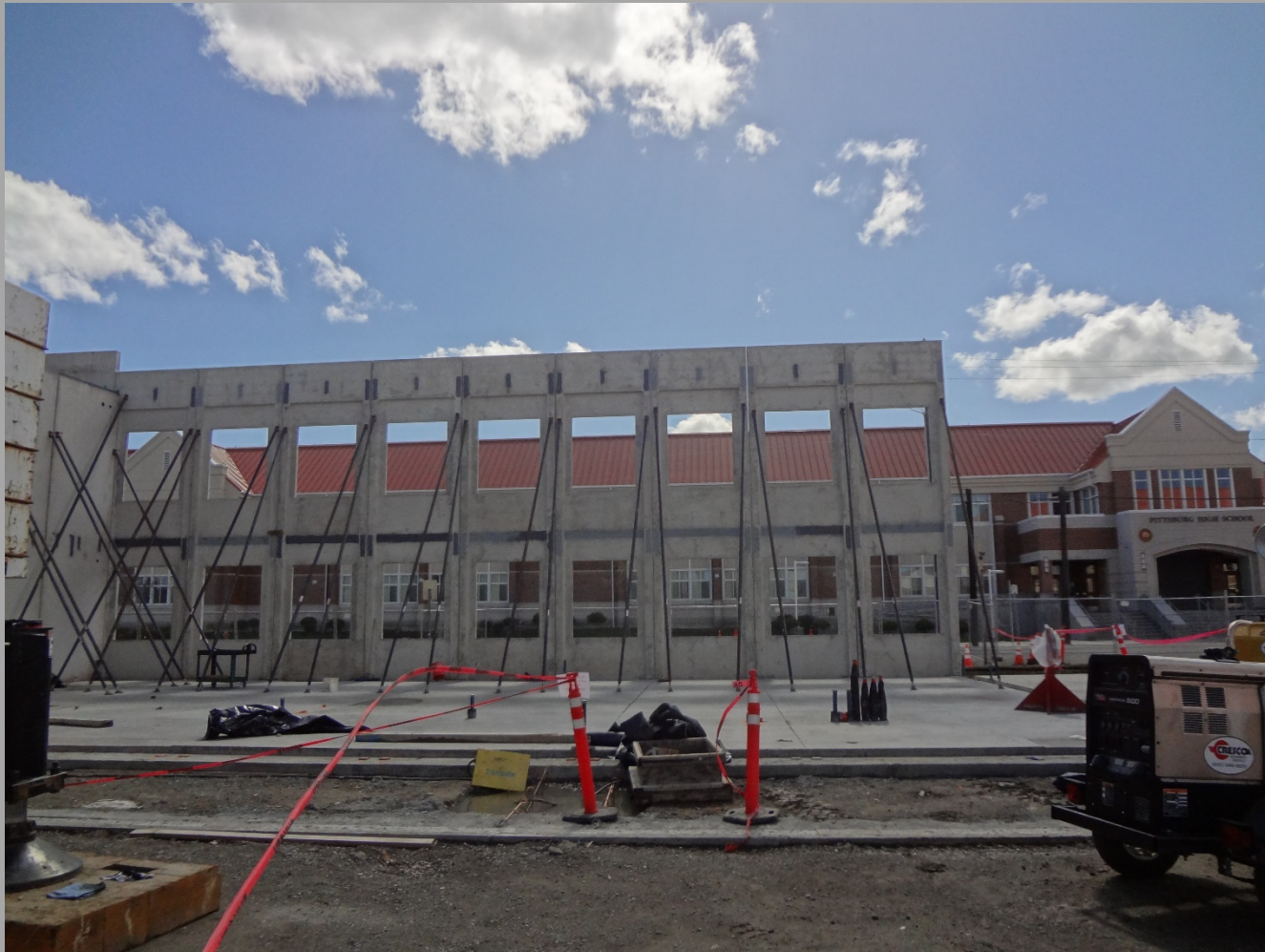
New 8 Classrooms Bldg. (Bldg. N3) South Exterior Wall Panels In Place
