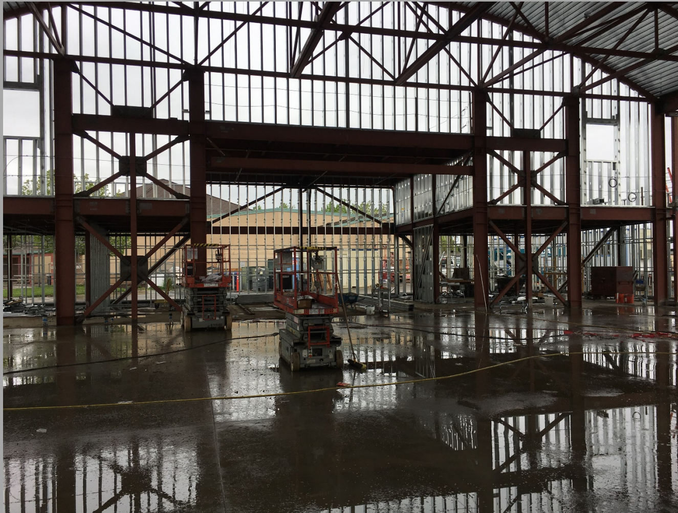
New Gym/MP Bldg. Interior View Of West Wall Gym/MP Space Wall
