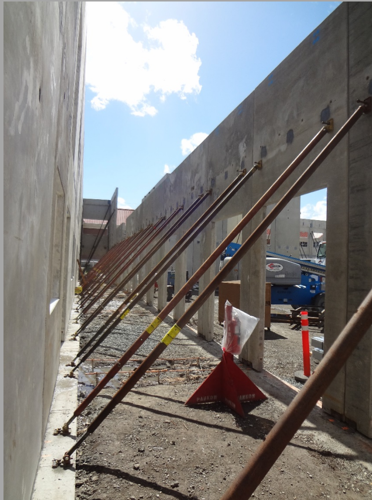
New 10 Classrooms Bldg. (Bldg. N2) View Of Walkway Panels In Place
