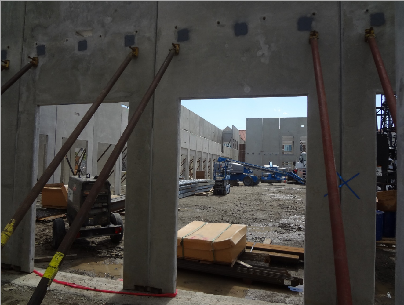
View Of Buildings N2 & N3 From Building N1 Walkway Looking South
