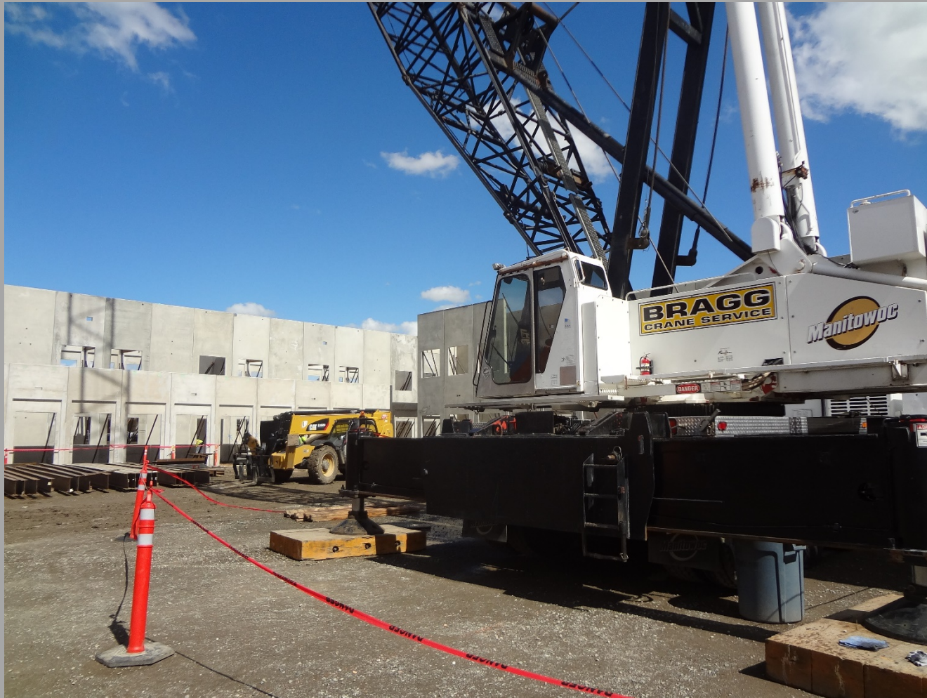
New 12 Classrooms Building (Bldg. N1) South Exterior Wall
