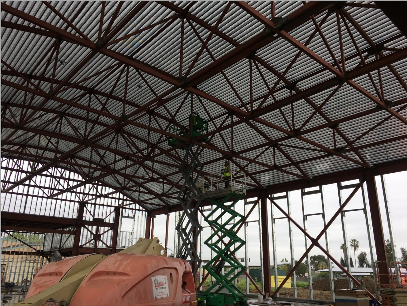
New Gym/MP Bldg. Interior View Of Gym/MP Space Roof
