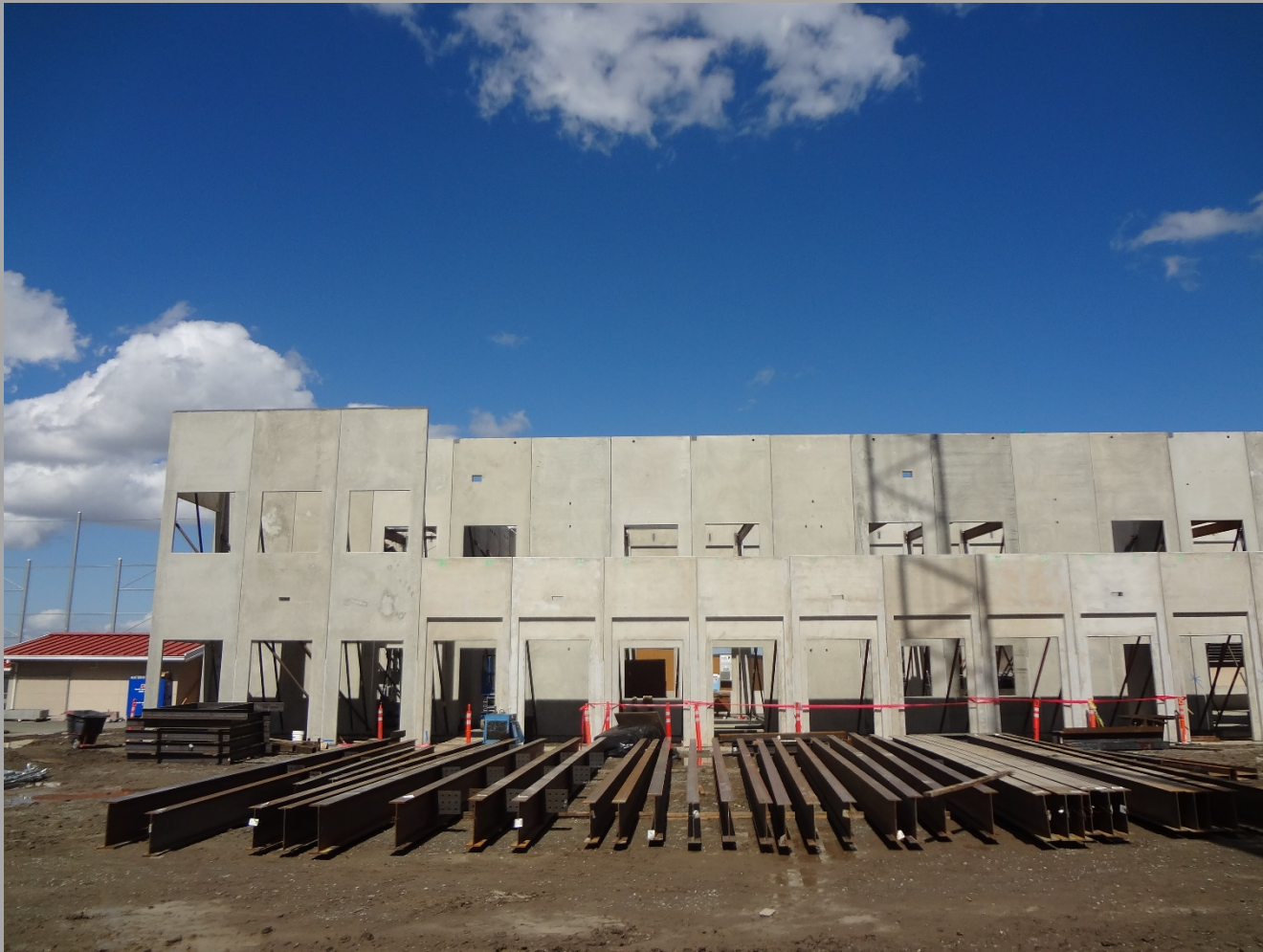
New 12 Classrooms Bldg. (Bldg. N1) South Exterior Wall Panels In Place
