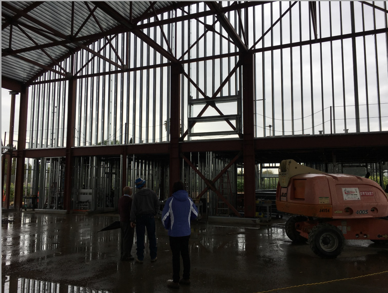
New Gym/MP Bldg. Interior View Of East Gym/MP Space Wall
