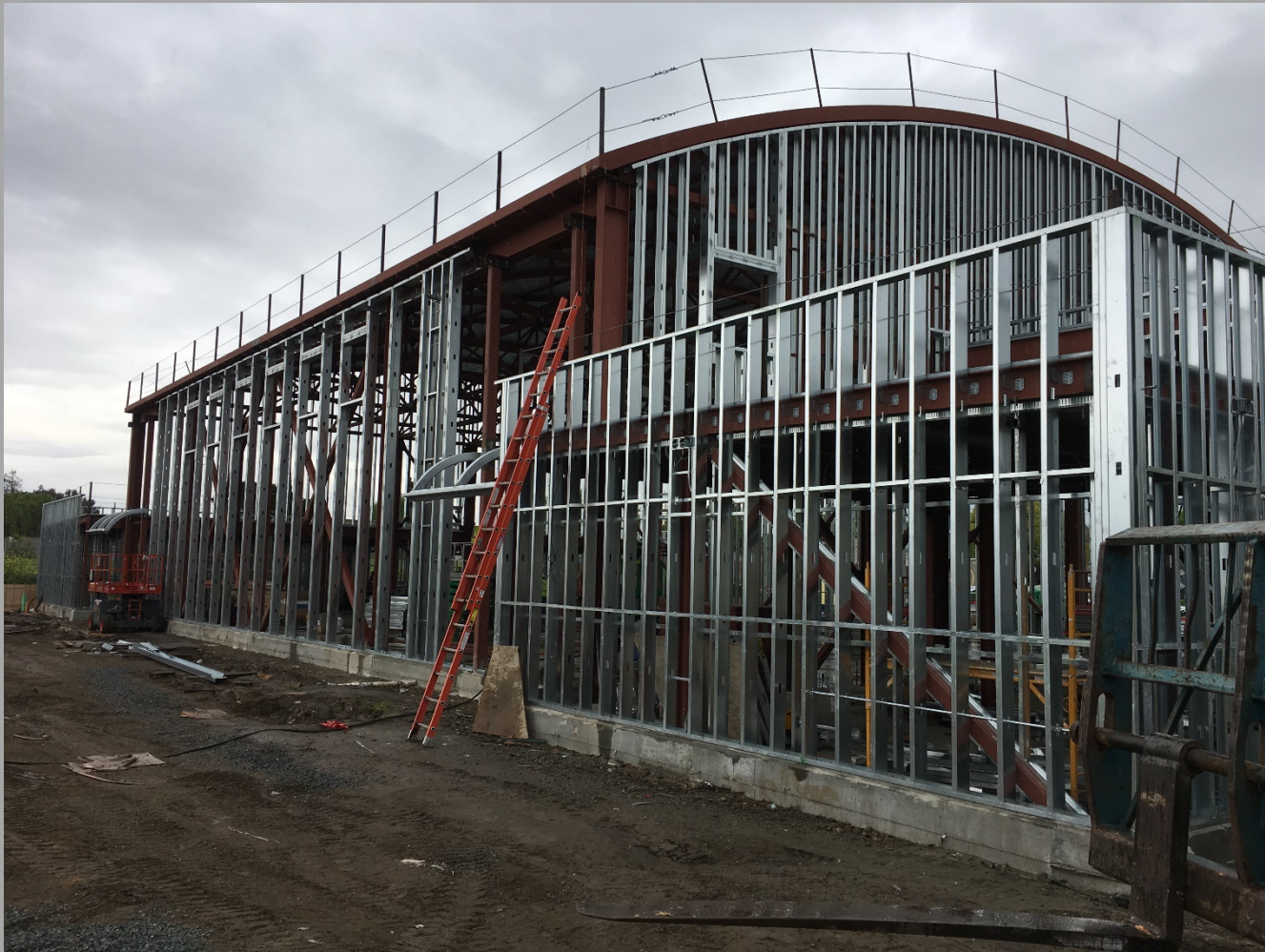
New Gym/MP Bldg. Exterior Walls Framing Ongoing- Looking Southeast
