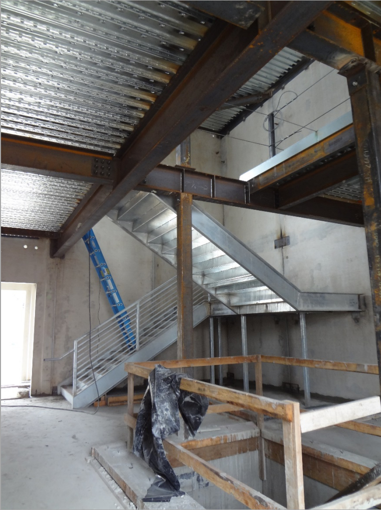
Left: New 12 Classrooms Building (Bldg. N1) Staircase Installed Adjacent To Elevator Pit. Right: Shows Stair Pans Already Poured
