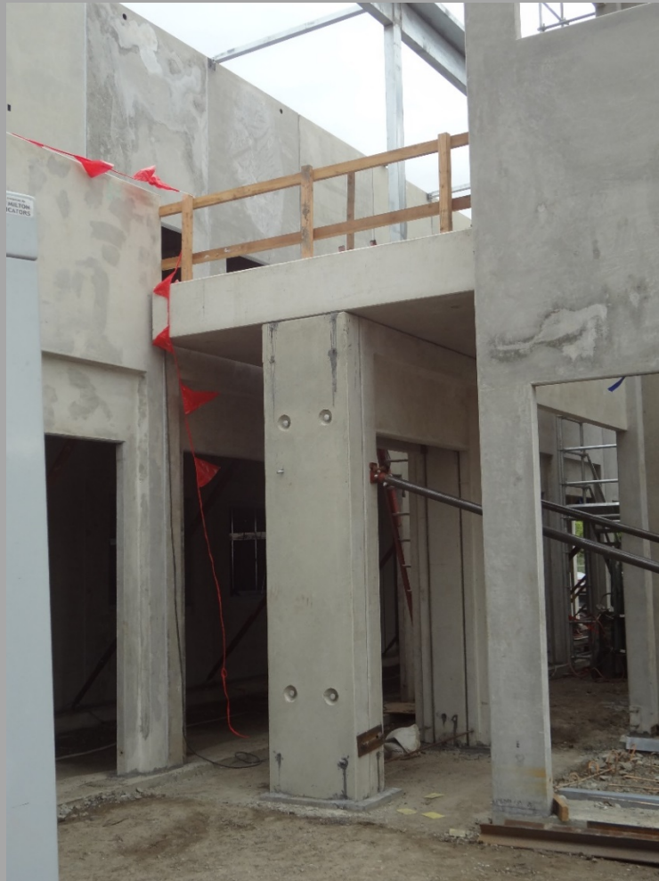
View Of Walkway Bridge Installed Between Building N1 and N2
