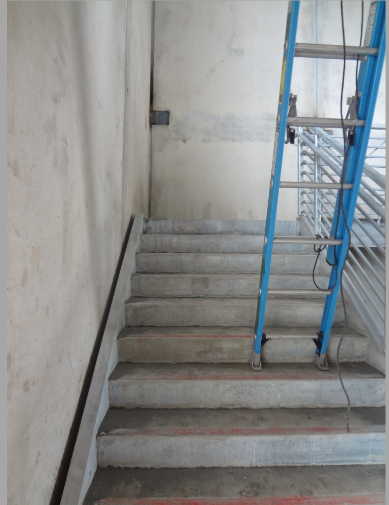
Left: New 12 Classrooms Building (Bldg. N1) Staircase Installed Adjacent To Elevator Pit. Right: Shows Stair Pans Already Poured
