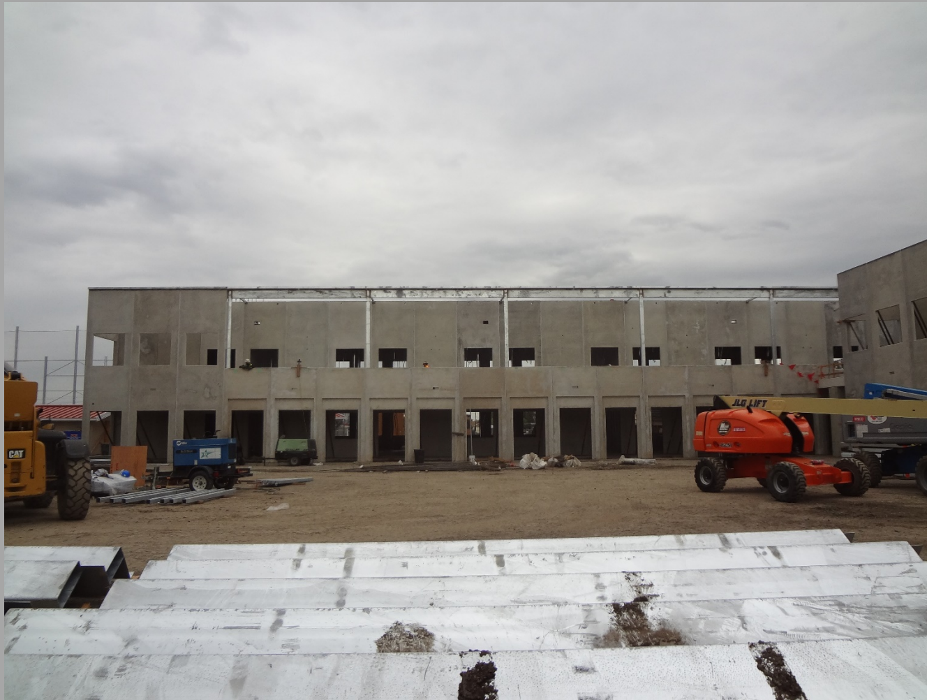
Quad Area View Of Bldg. N1 and N2
