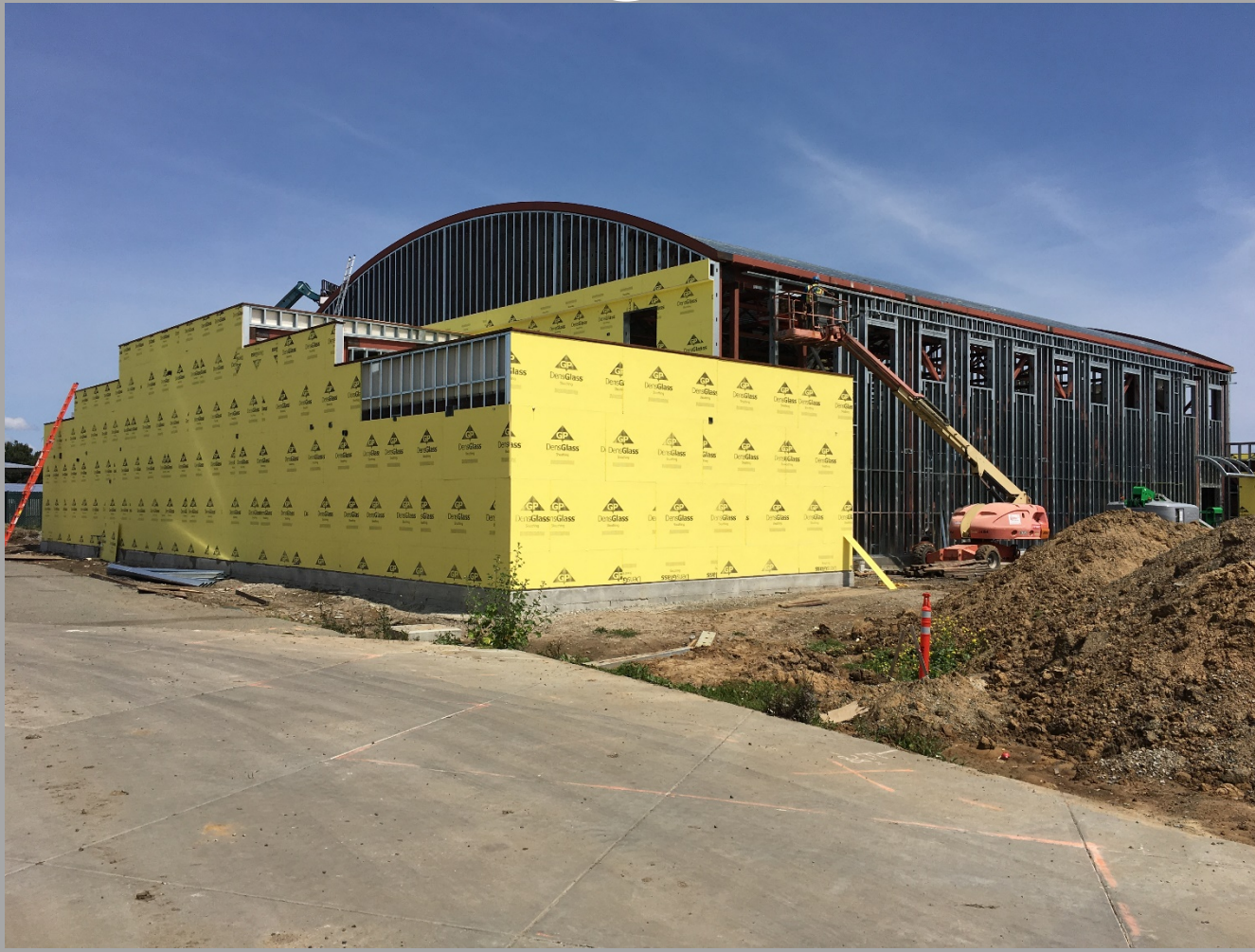
New Gym/MP Bldg. Exterior Wall Insulation Being Installed
