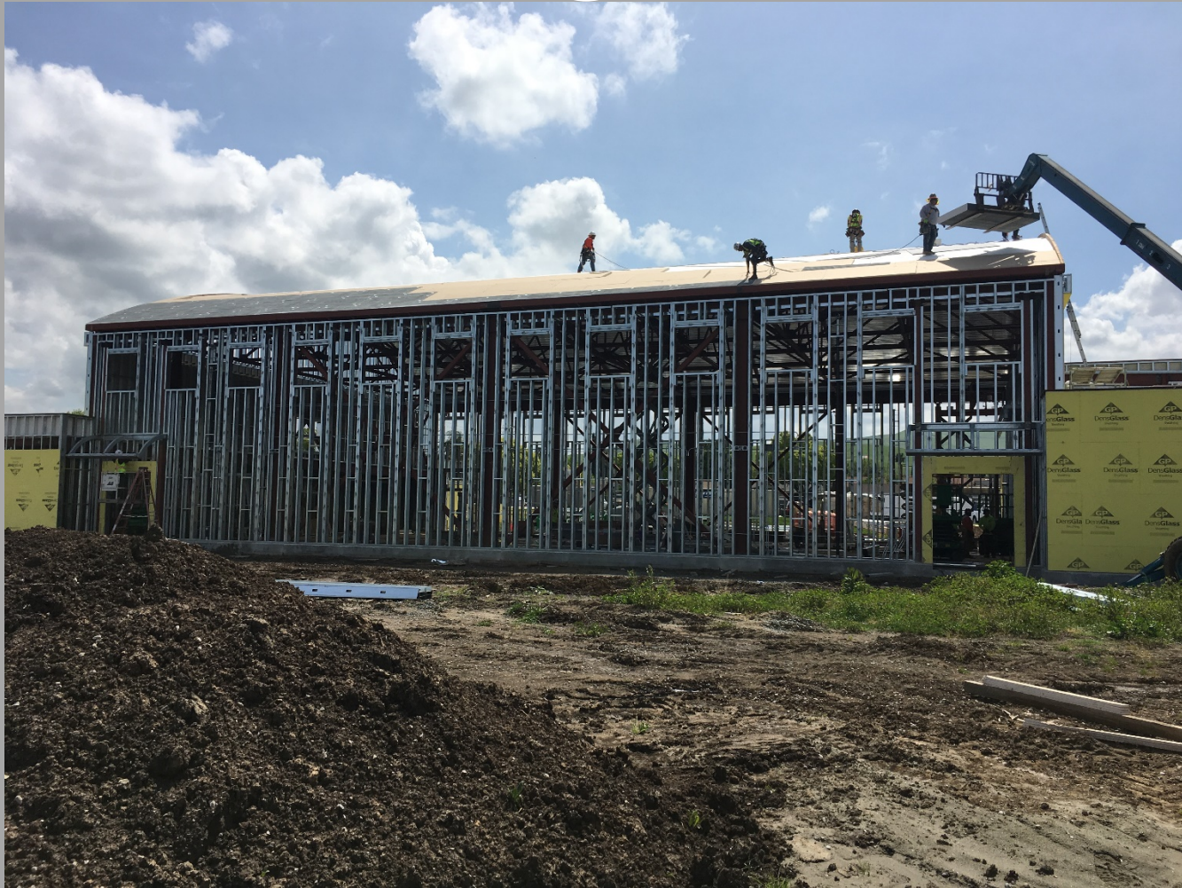
Insulation Being Installed At Gym/MP Roof
