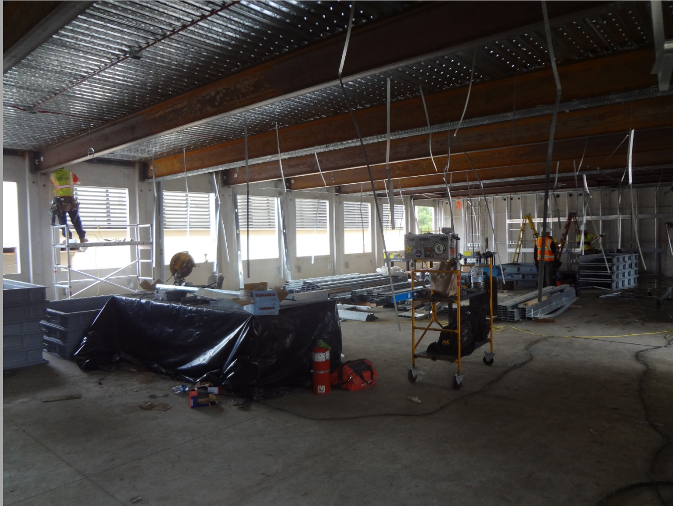
New 8 Classrooms Bldg. (Bldg. N1) Duct Work Installation In Progress
