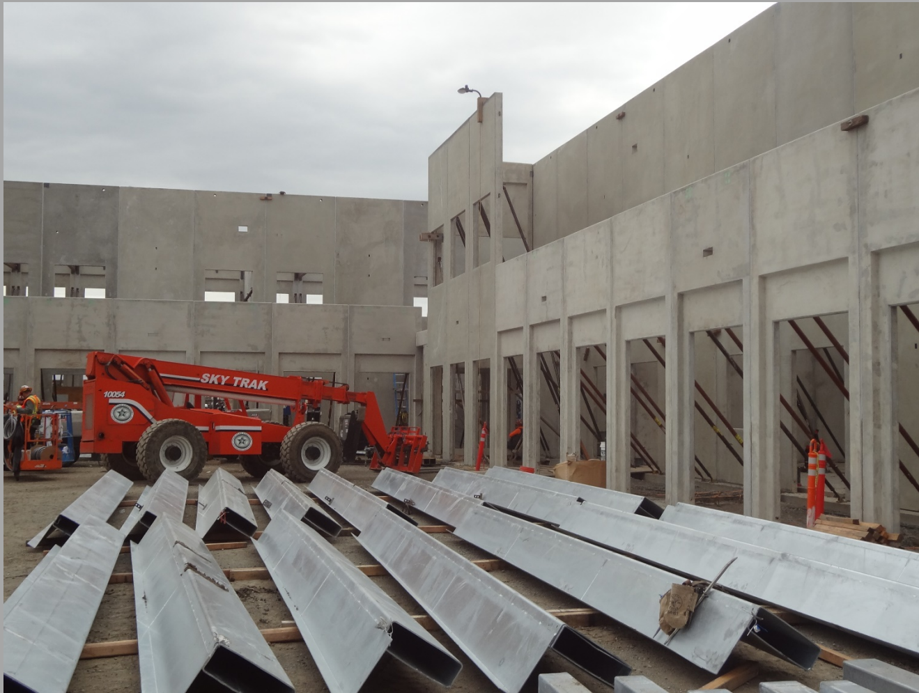
Quad Area View Of N1 and N2, Upper Walkway Steel
