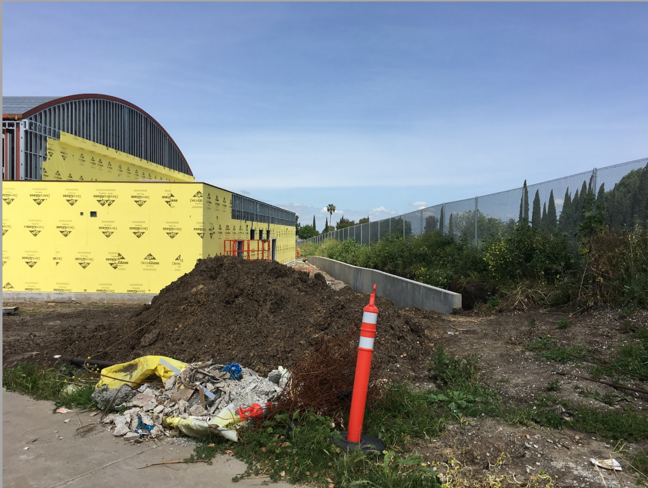
New Gym/MP Bldg. Kitchen Loading Area Retaining Wall Has Been Poured
