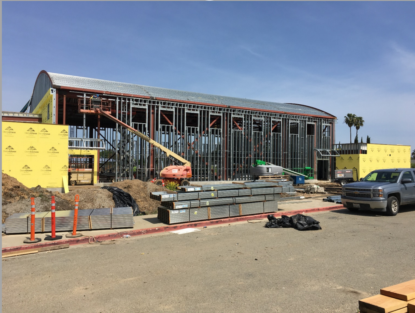
New Gym/MP Bldg. Roof Decking In Place & Exterior Walls Framing Continuing
