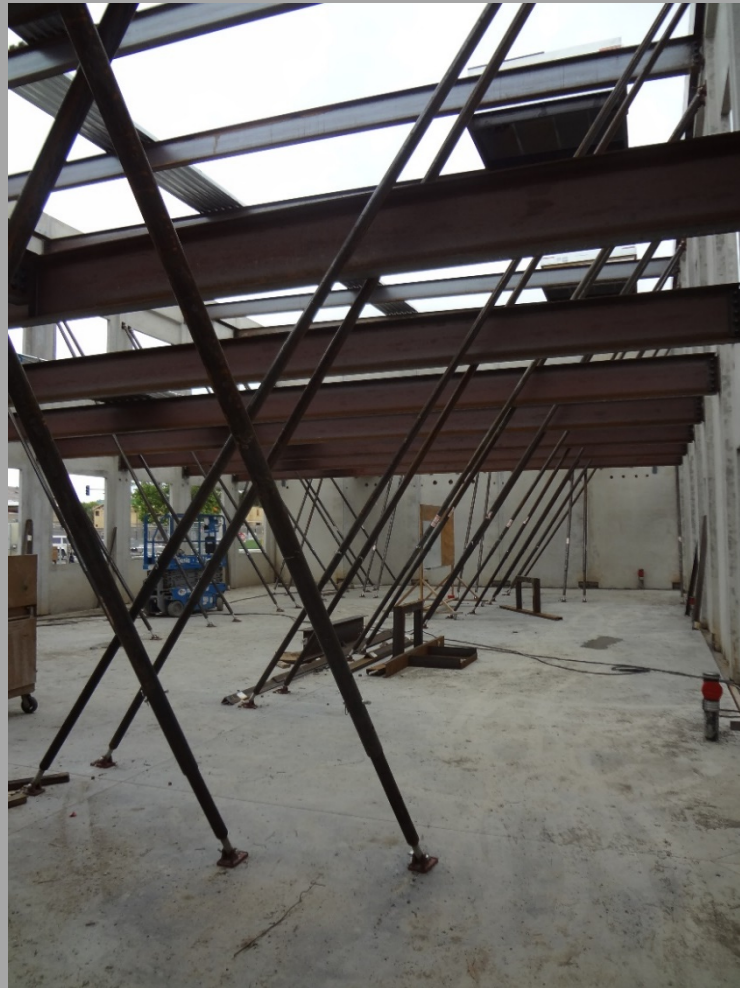
View Of Structural Steel Installation Ongoing In Building N2
