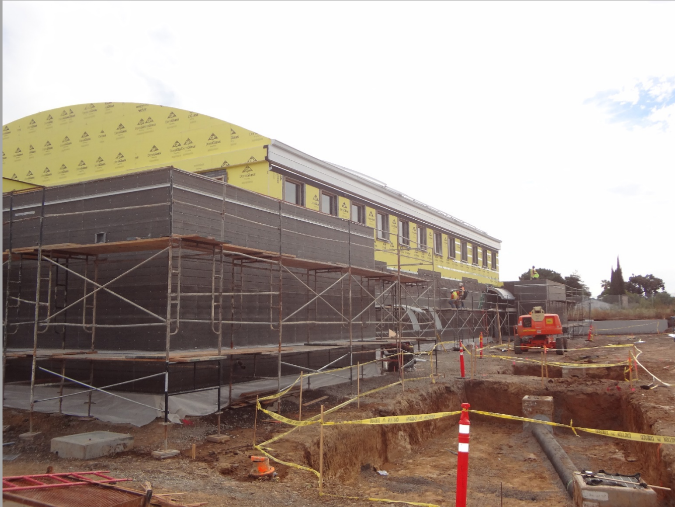
View Of Building Exterior & Bio Retention Swales Looking Northeast
