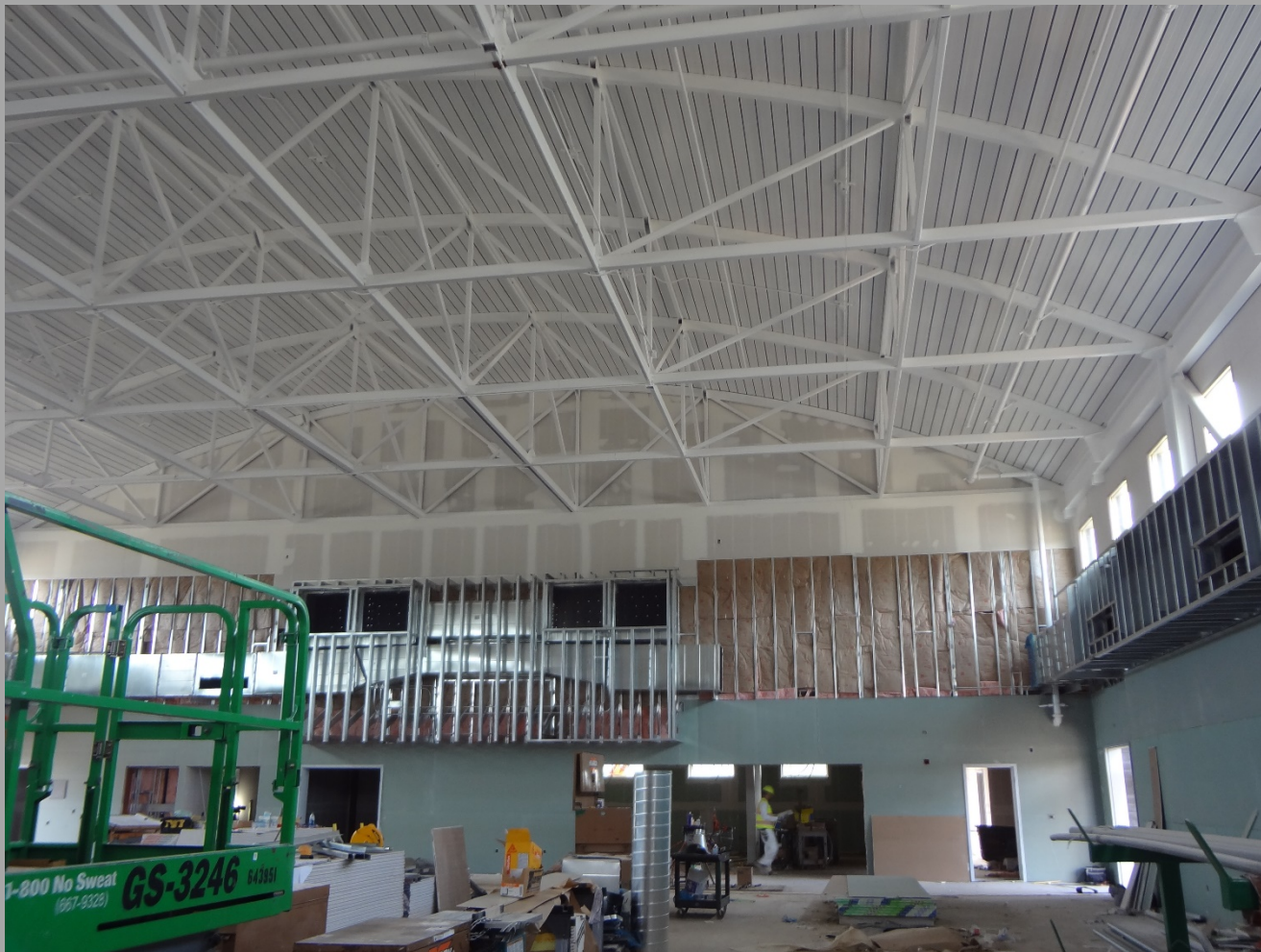
View Of Building Interior Looking East
