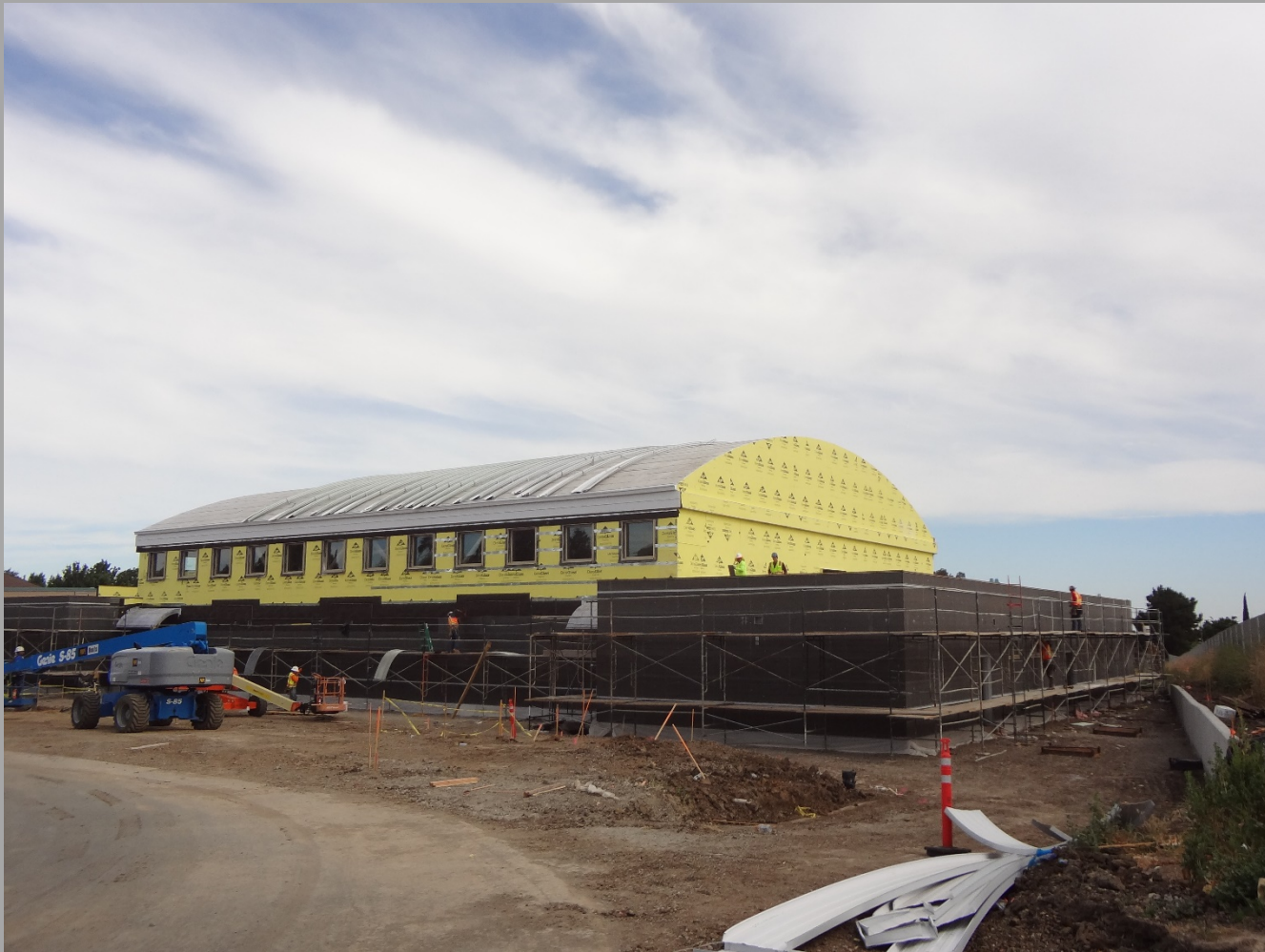
View Of Exterior Looking Northwest
