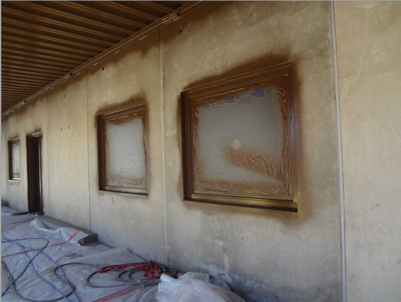
View Of Windows & Door At Covered Walkway Area
