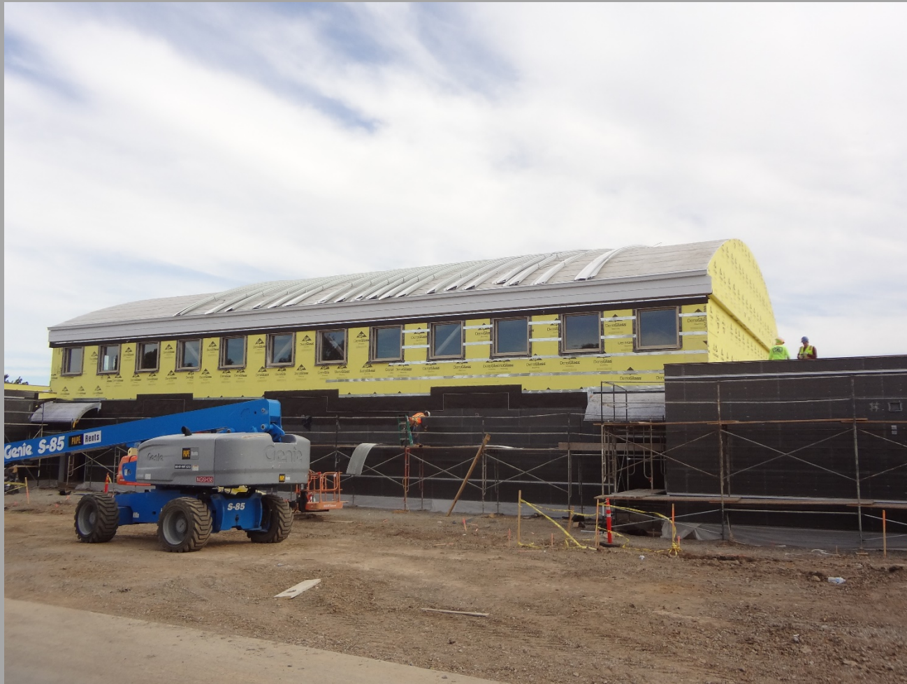
View Of Gym/M.P Exterior and Roof
