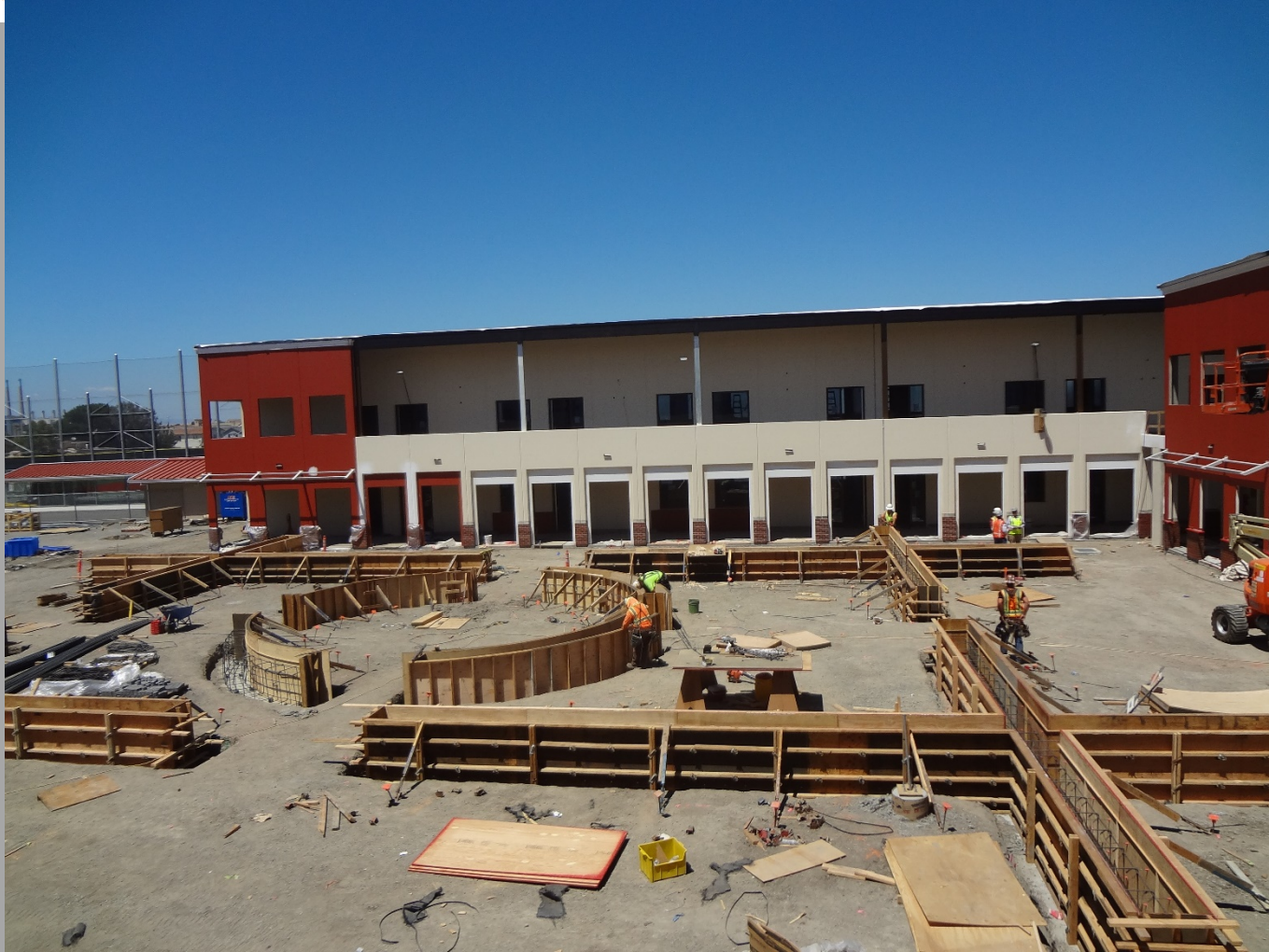
View Of Formwork Ongoing In Courtyard
