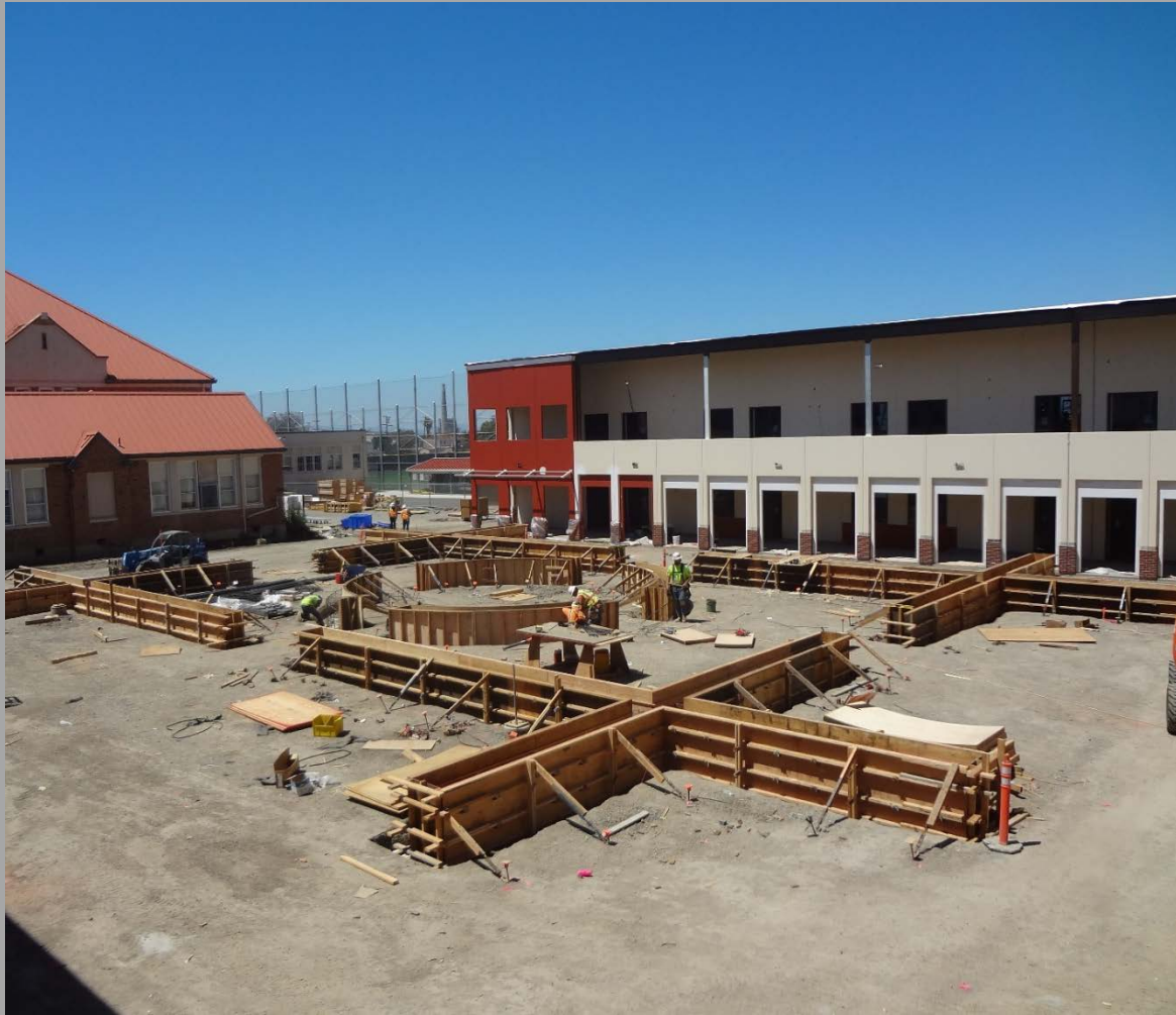
View Of Building N1 & Courtyard
