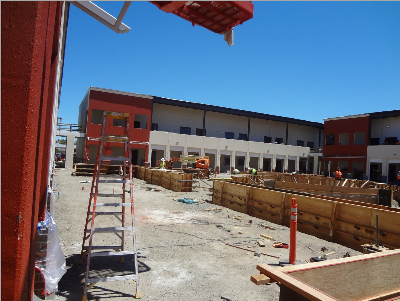
View Of Building N2 & N3 & Formwork Ongoing In Courtyard
