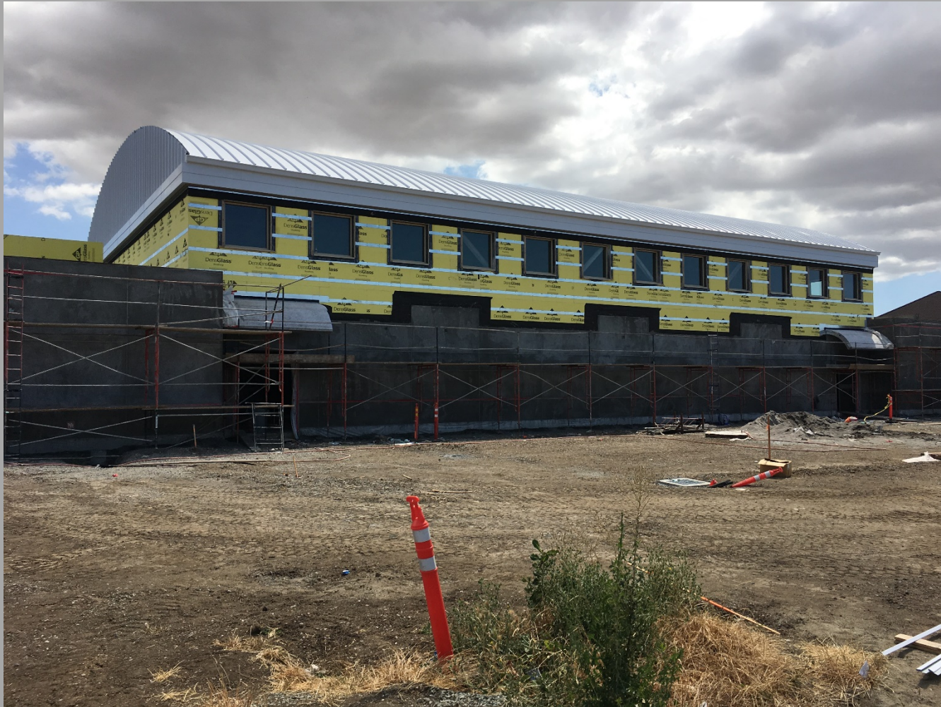
View Of North Face Of The Building Looking Southwest
