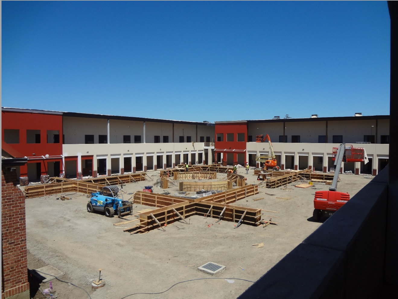
View Of Building N1 & N2 & Courtyard
