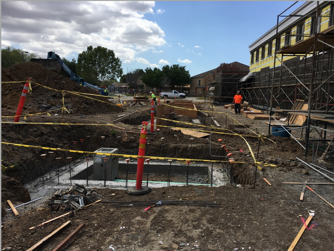
View Of Work On Bio Retention Swales Looking West
