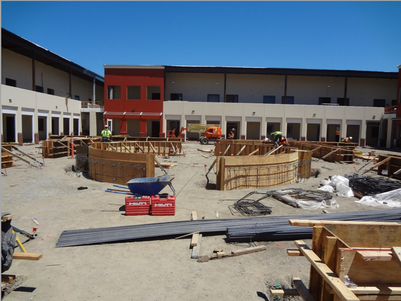
View Of Building N2 & Formwork Ongoing In Courtyard
