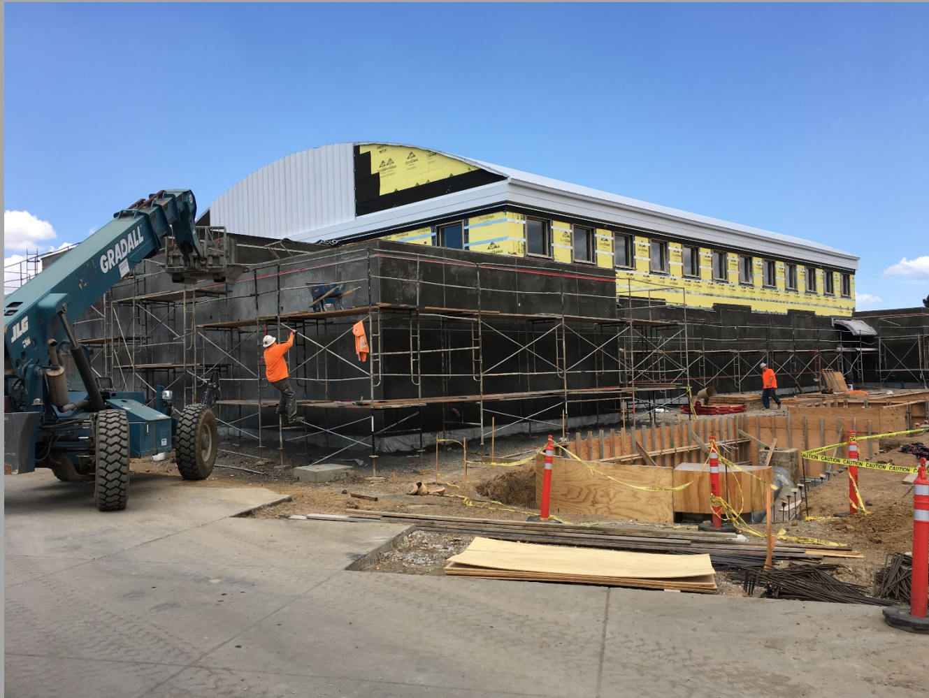
View Of Building Looking Northeast Working On Plaster & Metal Wall Panels
