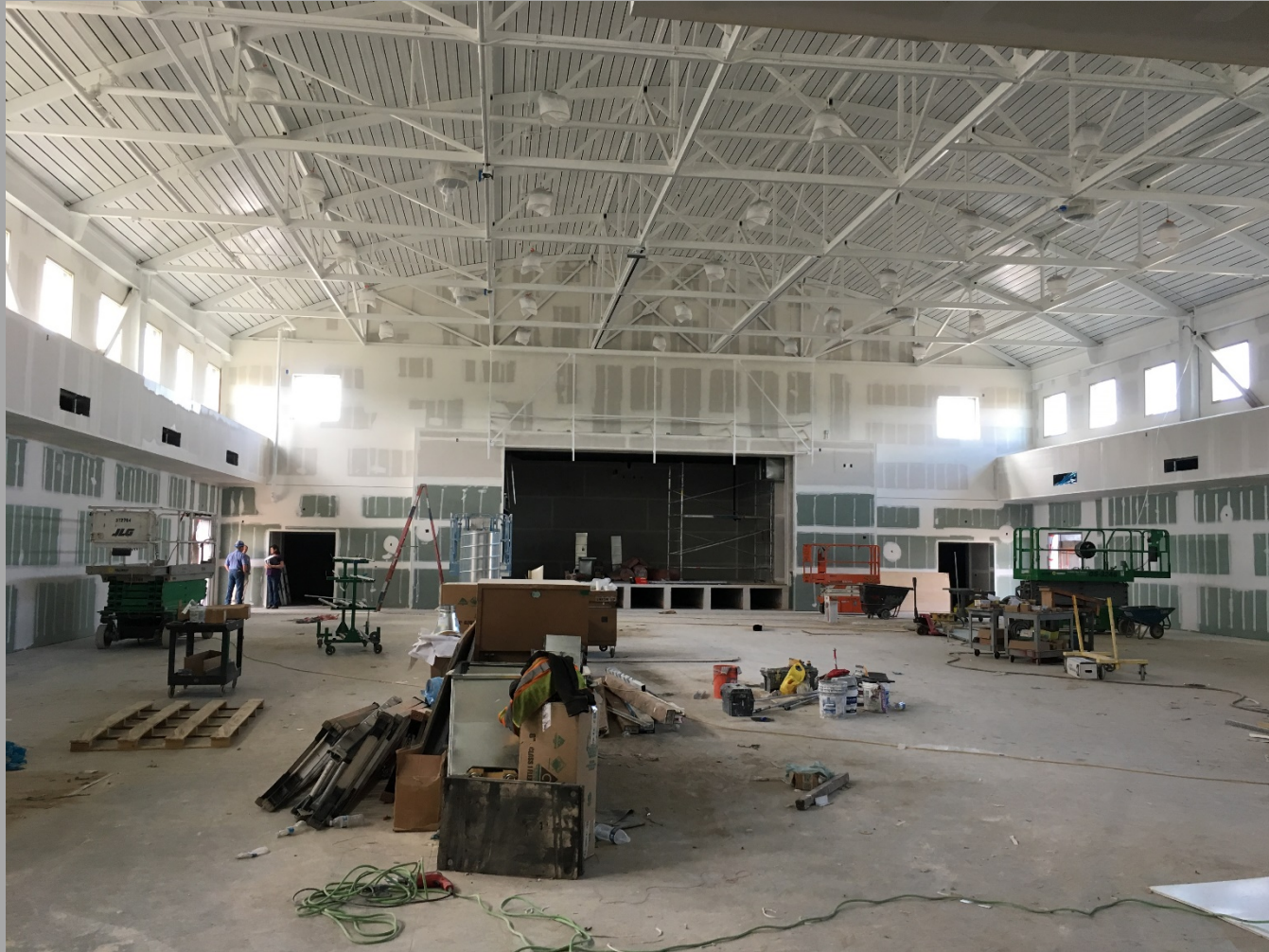
View Of Platform Looking West
