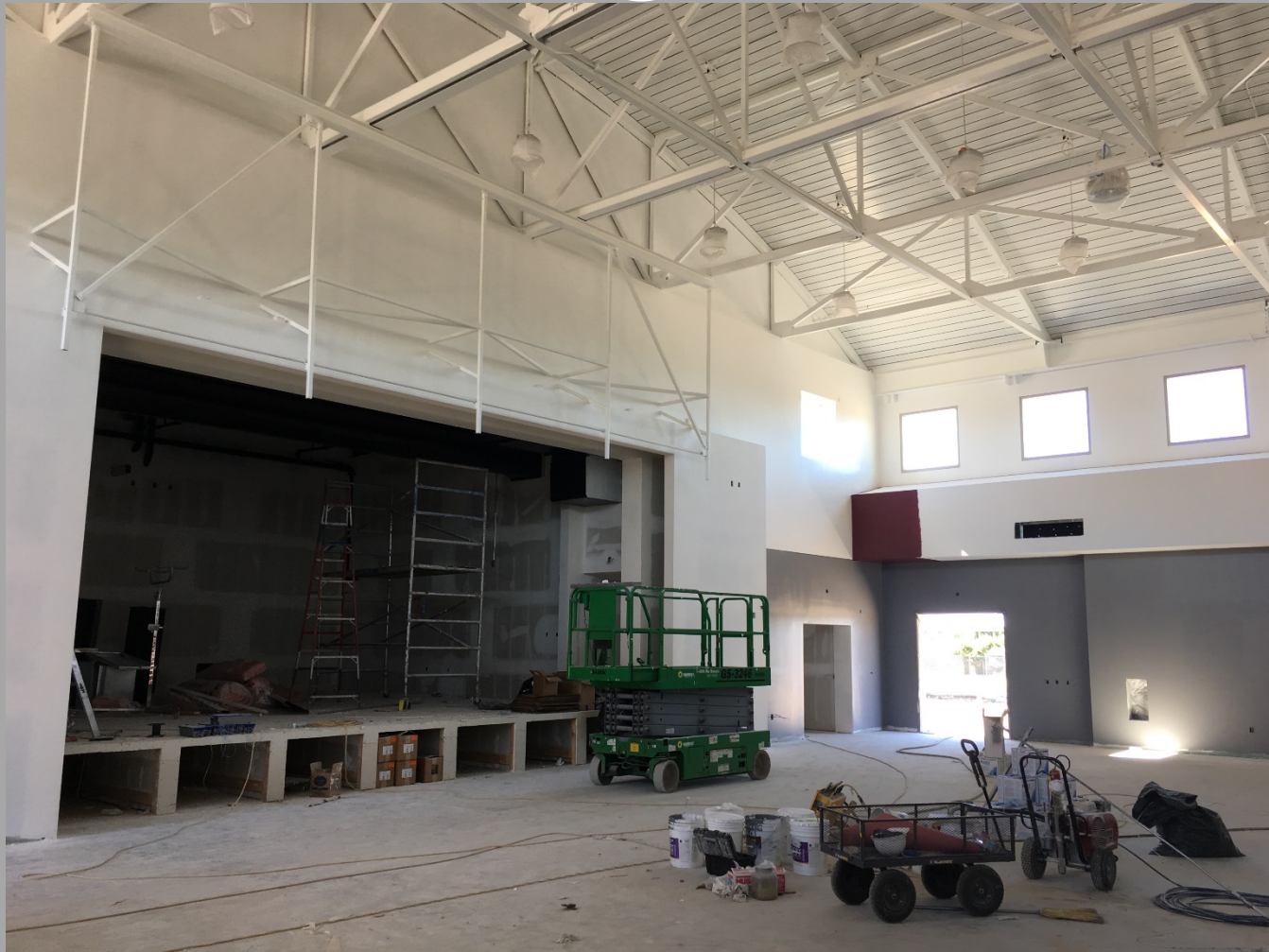
Interior View Of Gym/M.P Space Looking To The Northwest
