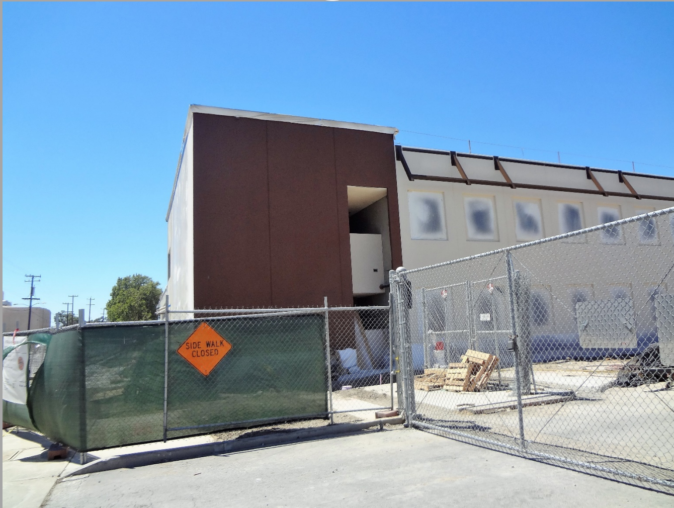
Exterior View Of Southeast Corner Of Building N2
