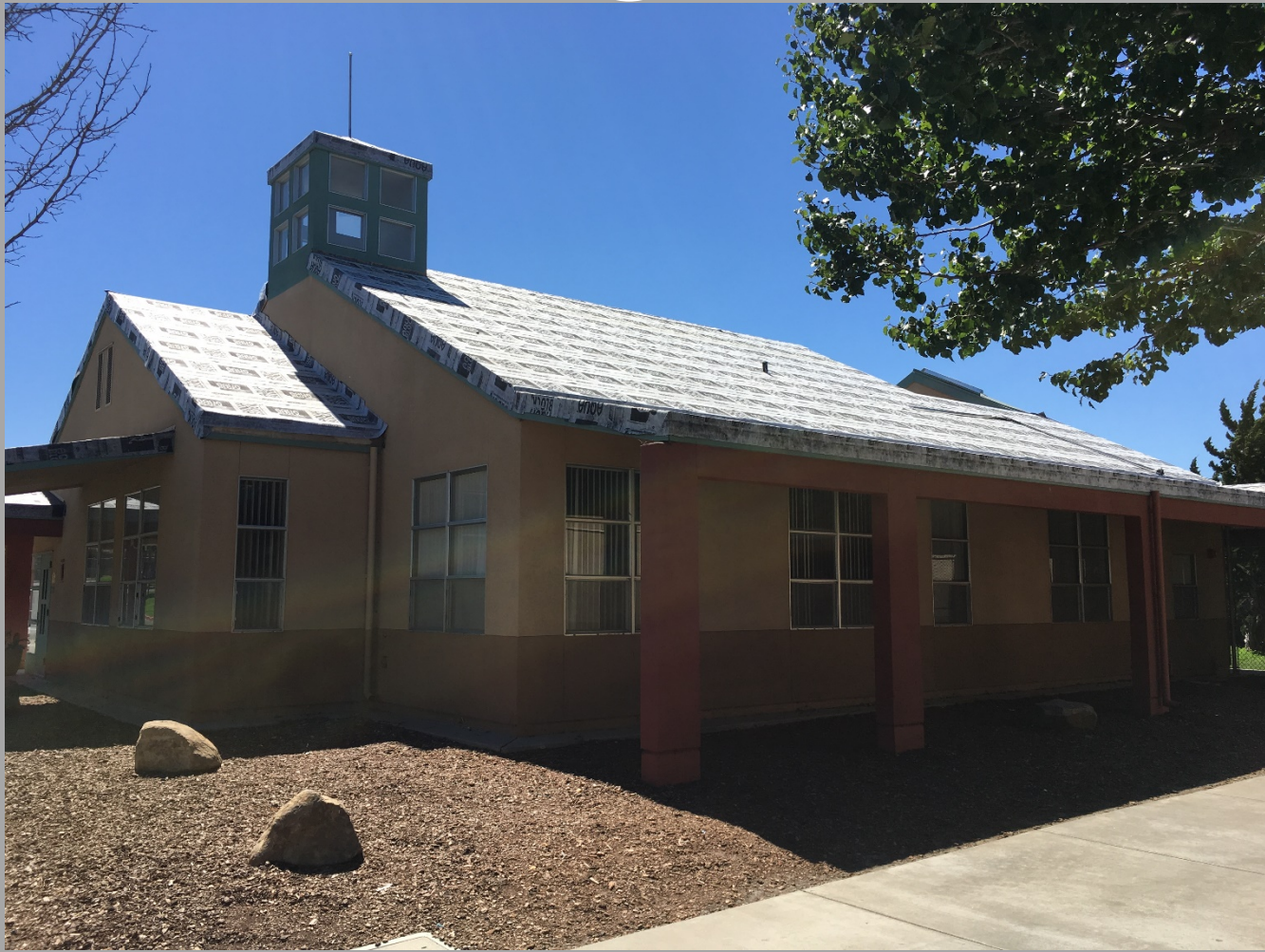
View Of Existing Admin Building Roofing Work
