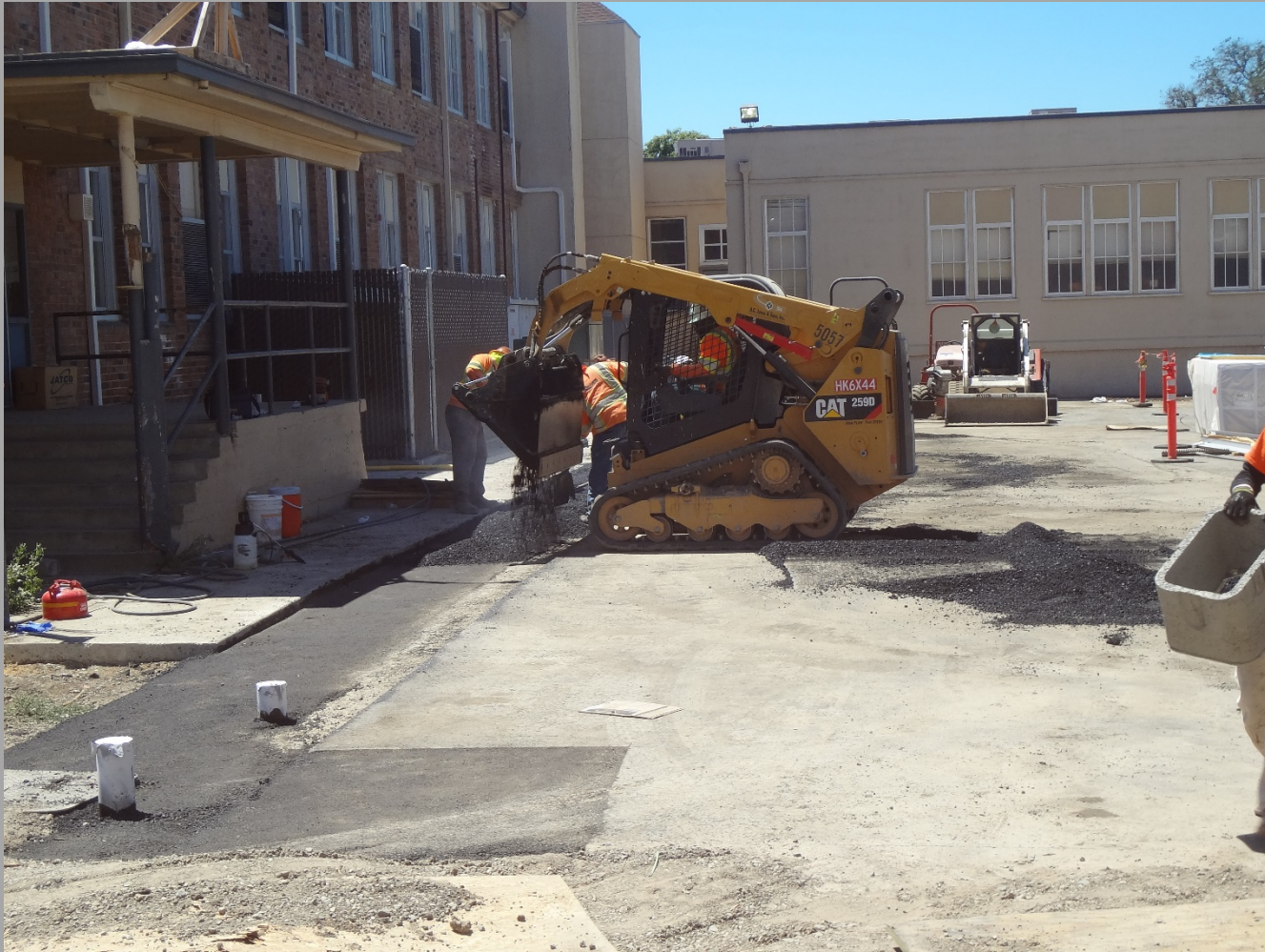
Paving Of New Utility Trenches Behind Existing North Campus Bldg.
