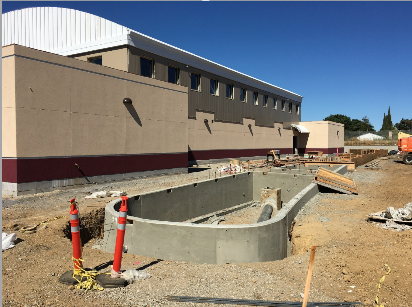
Close Up View Of Bio Retention Swales
