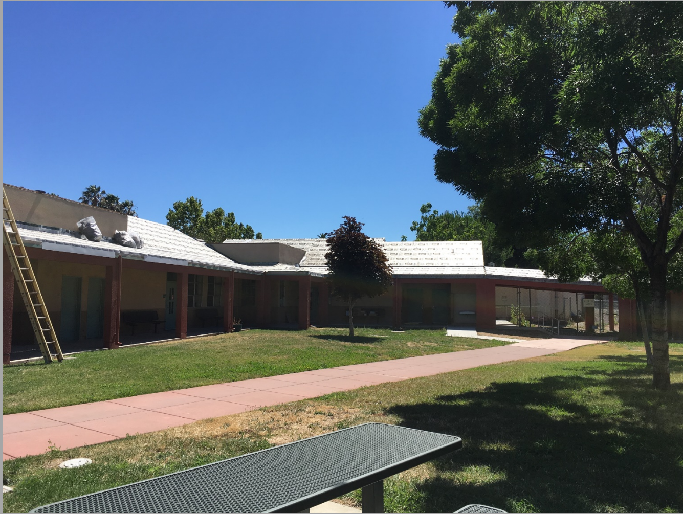
View Of Existing Classrooms Roofing Work
