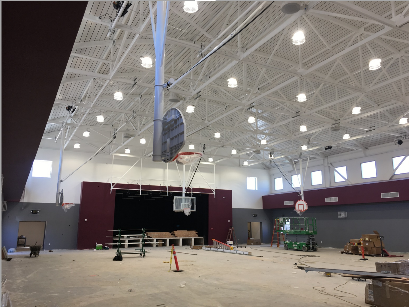
Interior View of New Building Looking Toward Platform
