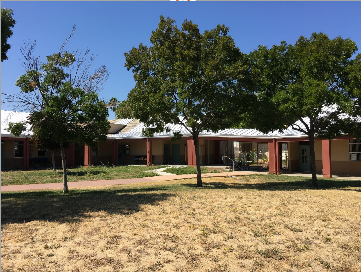
View of New Metal Roofing at Existing School from Interior Courtyard
