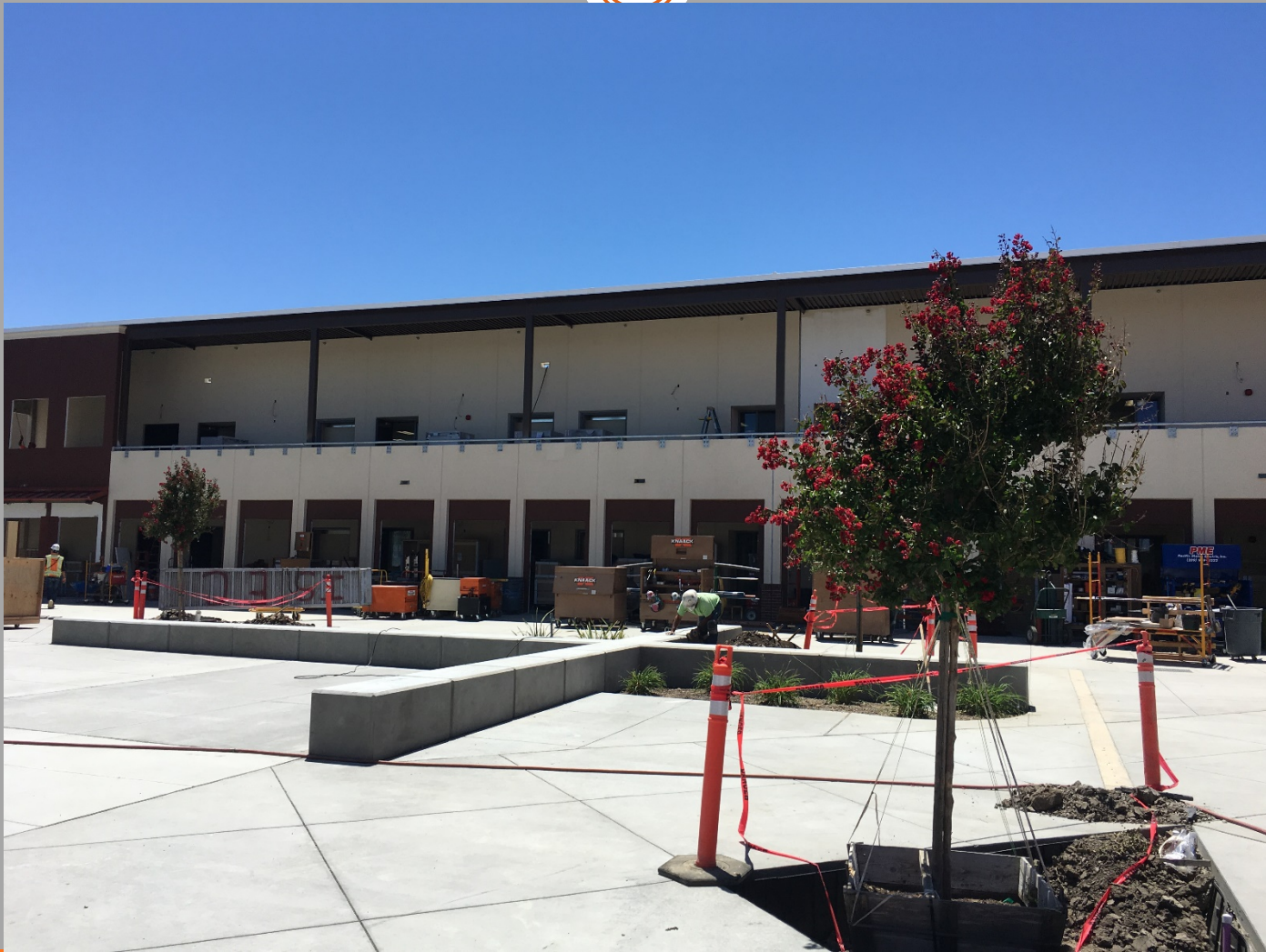
View of North Side of Building N3
