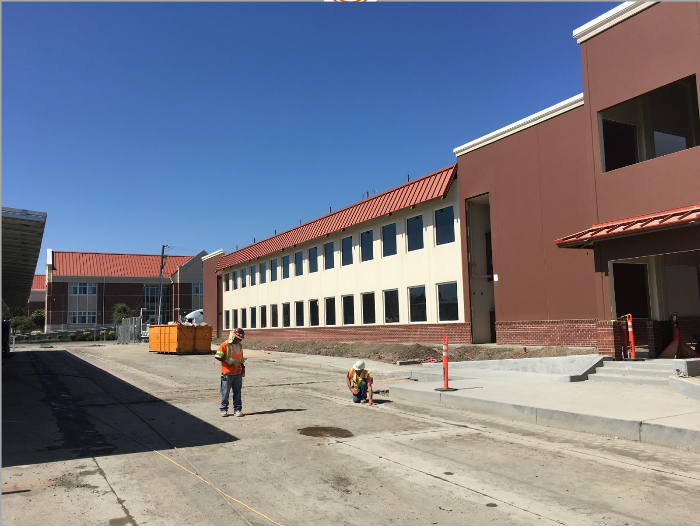
View of East Side of Building N2
