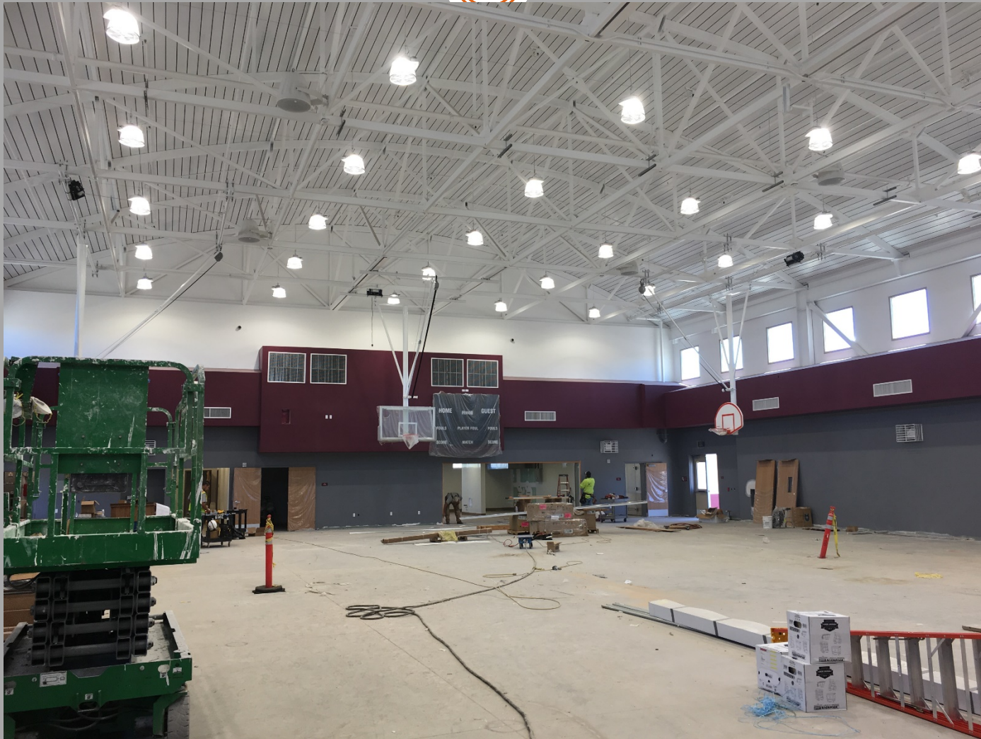
Interior View of New Building Looking Toward Kitchen
