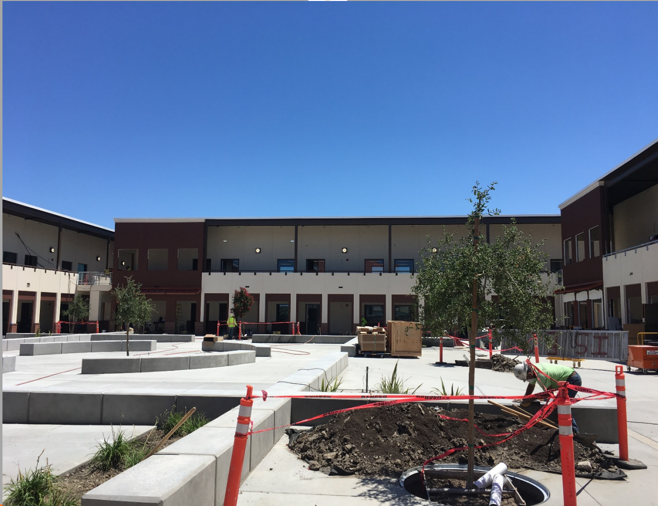
View of West Side of Building N2
