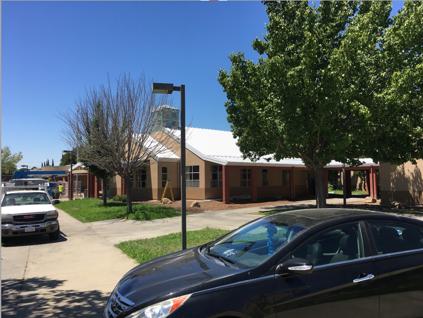
View of New Metal Roofing at Existing School Looking Northwest
