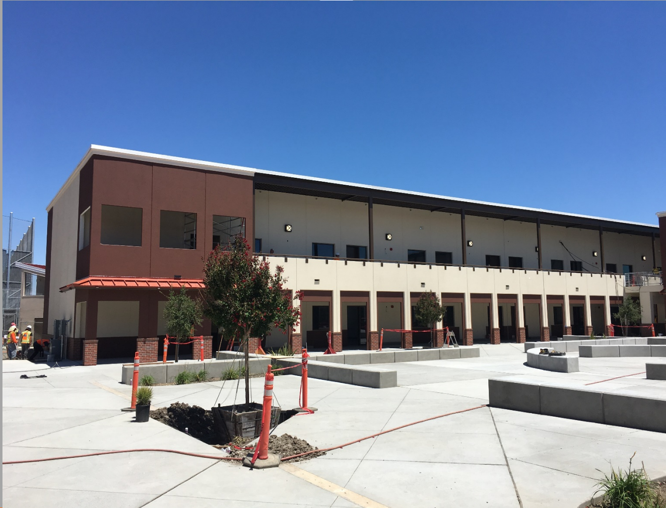
View of South Side of Building N1
