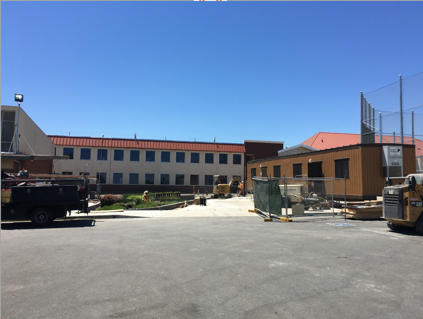
View of North Side of Building N1 & Bio-Retention Swale
