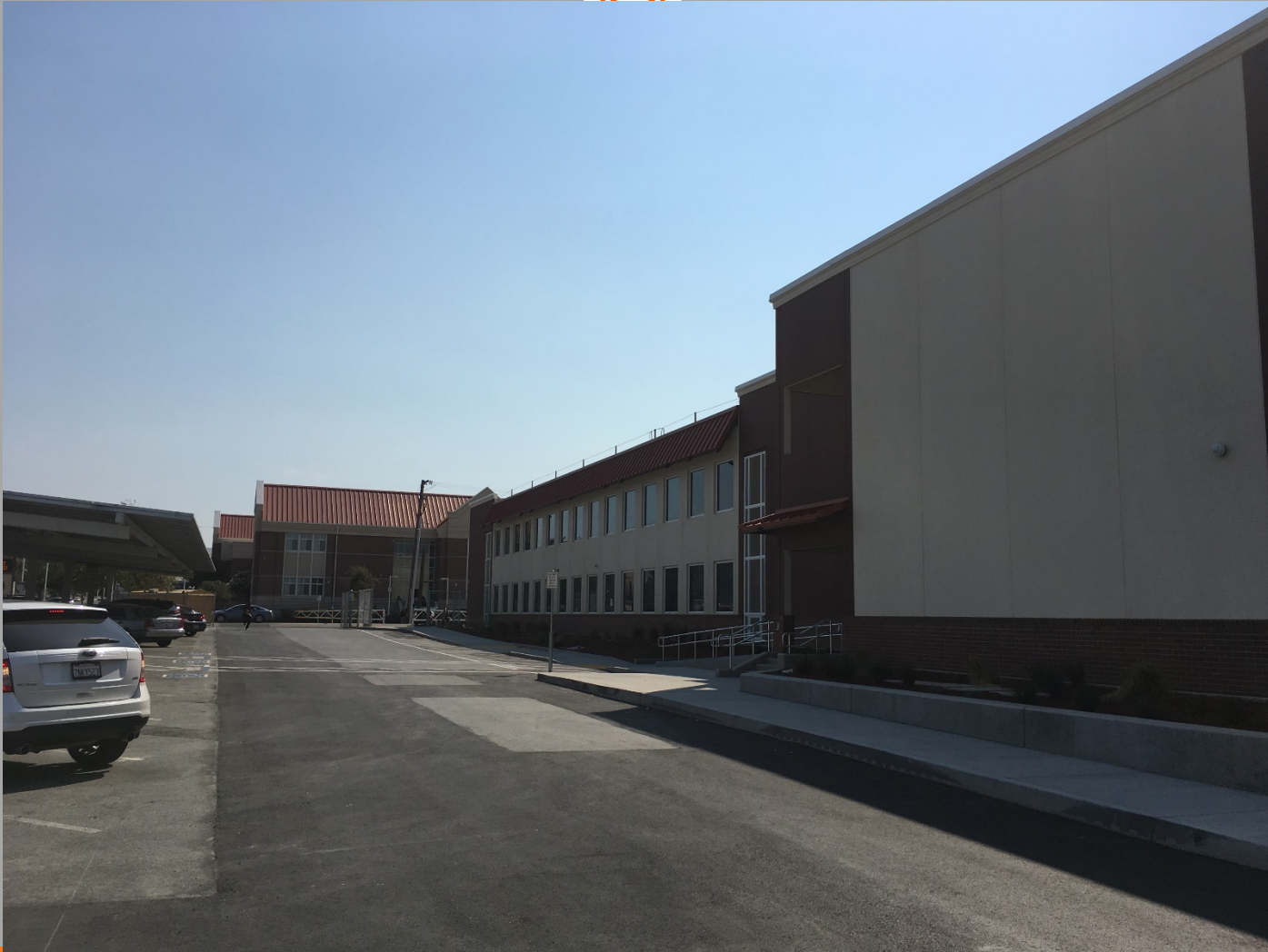
View of Building N1 & N2 from H Parking Lot
