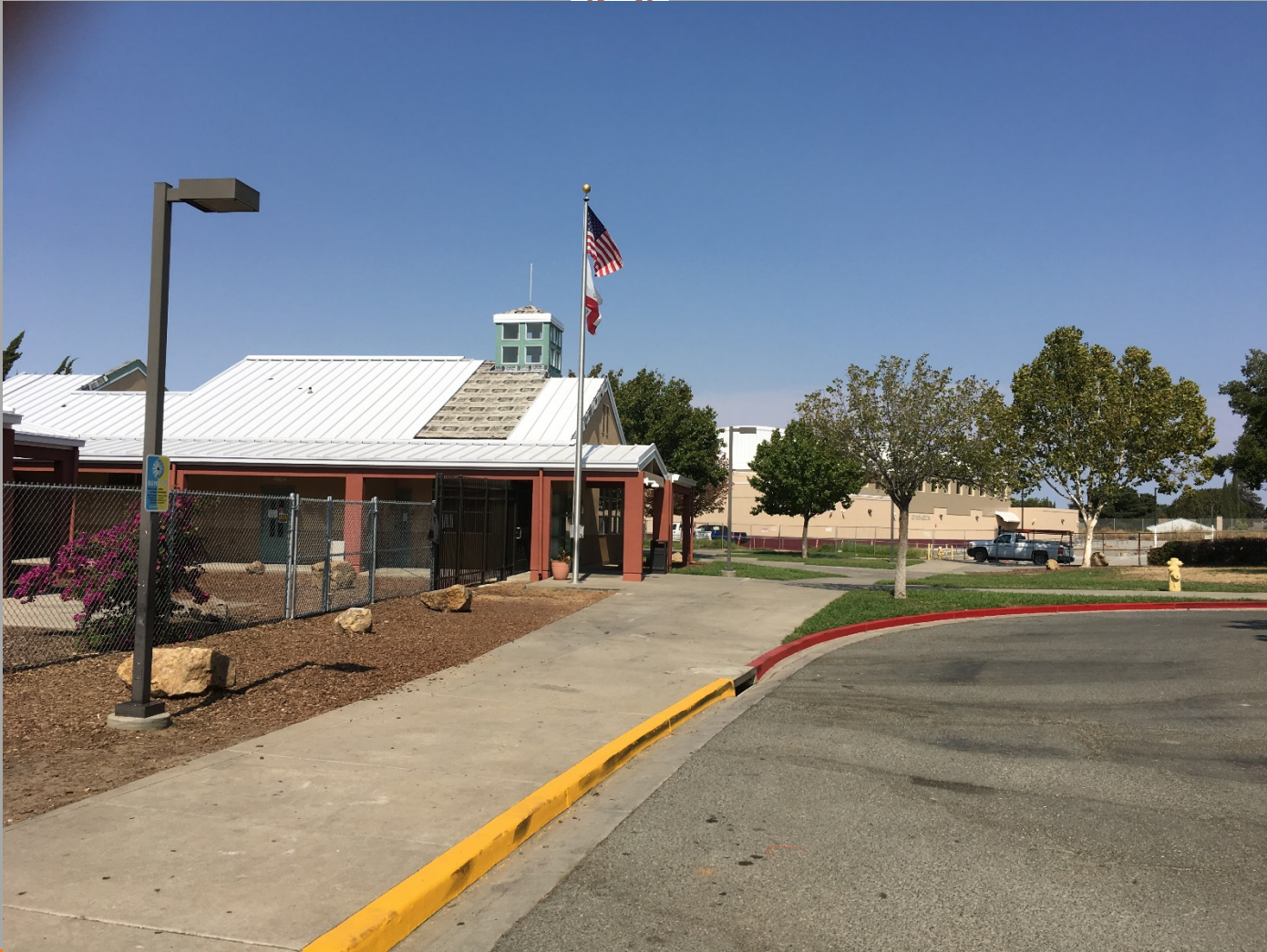
View of New Metal Roofing at Existing School from Front Parking Lot
