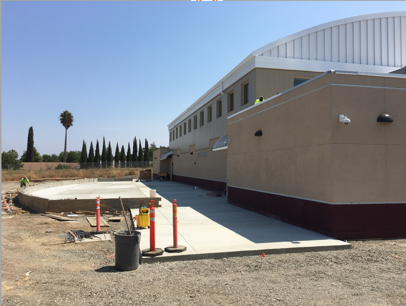
View of New Building Looking Southeast
