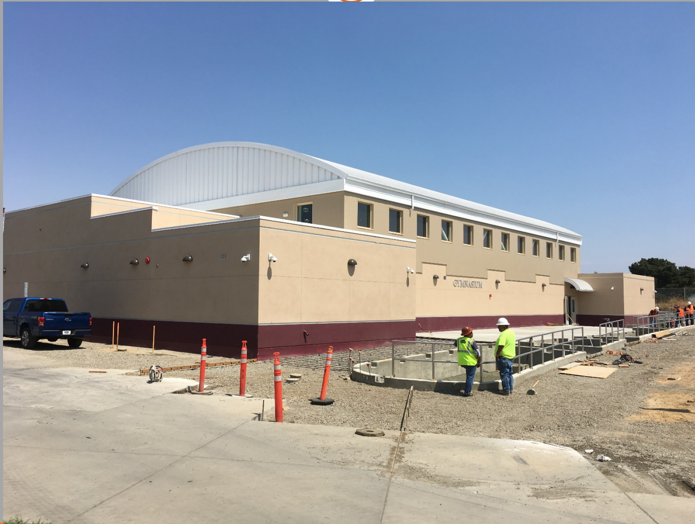
View of New Building Looking Northeast
