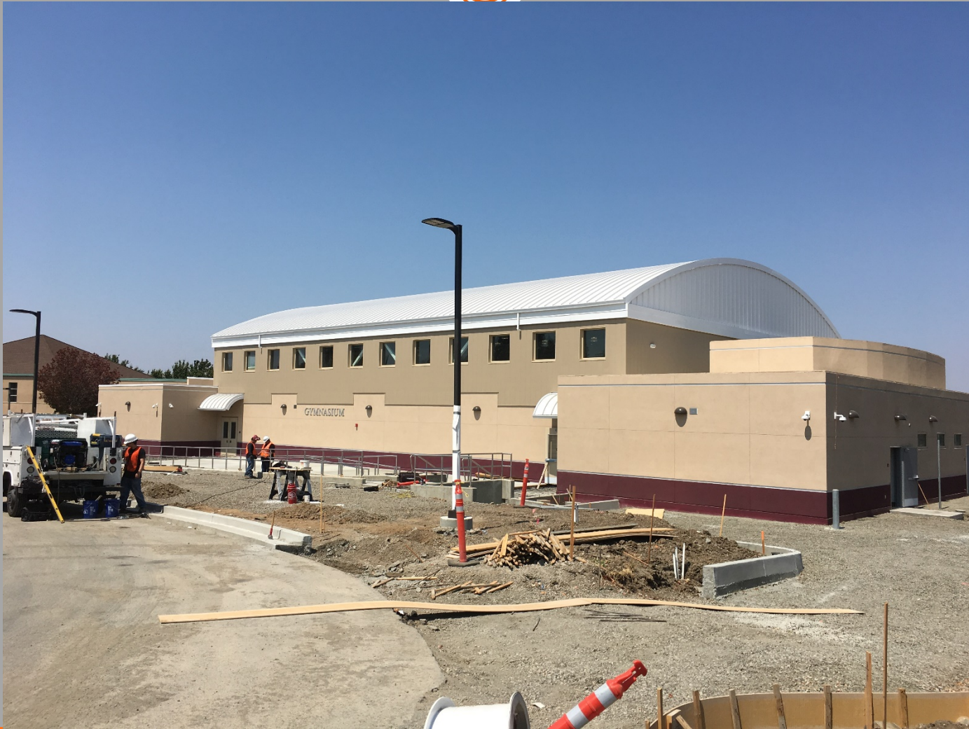
View of New Building Looking Northwest
