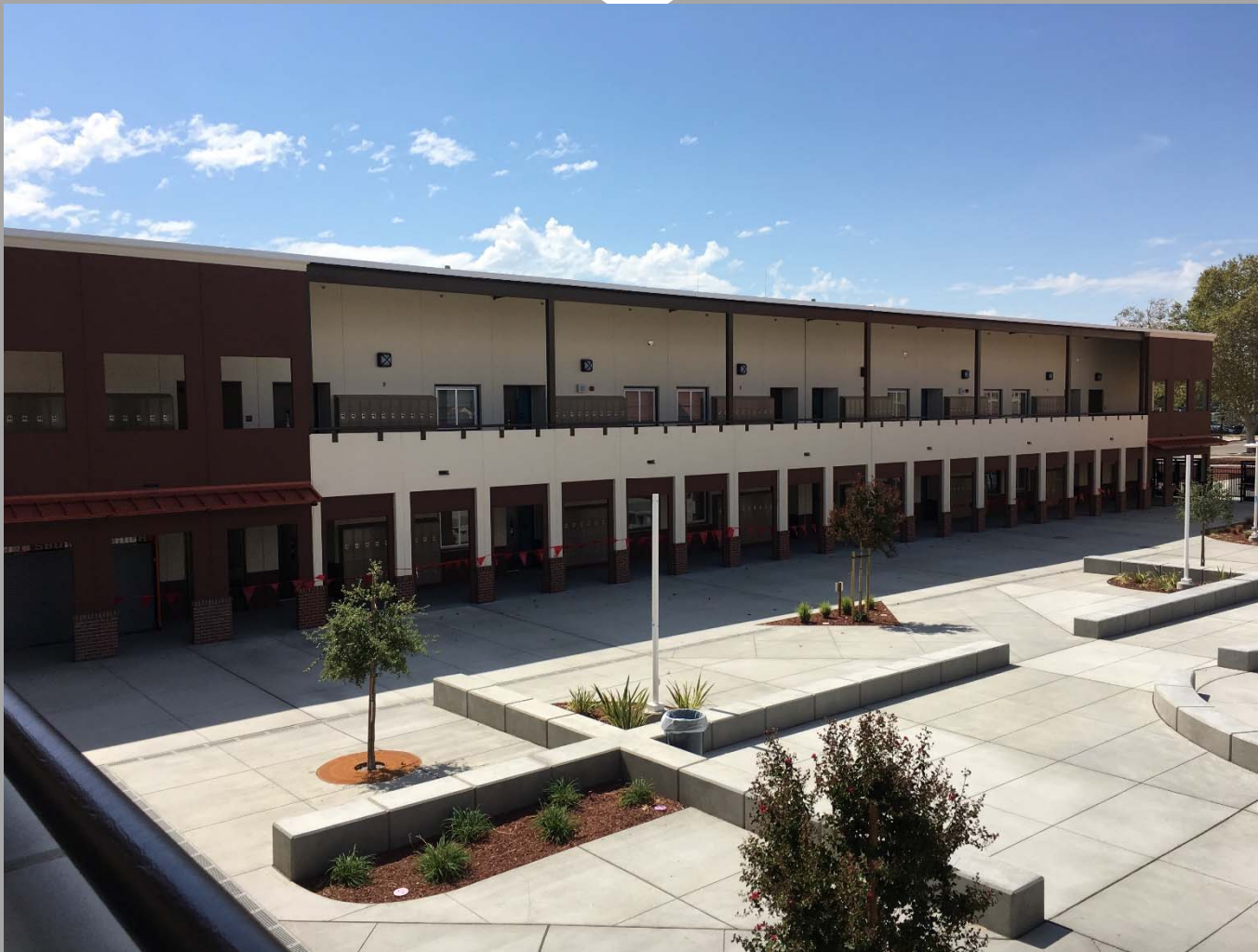
View of Building N3 (Science Labs)
