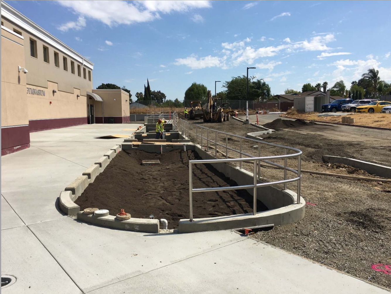
View of Grading Work at Parking Lot Side of New Building
