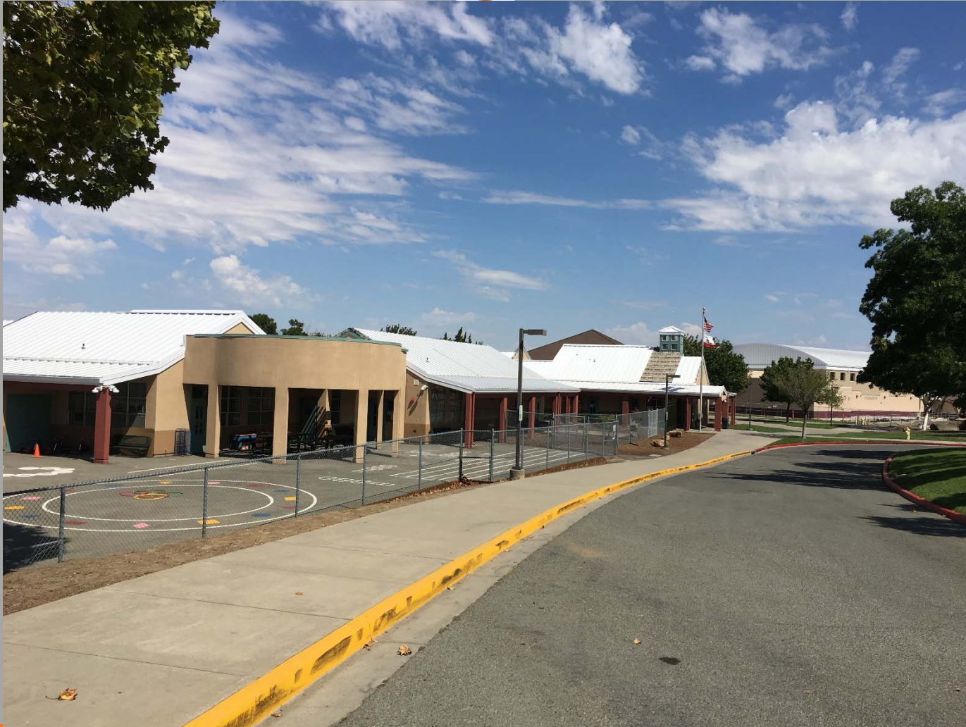
View of New Roofing at Existing Buildings
