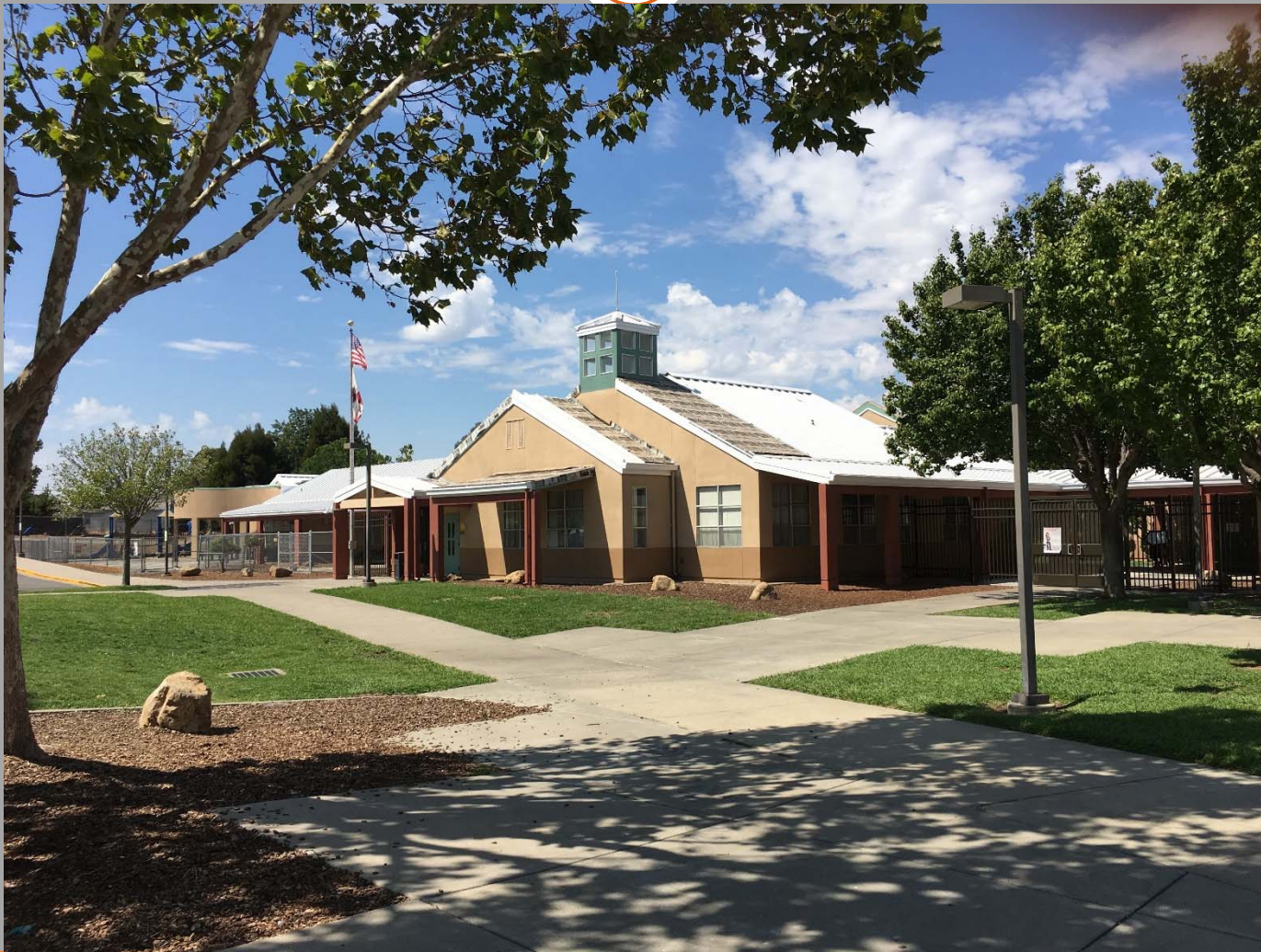
View of New Roofing at Existing Buildings
