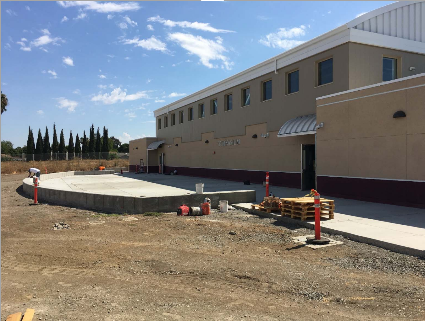
View of New Building Looking Southeast
