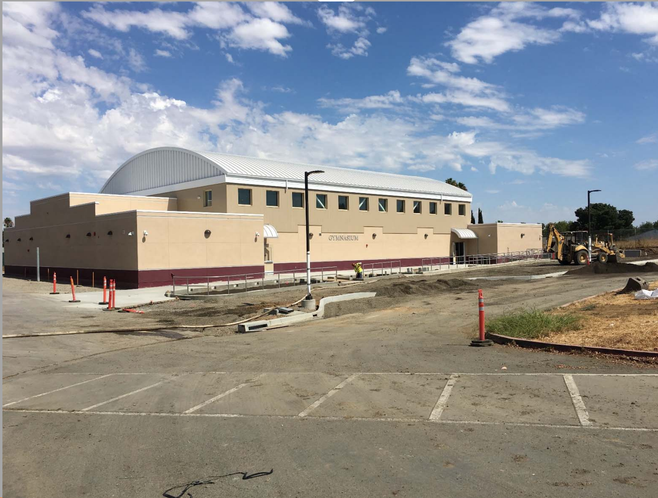
View of New Building Looking Northeast
