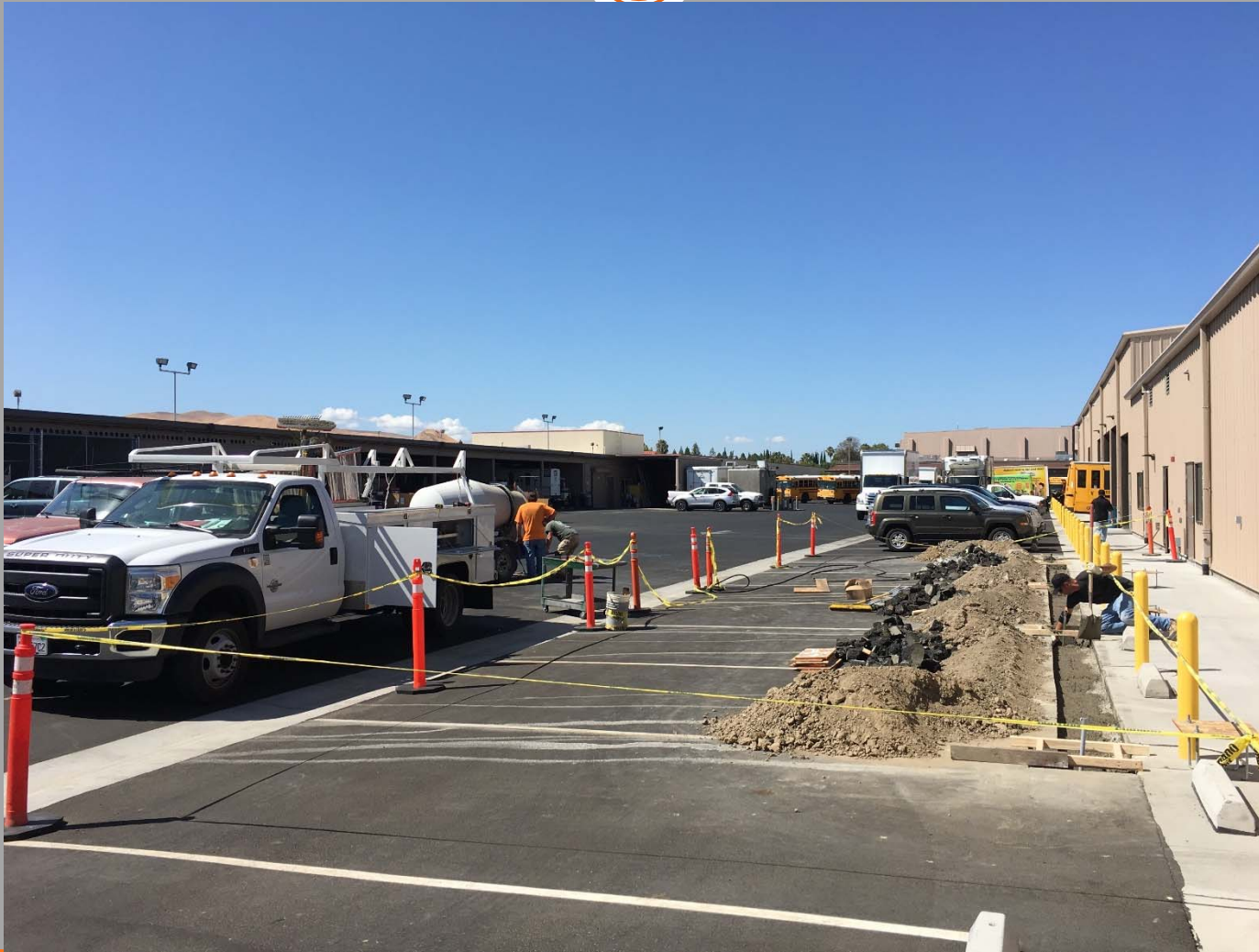
View of Concrete Pour at Charging Station Pedestals
