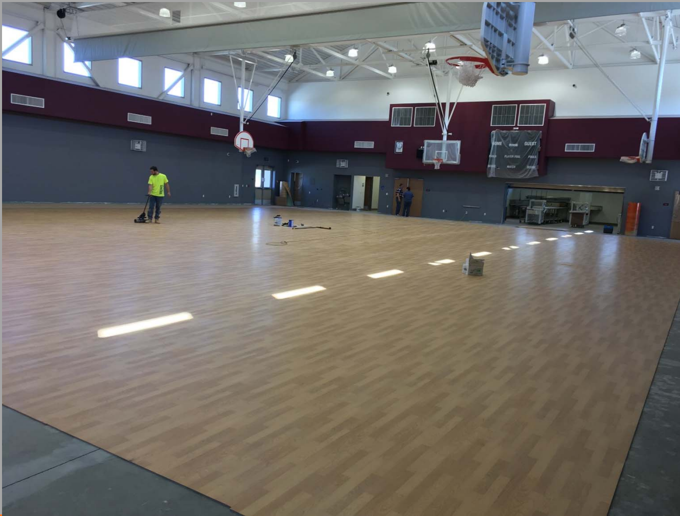
View of Flooring Installation in Gym./MP Space
