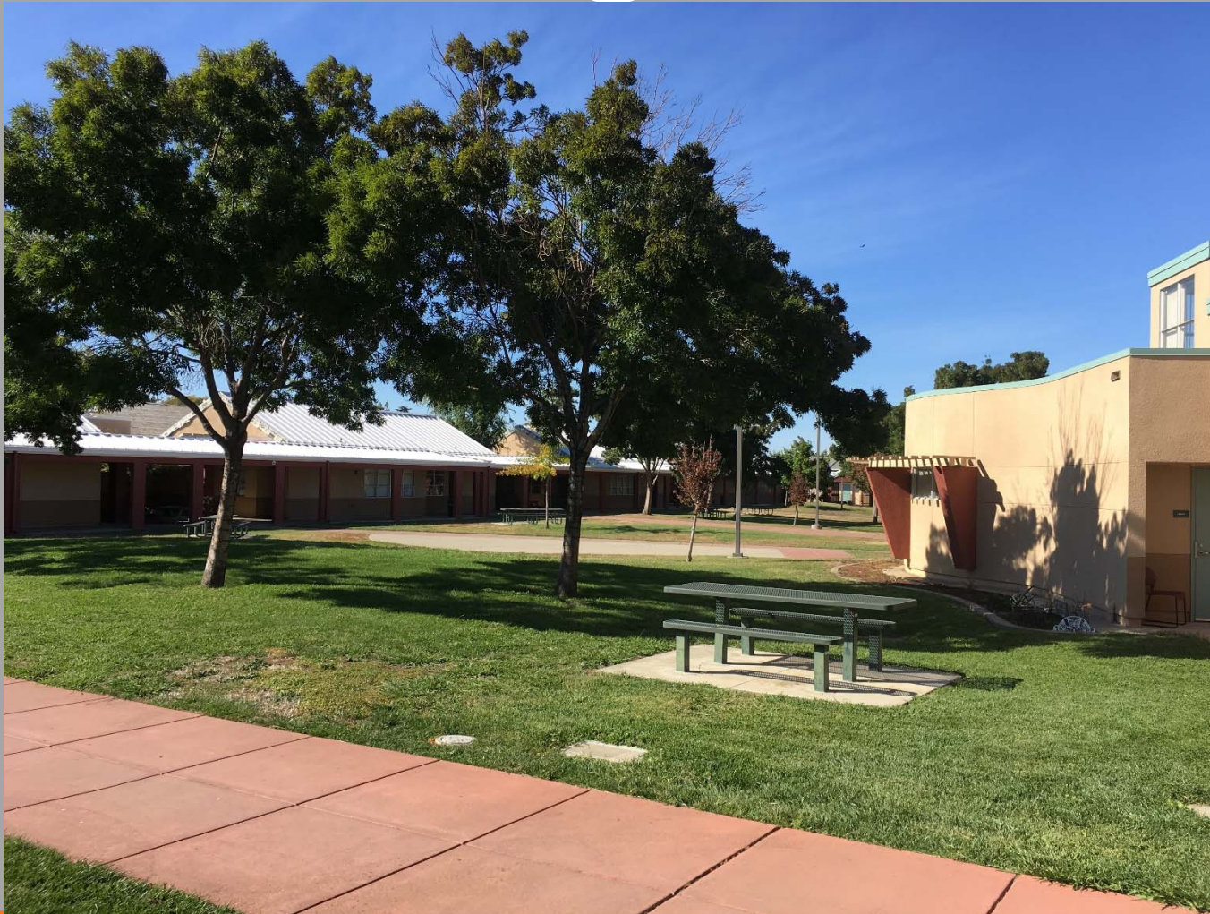
Courtyard Side View of New Roofing at Classrooms
