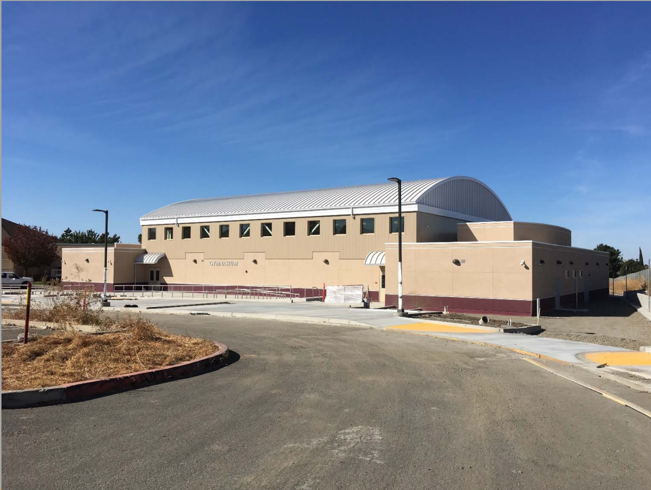
View of New Building Looking Northwest
