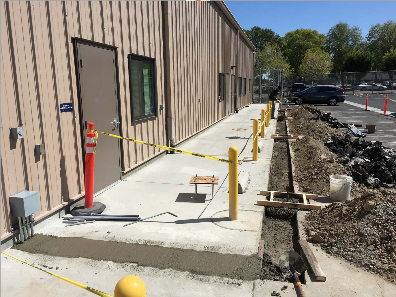
View of Concrete Repair and Forms for Charging Station Pedestals
