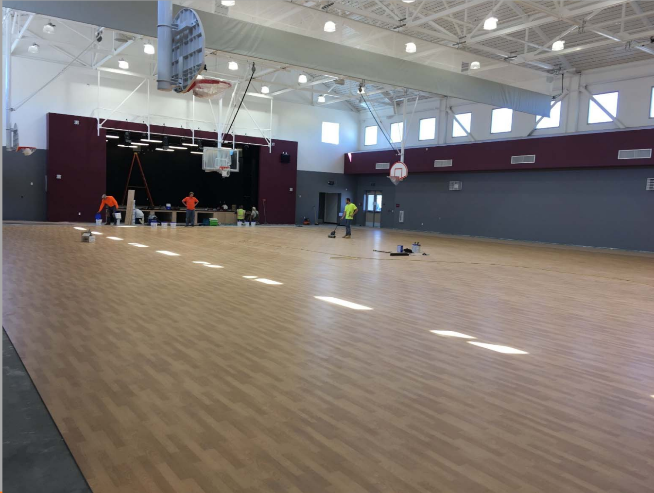
View of Flooring Installation in Gym./MP Space
