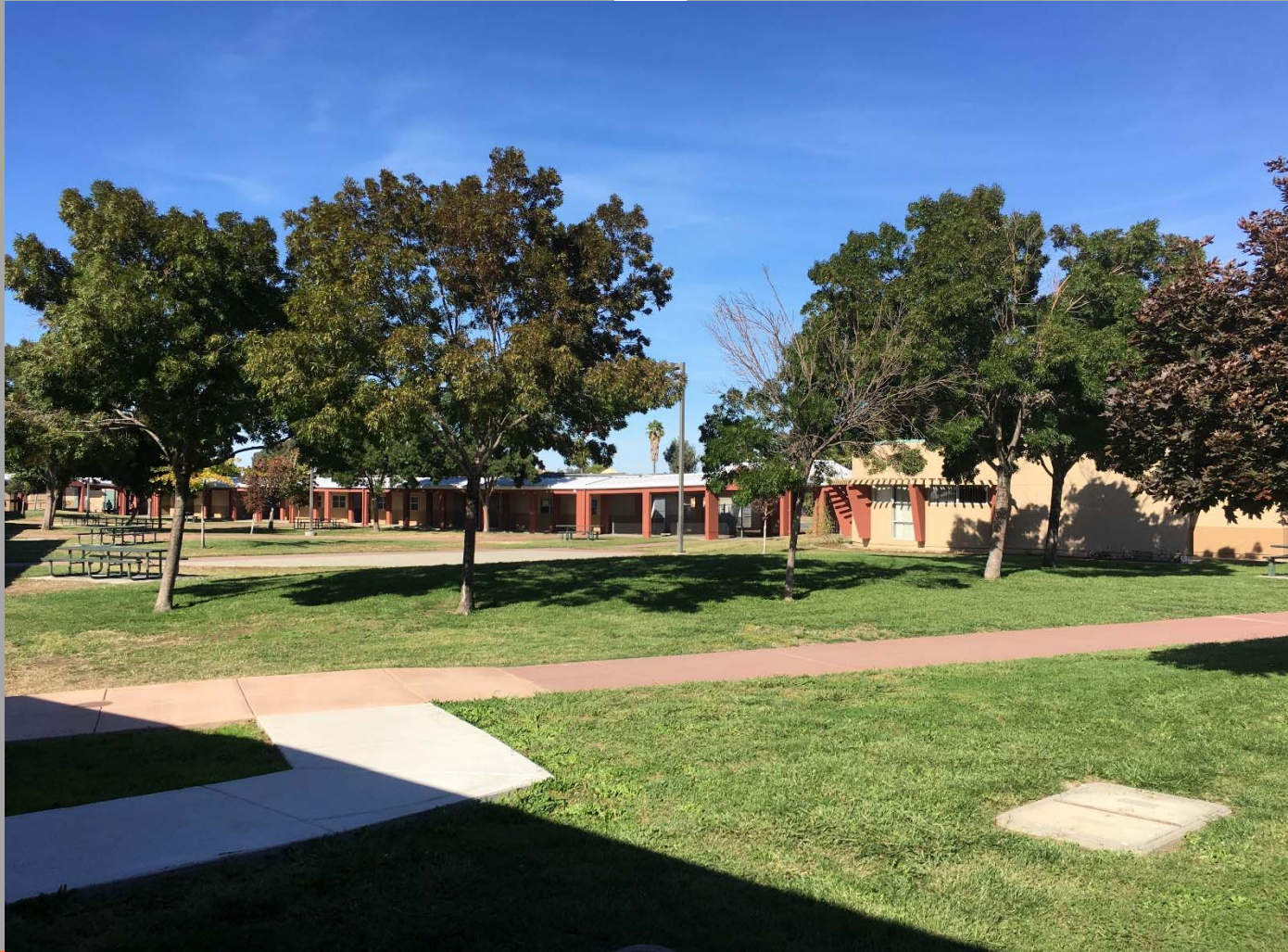
Courtyard Side View of New Roofing at Covered Walkway
