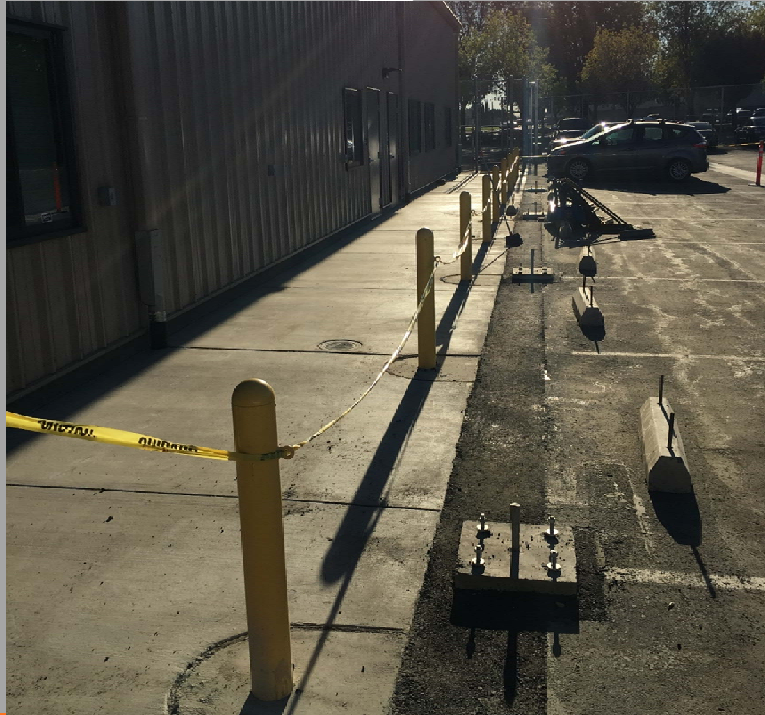
View of Completed Charging Station Pedestals and Paving Repair
