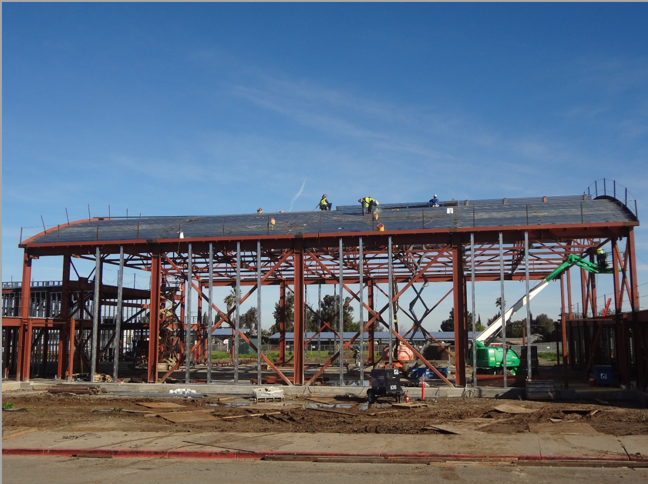
New Gym./MP Bldg. Roof Decking & Exterior Walls Framing Ongoing - Looking North
