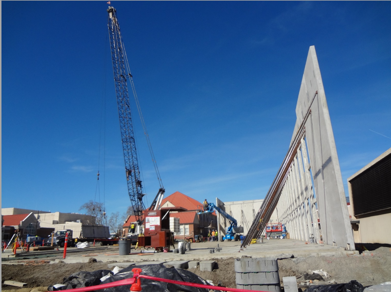
New 12 Classrooms Building (Bldg. N1) North Exterior Wall Panels Installation
