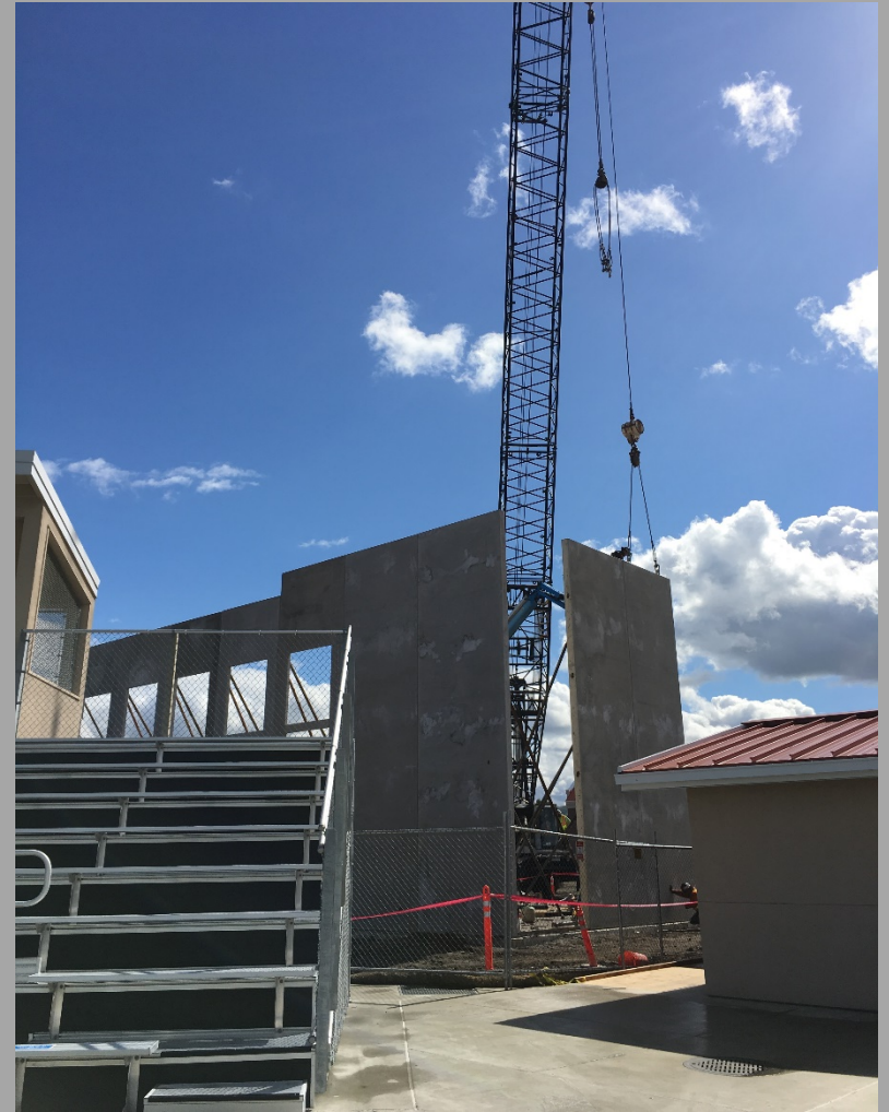
New 12 Classrooms Bldg. (Bldg. N1) Exterior Walls; Panels Installation Begins
