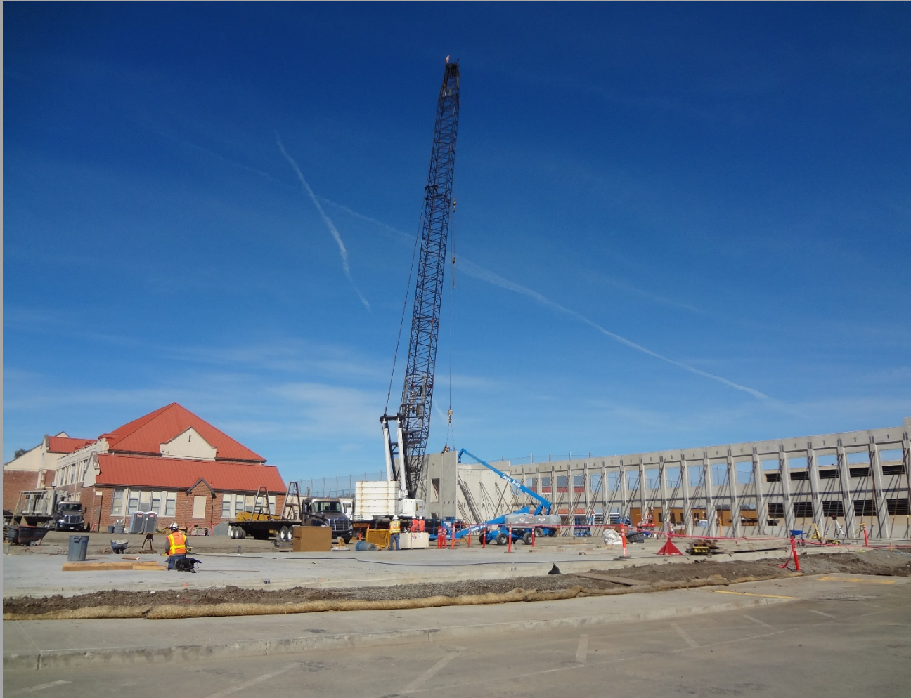
New 12 Classrooms Bldg. (Bldg. N1) Overall View Of Exterior Wall Panels In Place
