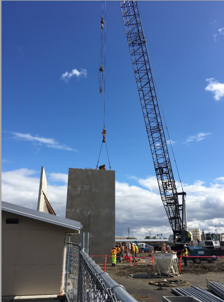
New 12 Classrooms Bldg. (Bldg. N1) Exterior Walls; Panels Installation Begins
