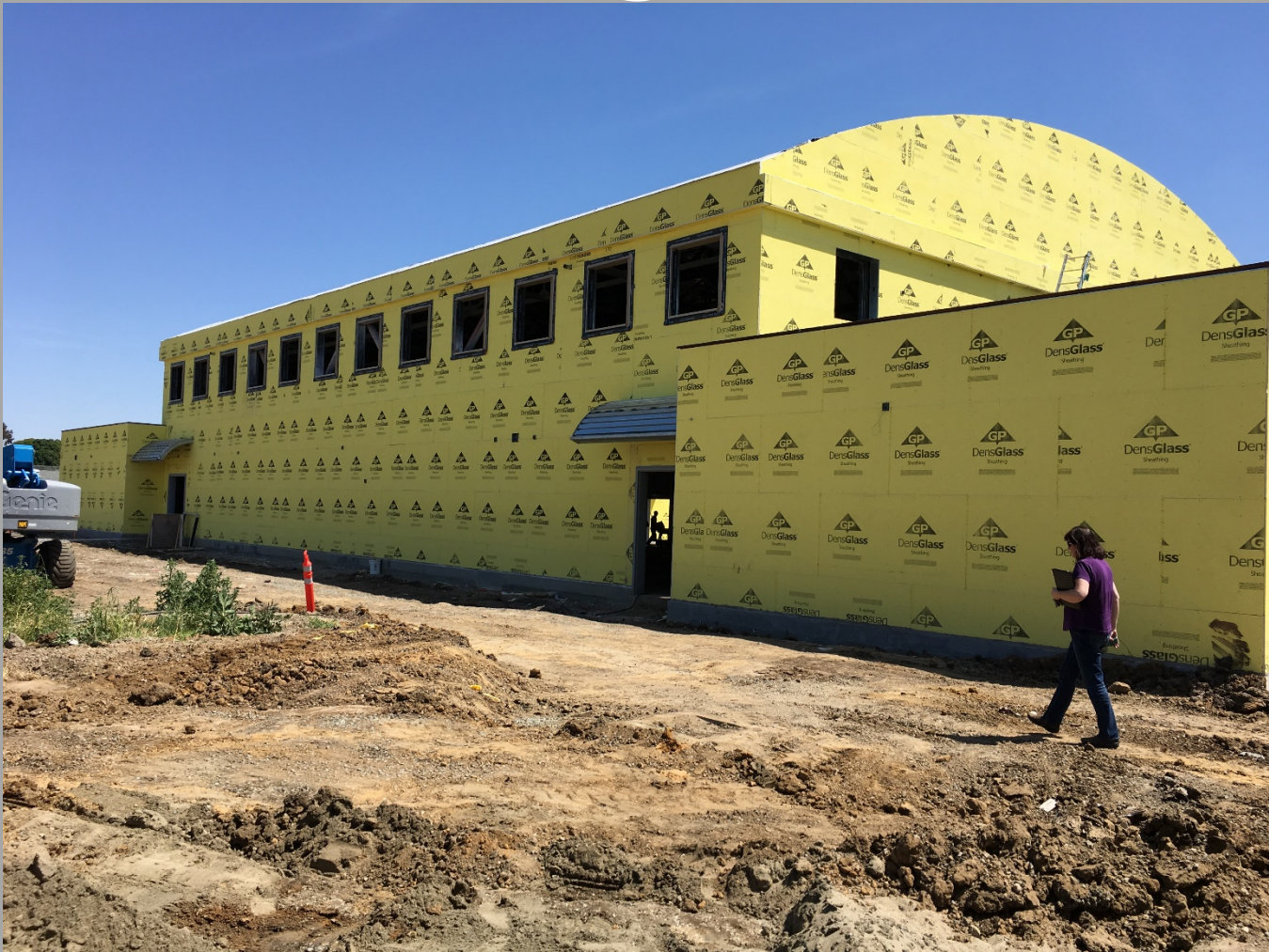
View Of Exterior Looking Southeast
