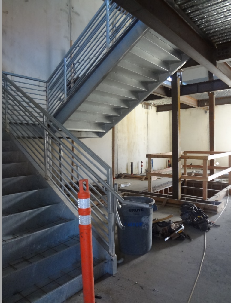
View Of Stairwell and Elevator At East End Of Building N3
