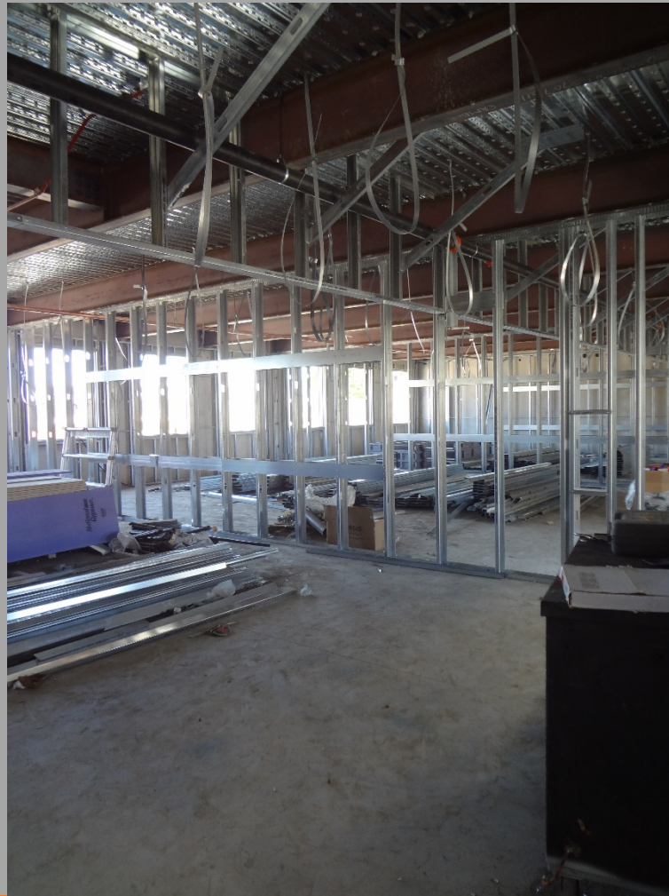
Classroom Wall Framing & Utility Rough-Ins In Progress At N2
