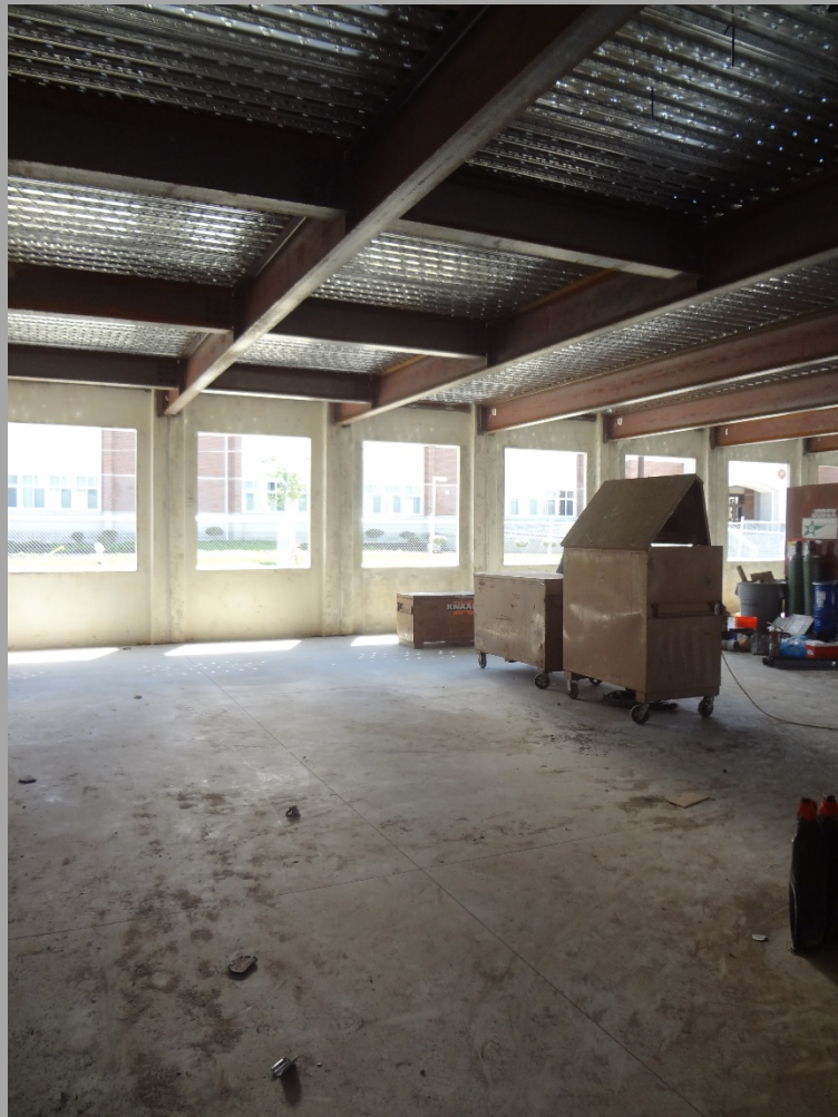
Interior View Of Typical Science Lab
